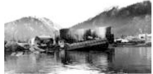
Damage to port facilities in Seward, Alaska, from the 1964 tsunami. Locating industrial facilities outside of inundation zones is the most effective mitigation technique. Credit: U.S. Army Corps of Engineers
