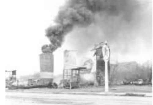
Petroleum tank on fire due to damage from the 1964 tsunami on Highway 101 near Crescent City, California. Credit: Del Norte Historical Society
