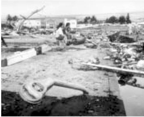
Damage from the 1960 tsunami in the Waiakea area of Hilo, Hawaii. Parking meters were bent by the force of the debris-filled waves. Credit: U.S. Navy
