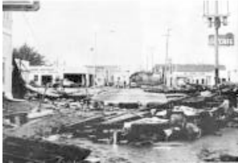
Damage to Crescent City, California, from the 1964 tsunami. Nearly 900,000 people in the five Pacific states live in the inundation zone for a 50-foot tsunami. Credit: Del Norte Historical Society
