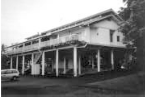
Elevated restaurant in Hilo, Hawaii. Lower level is designed to allow waves to pass through. Credit: Mintier & Associates
