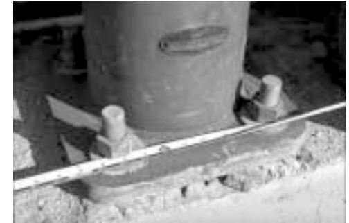
Anchor bolts. Measures to resist earthquake shaking, such as anchoring and bracing buildings, can also help to reduce tsunami damages. Credit: Northridge Collection, Earthquake Engineering Research Center, University of California, Berkeley
