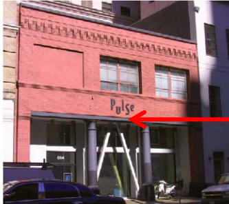
Steel braced frame inserted in a small commercial structure
