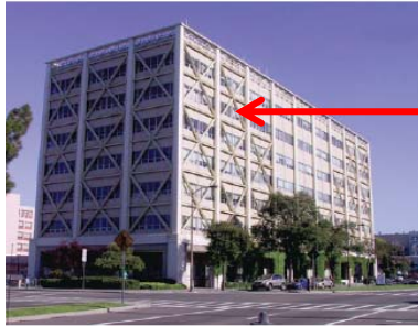
Steel braced frame on exterior of building to avoid construction on the building interior
