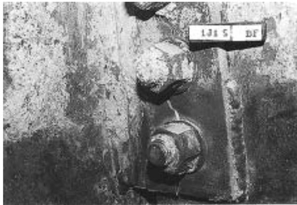
**Figure 1-5 Vertical Fracture through Beam Shear Plate Connection**
