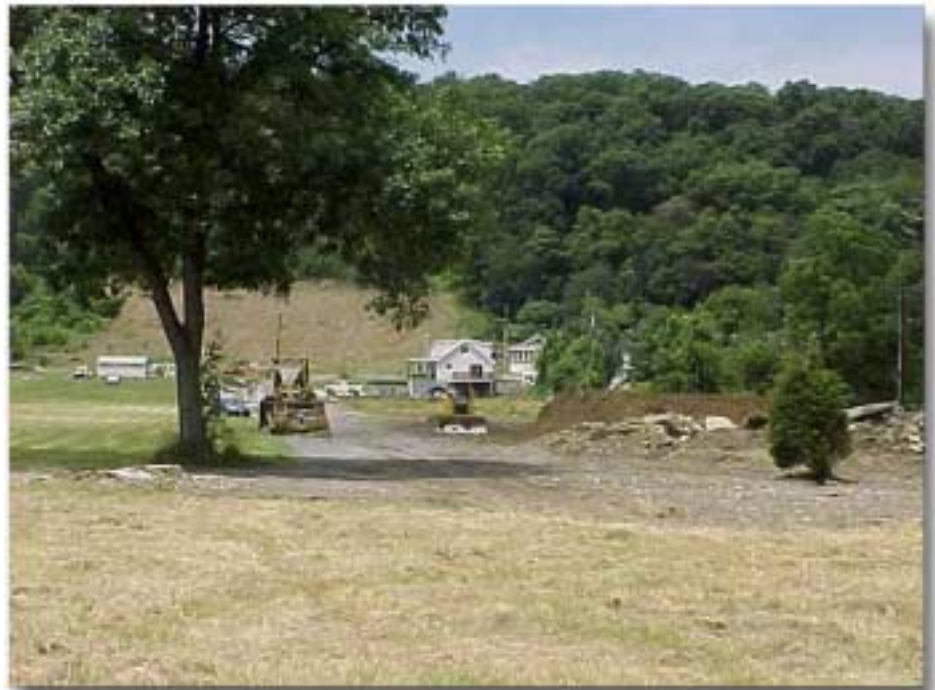
Relocation and land restoration in progress.
