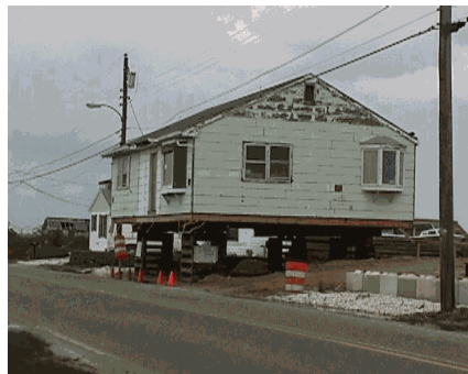
This house was recently moved to a new site at the end of Dock Road, close to the open bay. Homes pre-dating the Eagleswood Township Flood Damage Prevention Ordinance were not required to elevate. Today, projects such as this must comply with current elevation requirements.
