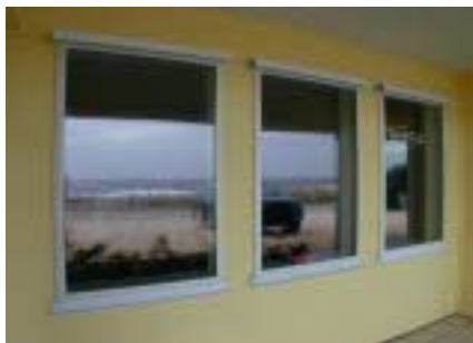
(Windows with extra strength glass and hurricane brackets pre-mounted)
