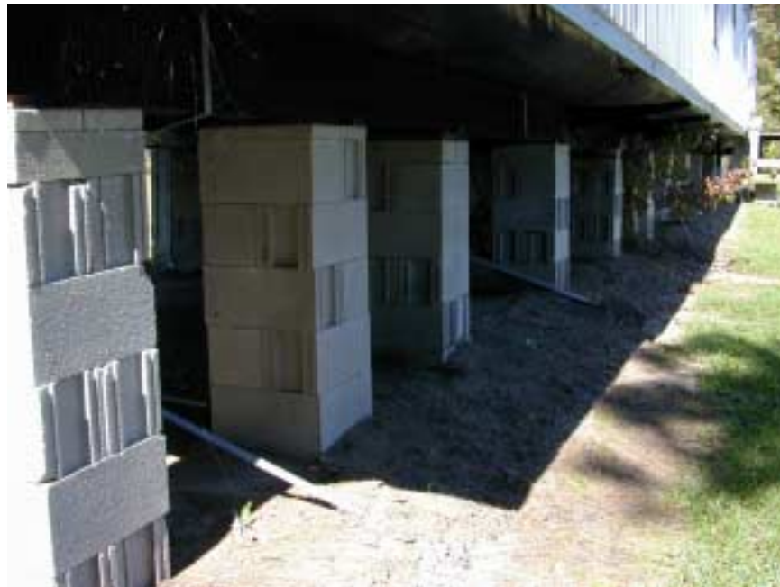
(Basic elevation using concrete blocks, it worked!)
