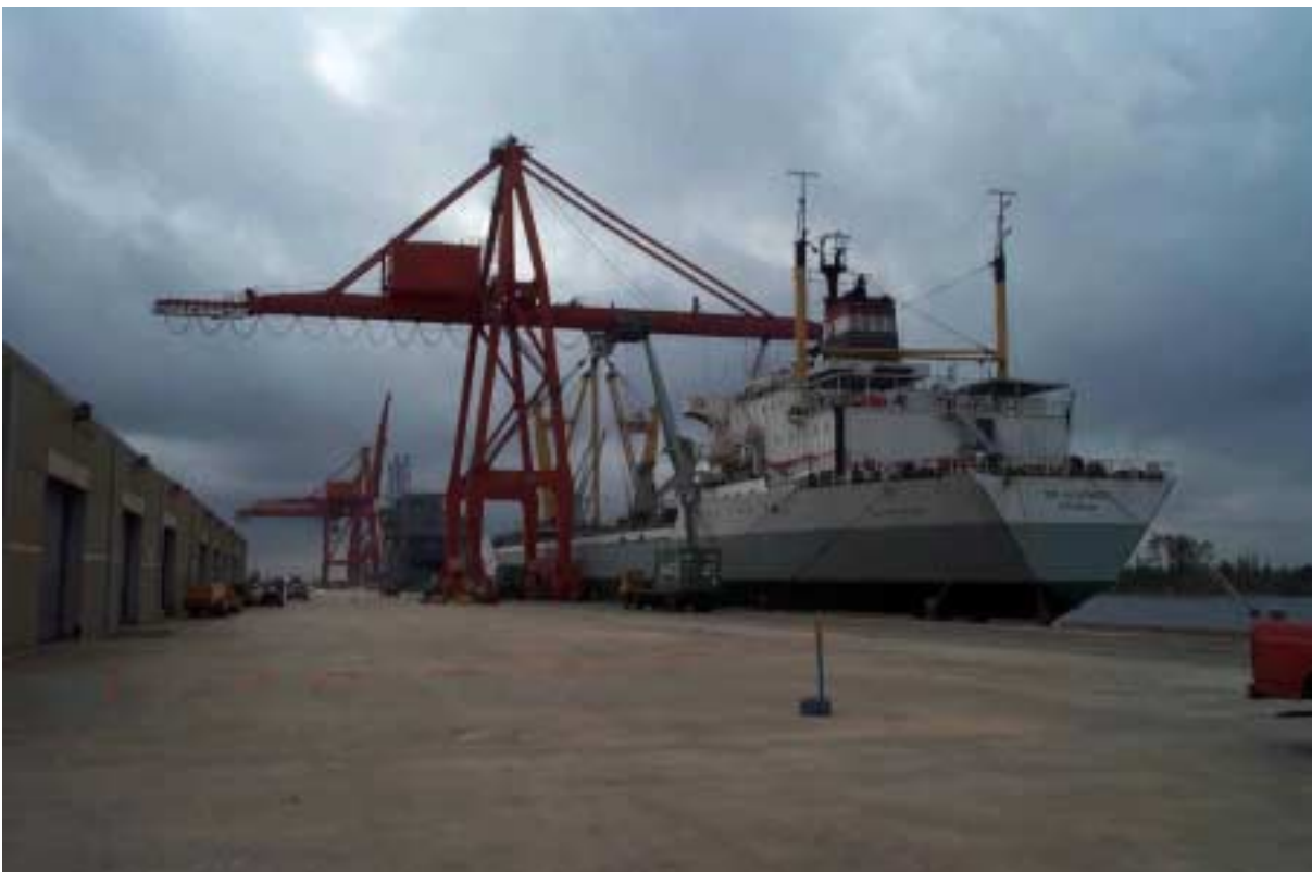
(Cranes used to move cargo at NCSPA are secured to prevent toppling during strong winds.)
