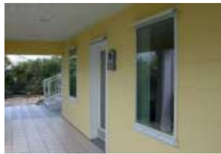
(Windows with extra strength glass and hurricane brackets pre-mounted)
