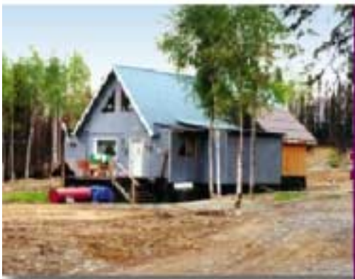
"Defensible space" around this home and a metal roof saved one of the few homes in Miller's Reach Wildfire in Alaska.
