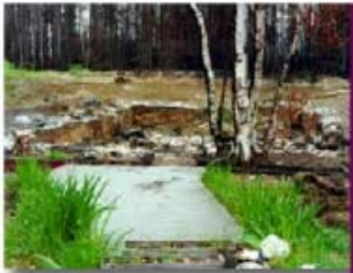
Like many of the 450 other structures, a foundation is all that remains of a two-story home that was nestled tight among the fire-fueling trees.
