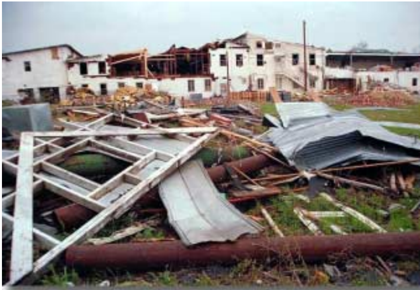
Oklahoma tornado damage
