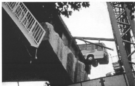
Freeway overpasses collapsed in Kobe, leaving this bus and other cars stranded.
