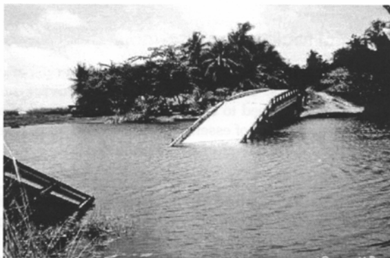
Oregon has over 4,000 bridges. This Costa Rican bridge failed during an earthquake.
