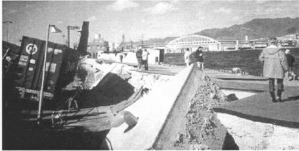
Properties along rivers, like port facilities, are especially vulnerable in an earthquake.
