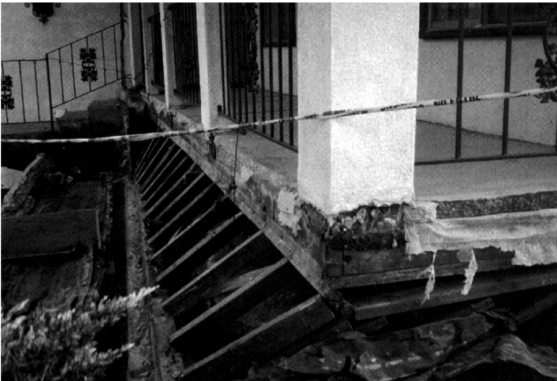
Figure 5. Cripple wall damage in the Northridge earthquake
