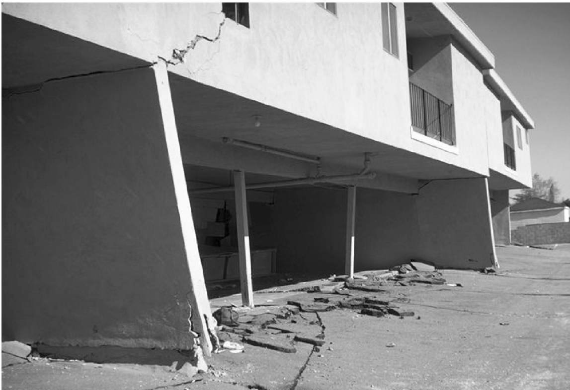
Figure 3. Damage to a tuck-under parking building with stucco shearwalls
