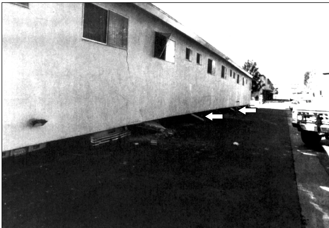
Figure 6. Damage to a tuck-under parking building in the Northridge earthquake.
