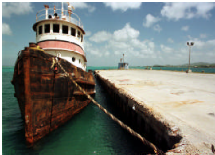
New fuel pier at Richmond Substation on St. Croix
