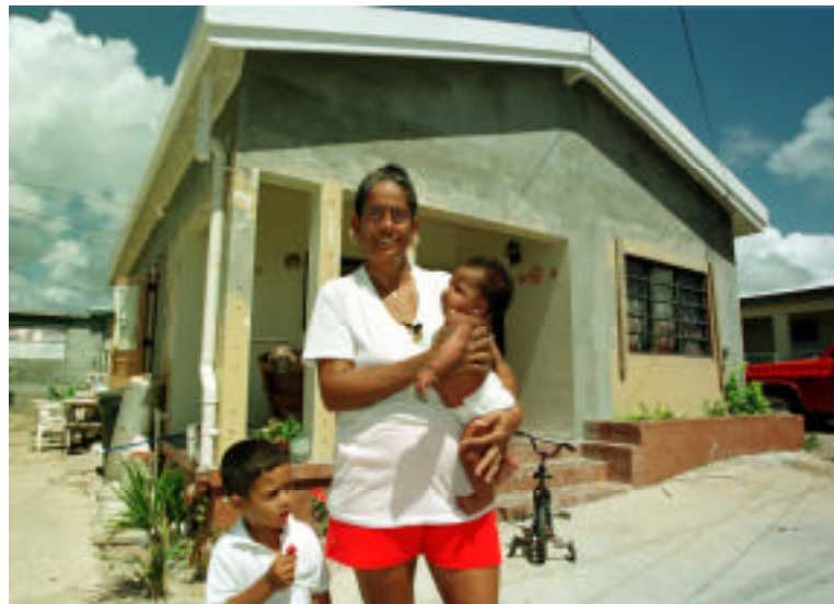
Homeowner stands in front of a newly constructed roof .
