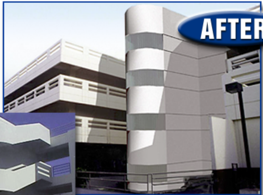
Guam Memorial Hospital before and after mitigation.
