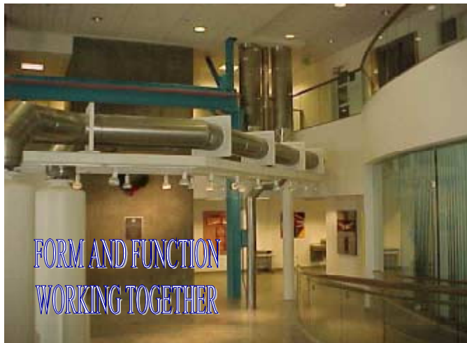
City of San Francisco Fire Department Station #1 Redesign and Retrofit—essential facility pipe bracing
