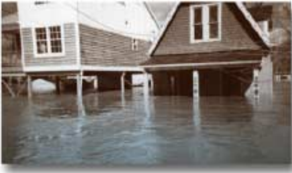
Homes inundated by flood waters.
