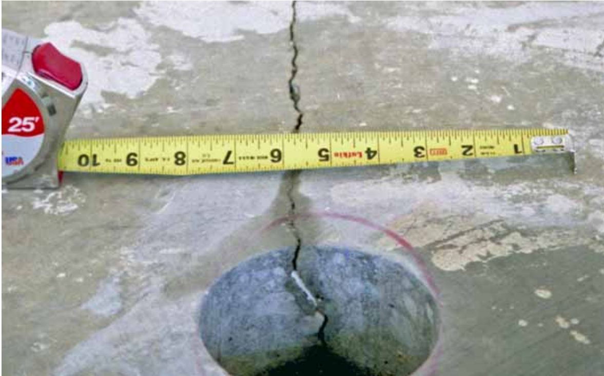
Figure 4.39. Linear shrinkage crack in concrete floor slab at location of a concealed control joint created by a “zip strip” [Exponent].
