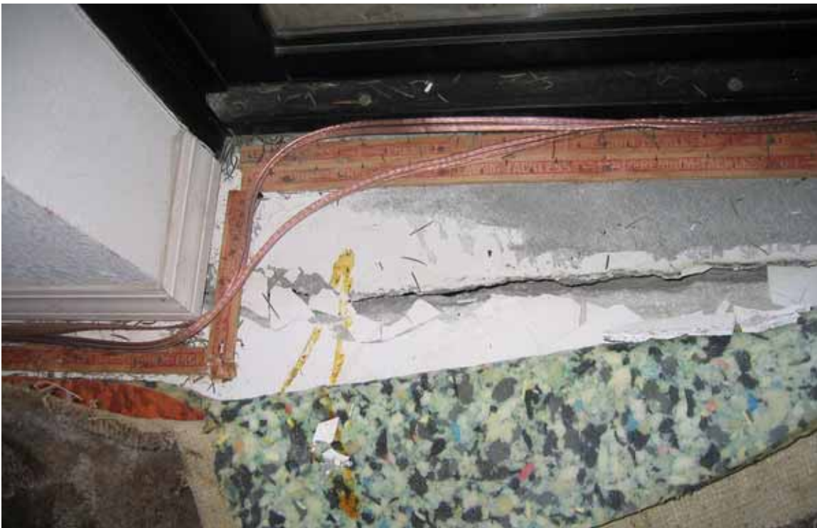
Figure 4.18. Opening of cold joint between floor slab and perimeter footing [Exponent].
