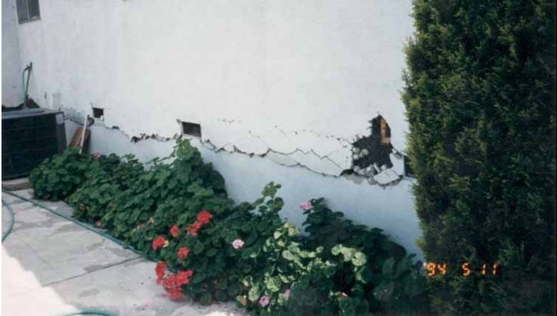
Figure 5.20. Earthquake-induced cracking and buckling of stucco at the plate line where stucco was extended onto the perimeter concrete stem wall [Exponent].
