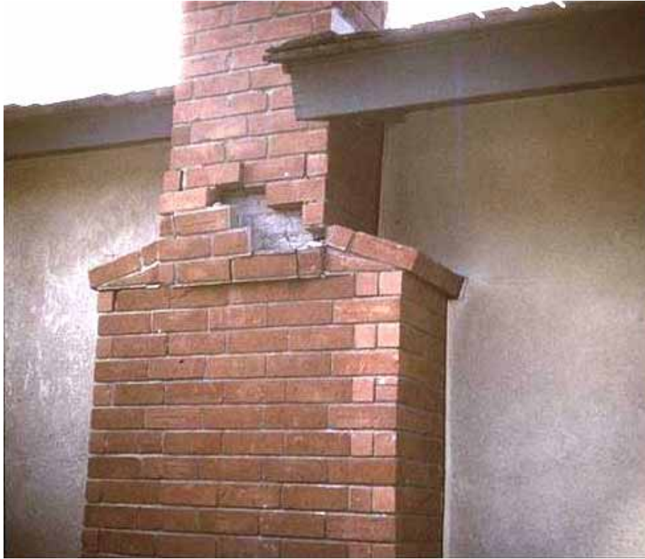
Figure 7.22. Damage to masonry chimney at shoulder.
