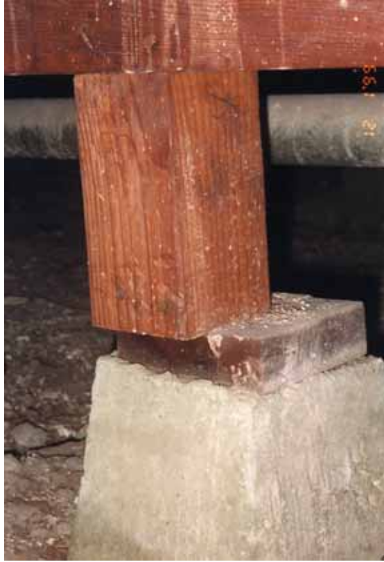
Figure 6.12. As-built misalignment between girder and footing accommodated with offset post (not earthquake damage) [Exponent].
