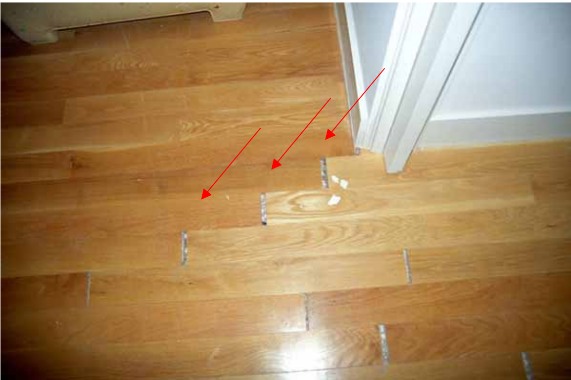
Figure 6.11. Gaps in flooring due to elongation of floor diaphragm caused by earthquake-induced slope movement [Exponent].
