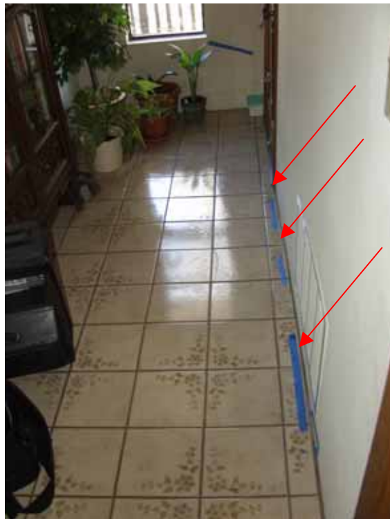
Figure 6.27. Earthquake-induced gap between floor and wall supported on retaining wall on uphill side of house on sloped lot [Exponent].
