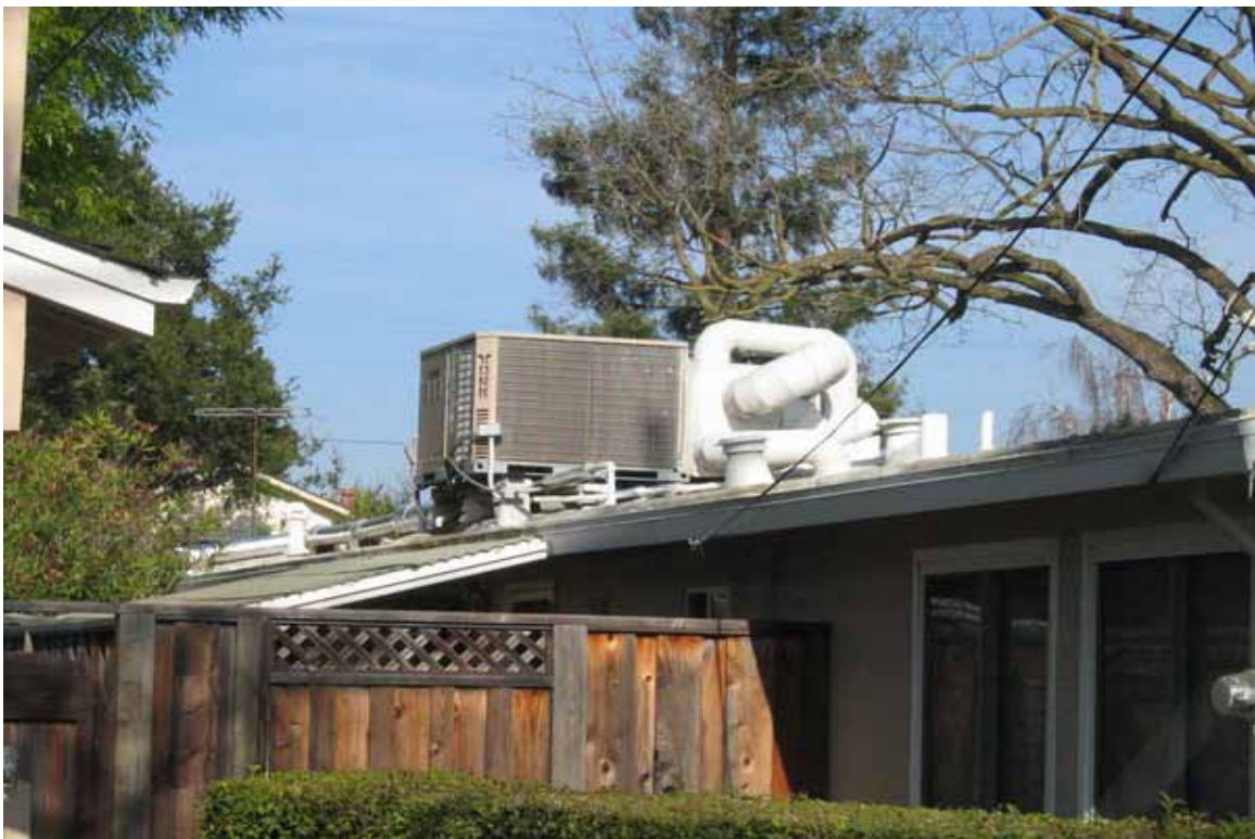
Figure 8.7. Rooftop HVAC unit (no damage) [Exponent].
