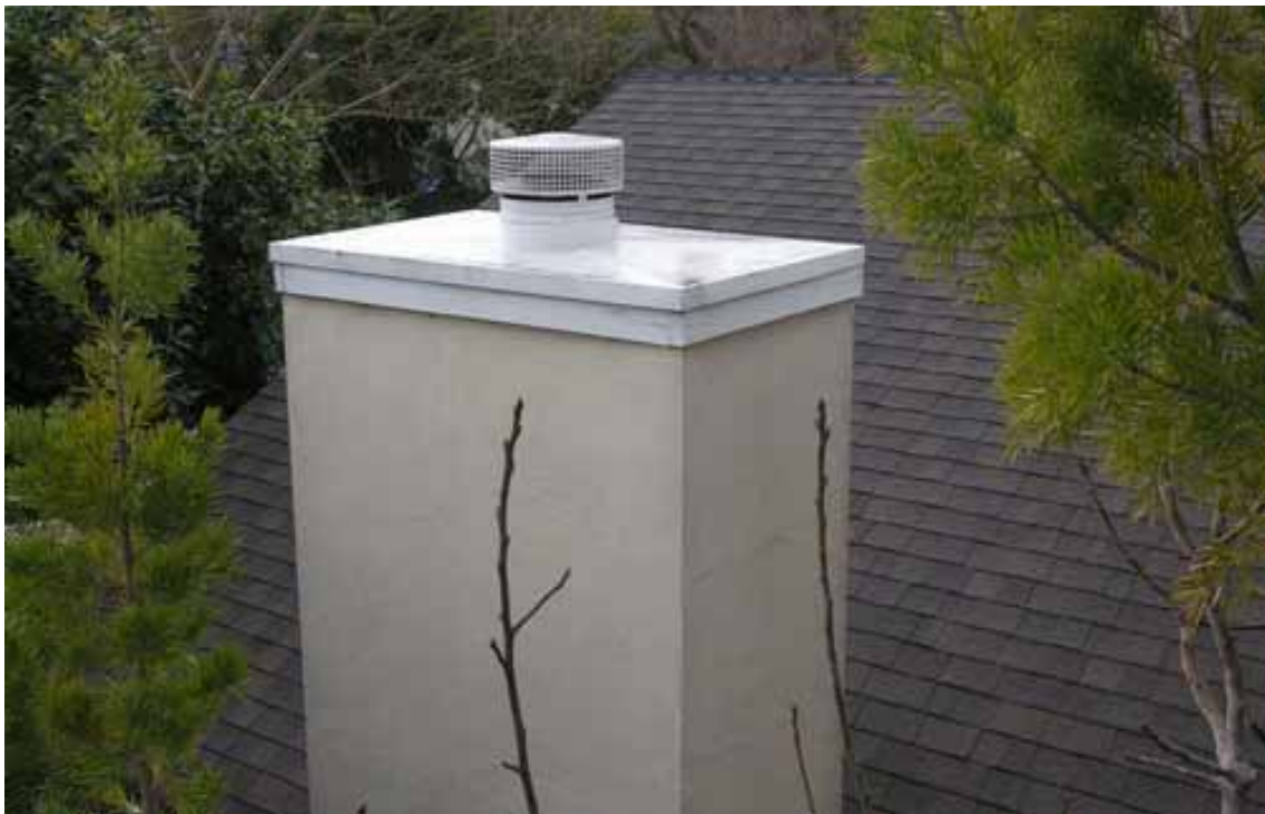
Figure 7.8. Stucco-clad, woodframed chimney chase (no damage) [Exponent].
