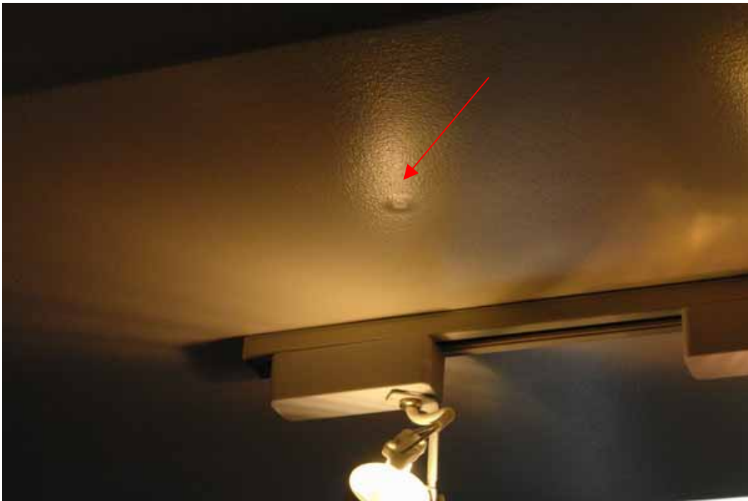
Figure 6.7. Nail pop visible in ceiling (not earthquake damage) [Exponent].
