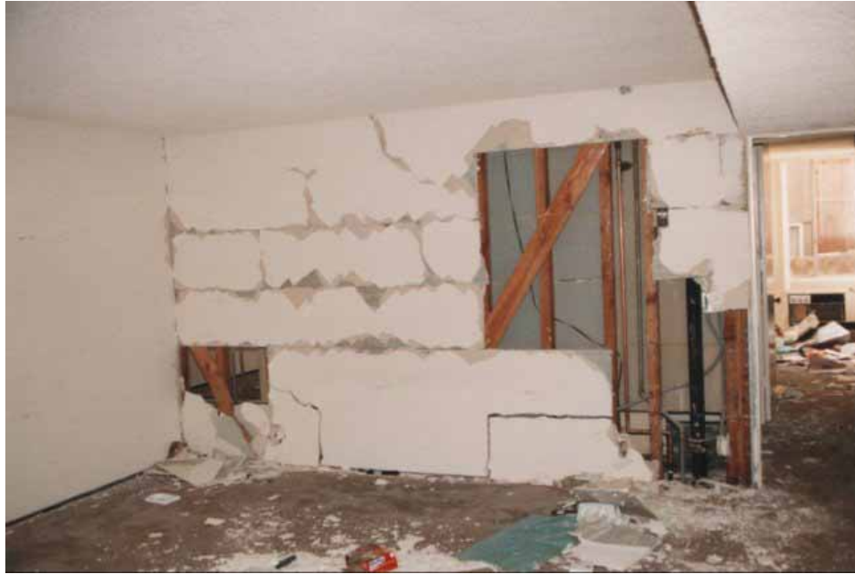
Figure 5.18. Earthquake-induced cracking and delamination of gypsum lath and plaster [Exponent].
