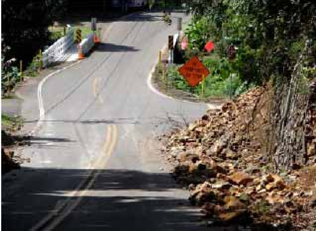
Figure 3.23. Rockfall on a road cut at northern end of North Kohala from 2006 Hawaii Earthquakes [UHM].
