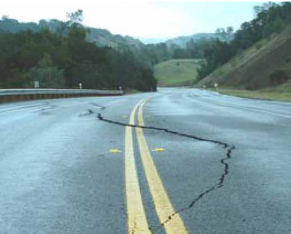
Figure 3.28. Asphalt pavement cracking along SR 46 as a result of a deep rotational slope failure in fill during the 2003 San Simeon Earthquake [EERI].
