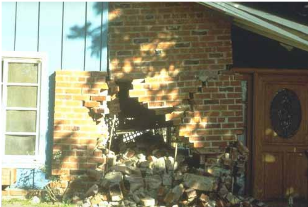
Figure 7.16. Failure of masonry fireplace at firebox level caused by 1994 Northridge Earthquake [Reitherman].
