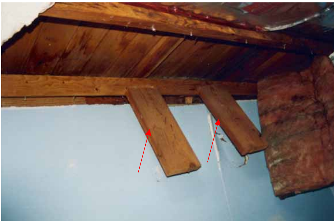
Figure 6.24. Significant earthquake damage to finishes where framing has failed (arrows identify blocking attached to chimney strap) [Exponent].
