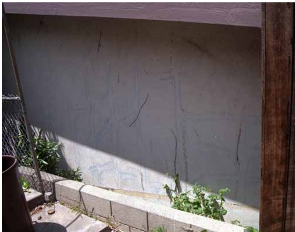
Figure 5.7. Roughly linear vertical non-earthquake shrinkage cracks corresponding to the locations of underlying studs; crack locations have been highlighted with parallel lines of blue chalk [Exponent].
