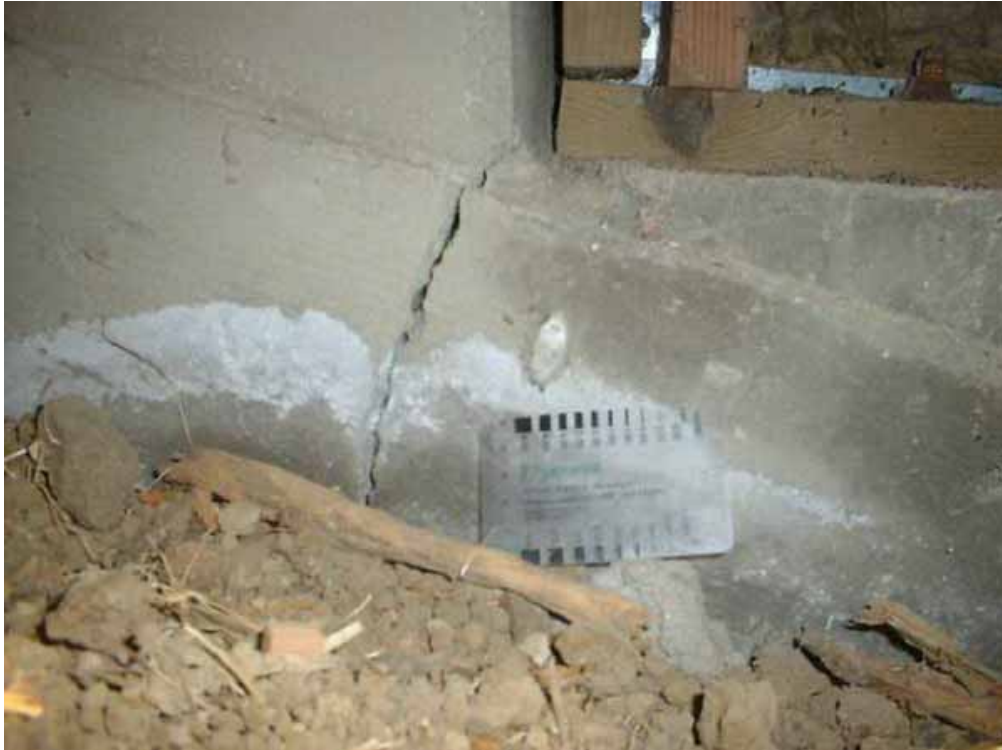
Figure 4.9. Concrete shrinkage crack emanating from reentrant corner at a step in a perimeter stem wall [Exponent].
