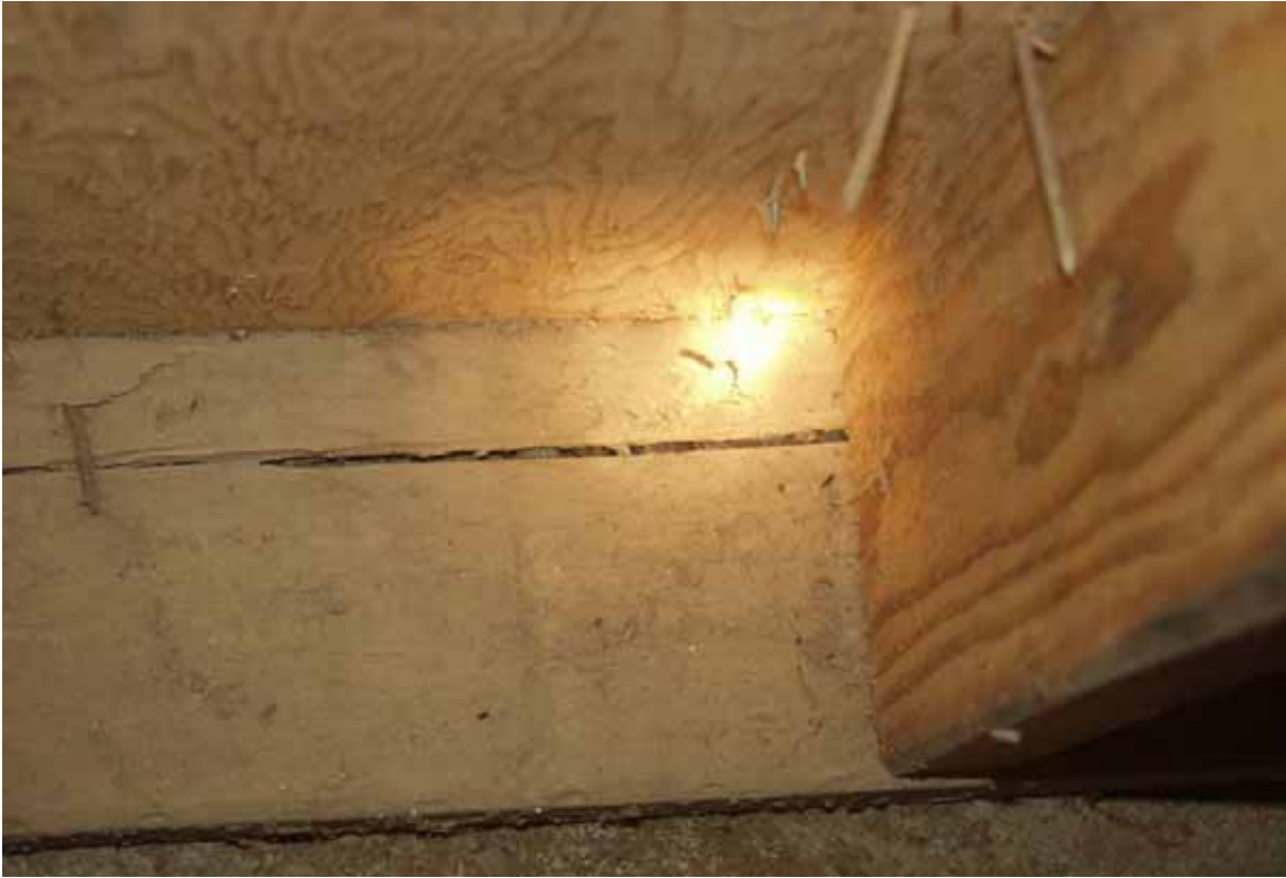
Figure 6.10. Cracked mudsill and missed nails (not earthquake damage) [Exponent].
