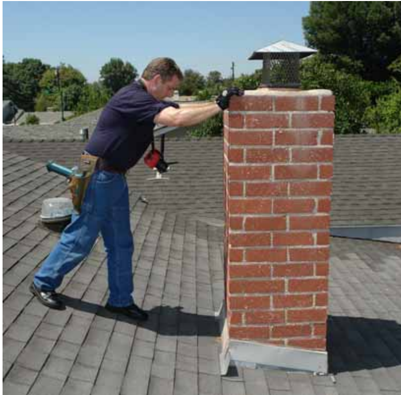
Figure 7.32. Illustration of rocking procedure for checking for chimney for earthquake-induced cracking [Exponent].
