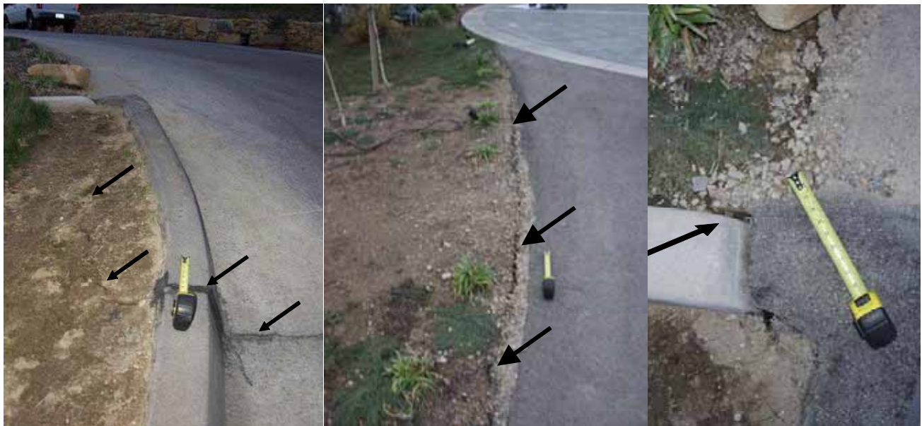
Figure 3.35. Driveway cracking following the 2003 San Simeon Earthquake; arrows indicate pavement cracking (top and bottom left), ground cracking (bottom), and offset in curb (bottom right) [Exponent].
