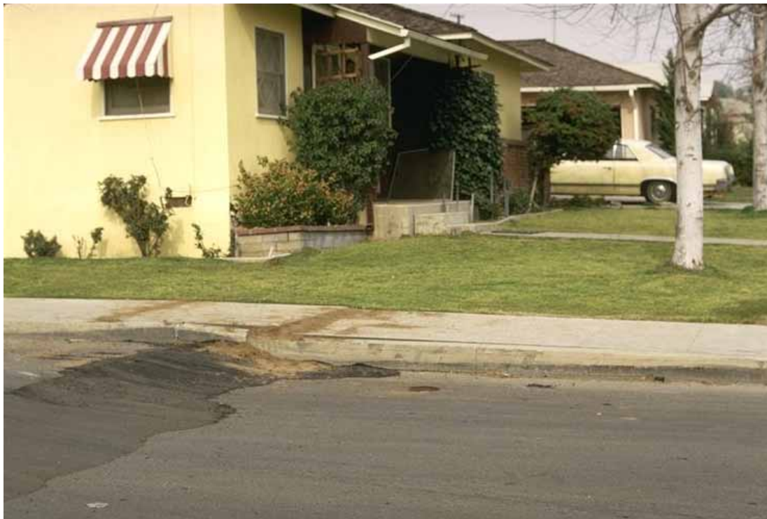
Figure 3.30. Pavement patching and damage to adjacent sidewalk in City of San Fernando following the 1971 San Fernando Earthquake [NISEE].
