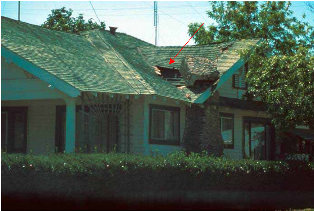
Figure 6.18. Earthquake damage from impact of falling masonry chimney [USGS].
