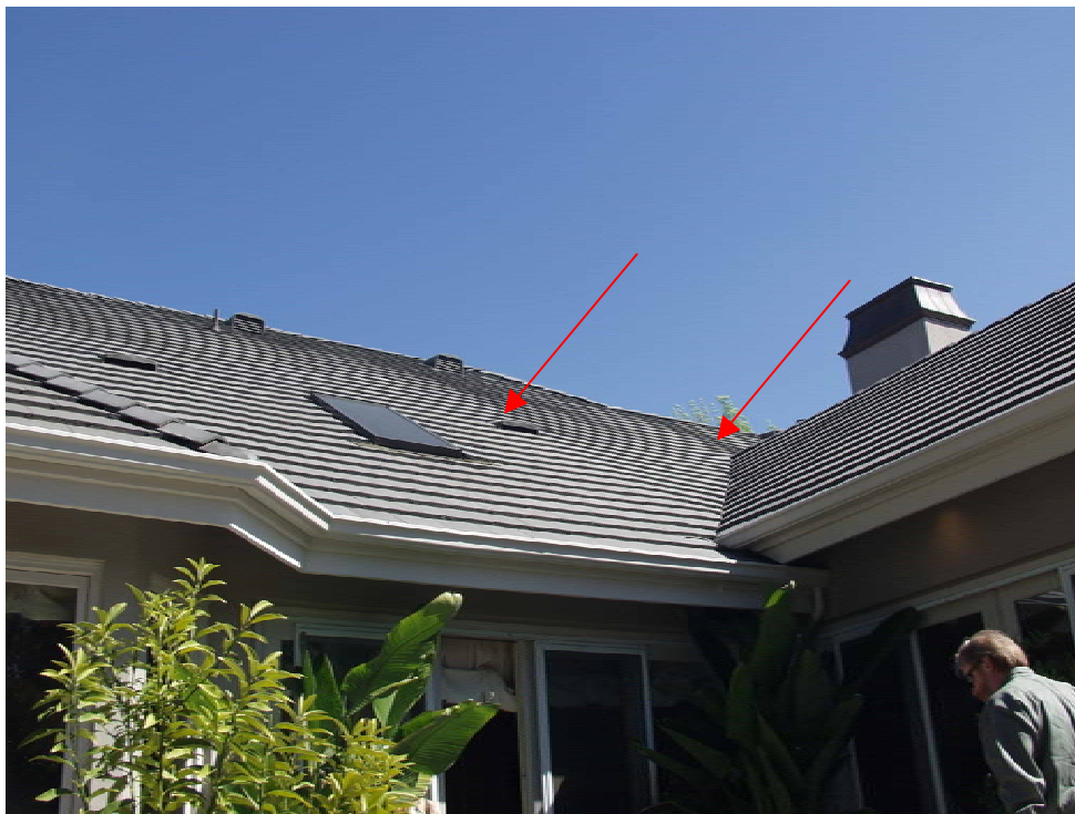
Figure 6.3. Heavy tile roof sags between wall supports, located by arrows (not earthquake damage) [Exponent].
