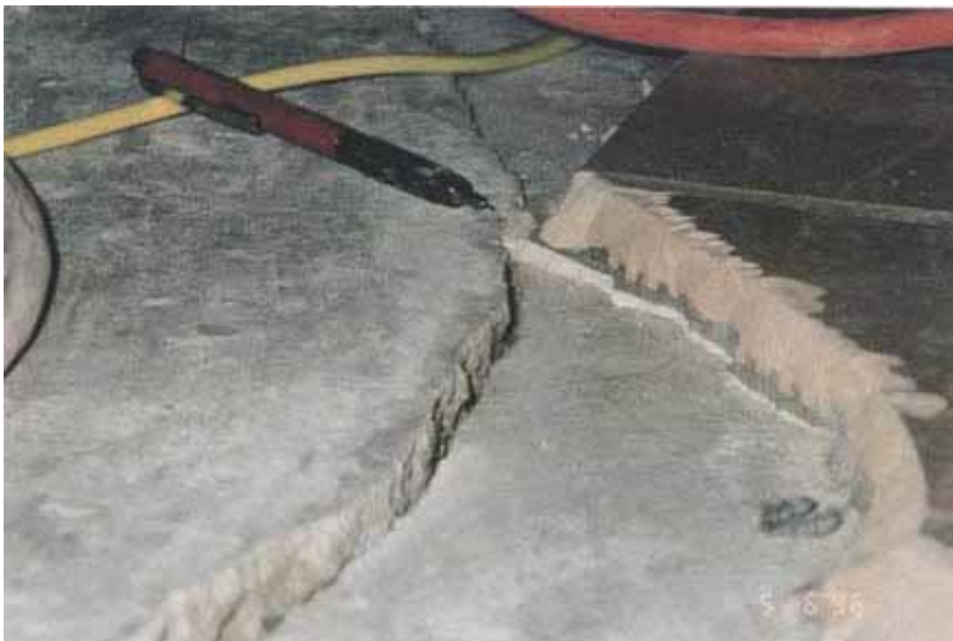
Figure 4.35. Grout completely filling slab-on-grade crack (indicated by pen) indicates that slab crack was present at the time of the tile installation and has not experienced movement since tile installation (not earthquake damage) [Exponent].
