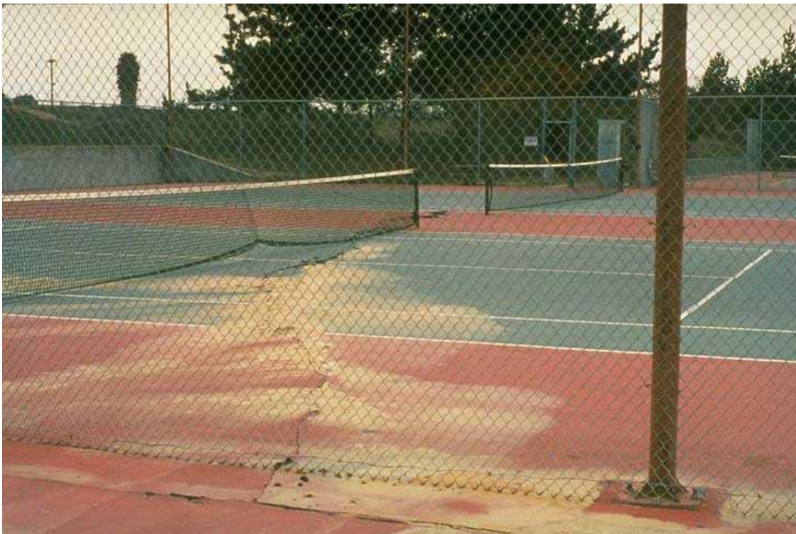
Figure 3.14. Tennis court damage with ejection of wet sand from soil liquefaction (site is adjacent to a river) during the 1989 Loma Prieta Earthquake [NISEE].
