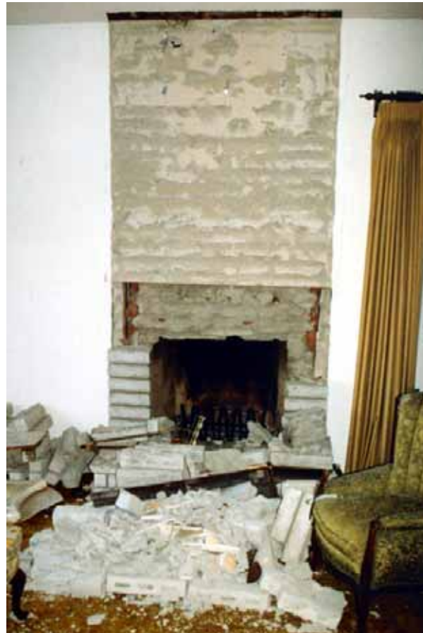
Figure 7.31. Collapsed masonry facing during the 1994 Northridge Earthquake [Exponent].
