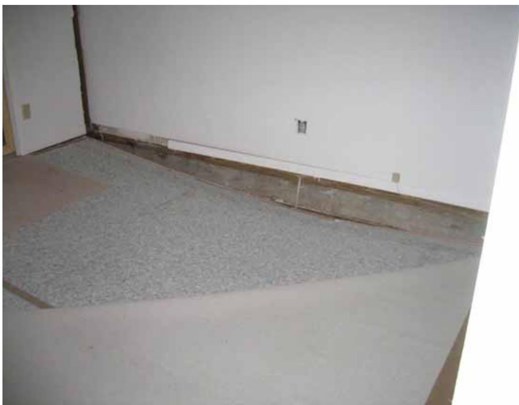
Figure 6.25. Sagging floor due to earthquake-induced shifting and loss of support [Exponent].
