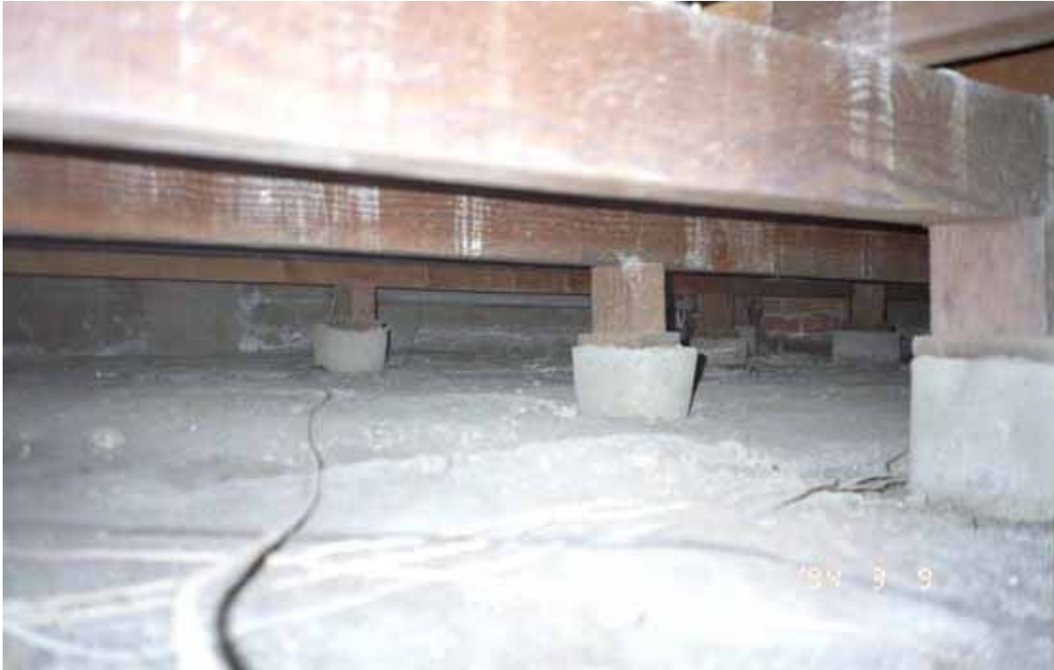
Figure 4.5. Undamaged isolated footings supporting wood posts of first floor woodframing [Exponent].
