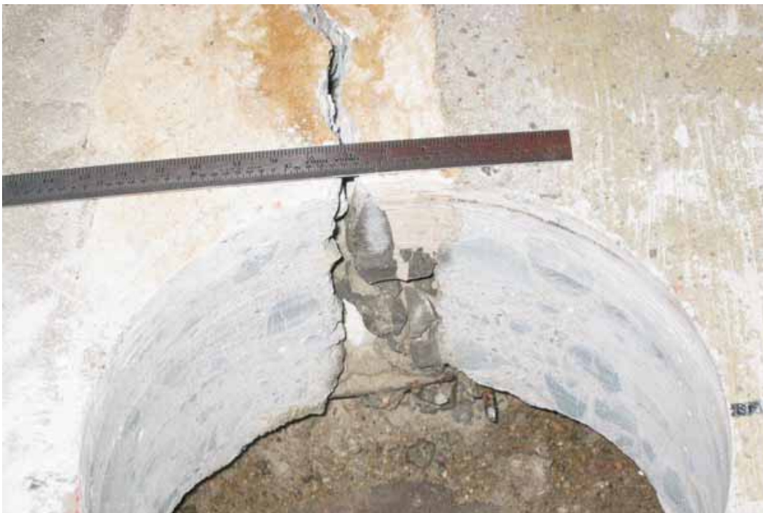
Figure 4.30. Crack in concrete slab-on-grade floor that exhibits two prior generations of patching as well as opening since last patching (not earthquake damage) [Exponent].
