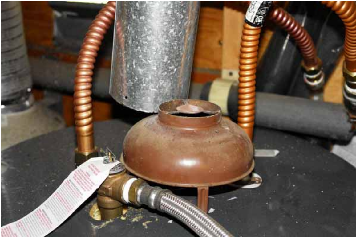
Figure 8.4. Displacement of unsecured water heater vent during 1989 Loma Prieta Earthquake [Exponent].
