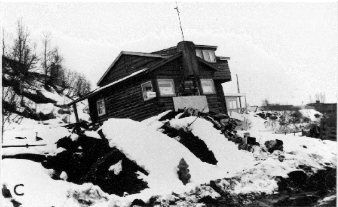
Figure 3.20. House displaced by large blocks of soil uplifted at toe of L Street landslide, Anchorage district, during the 1964 Anchorage, Alaska Earthquake [USGS].
