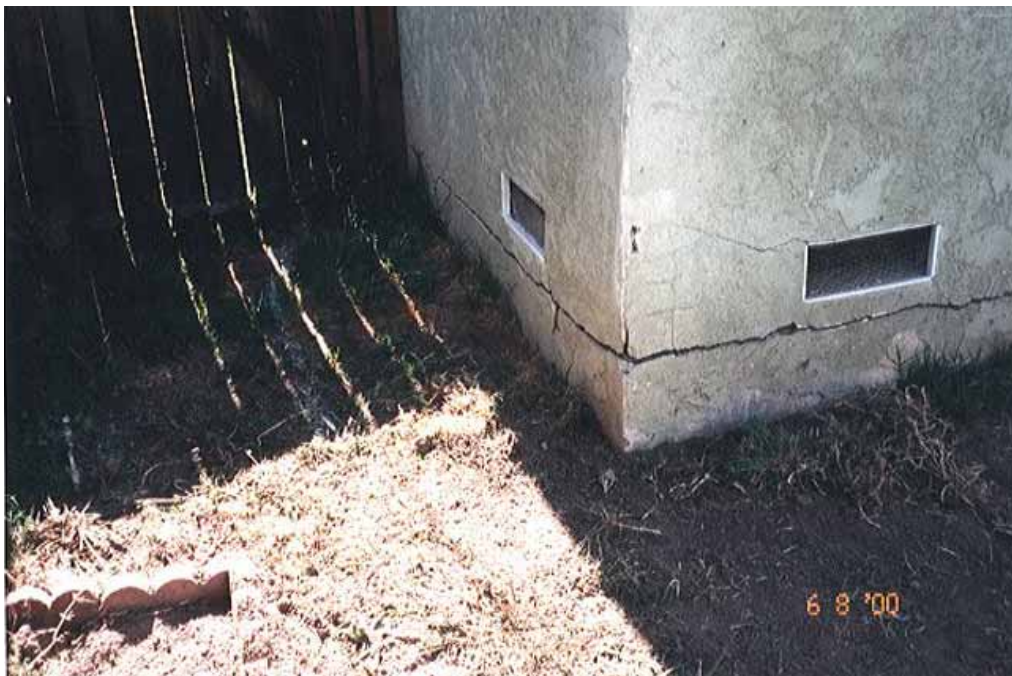
Figure 5.16. Earthquake-induced crack in stucco at sill line where stucco was extended down over the foundation, as commonly done prior to the early 1970s (concealed framing is raised wood floor over continuous perimeter concrete stem wall) [Exponent].
