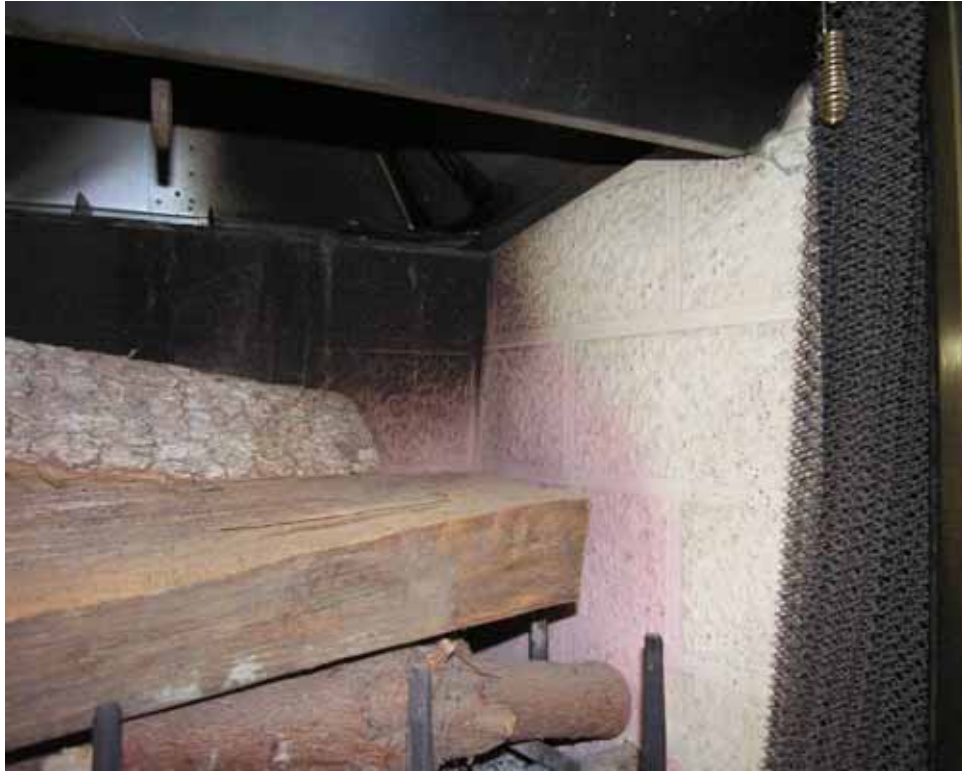
Figure 7.9. Firebox of factory-built fireplace with brick patterned refractory panels (no damage) [Exponent].
