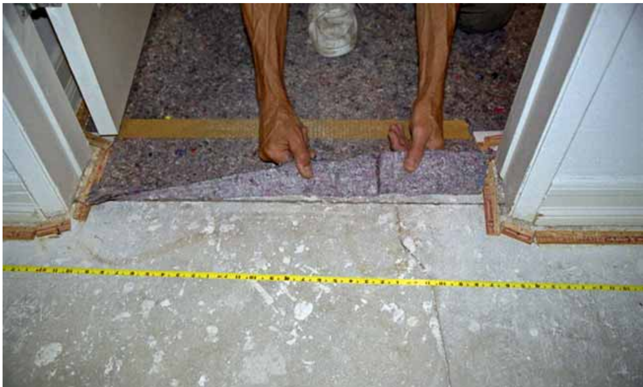
Figure 6.13. Shrinkage cracks in lightweight concrete fill (not earthquake damage) [Exponent].
