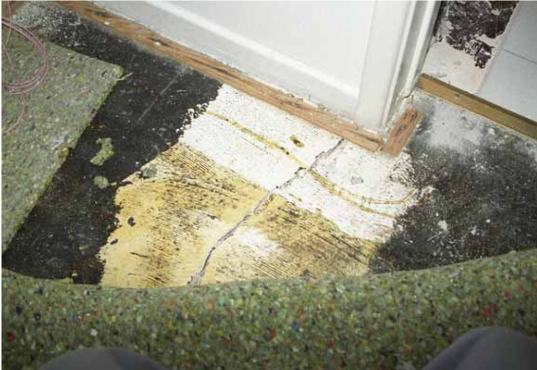
Figure 4.31. White leveling compound spread across existing crack at time of carpet installation [Exponent].
