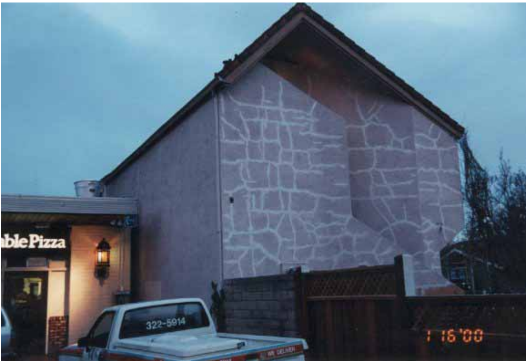
Figure 5.6. Semi-random, semi-orthogonal grid work of non-earthquake shrinkage cracks in stucco – note that cracks are highlighted by patching material applied in the course of repainting the building [Exponent].
