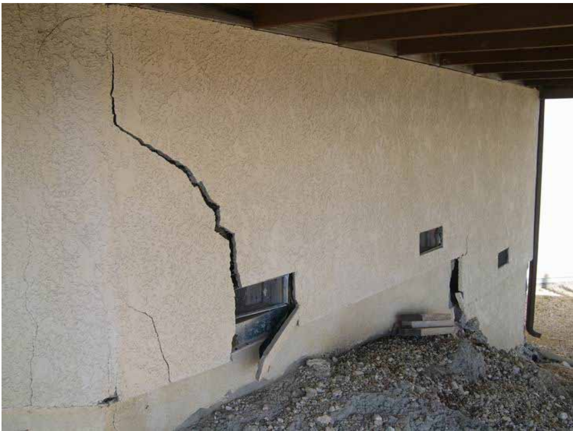
Figure 5.21. Stucco cracking and buckling at cripple wall following the 2003 San Simeon Earthquake [Exponent].
