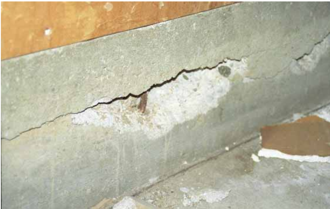
Figure 4.16. Earthquake-induced differential movement and spalling at cold joint between stem wall and slab in two-pour construction [Exponent].
