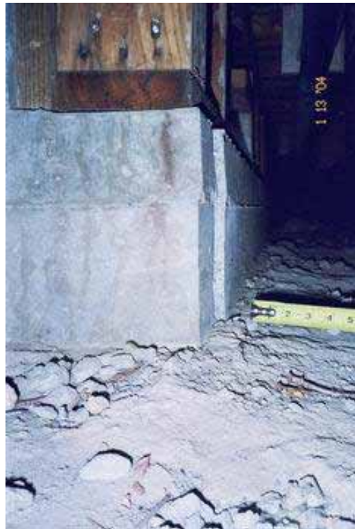
Figure 3.47. Foundation and ground cracking following the 2003 San Simeon Earthquake; bottom shows the out-of-plane offset present across foundation crack shown in top photograph [Exponent].
