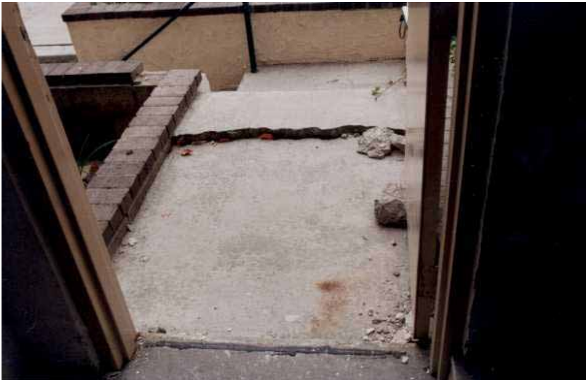
Figure 3.39. Dropping of entry walkway supported on poorly compacted backfill during the Northridge Earthquake [Exponent].
