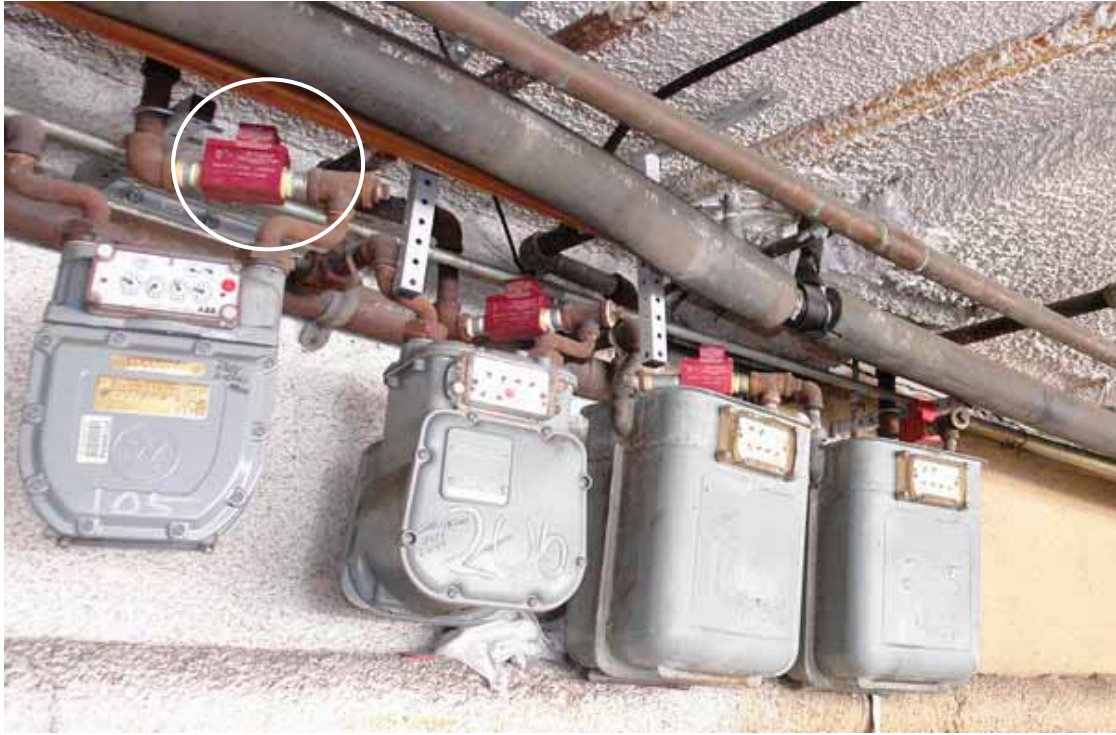
Figure 8.1. Gas meters with seismic shut-off valves [Exponent].
