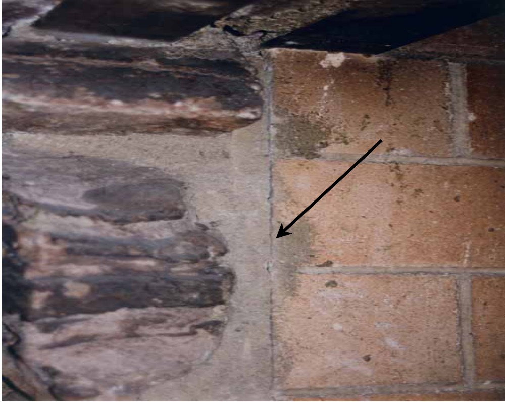
Figure 7.15. Mortar joint between firebox and masonry facing where hairline cracks are frequently found (not earthquake damage) [Exponent].
