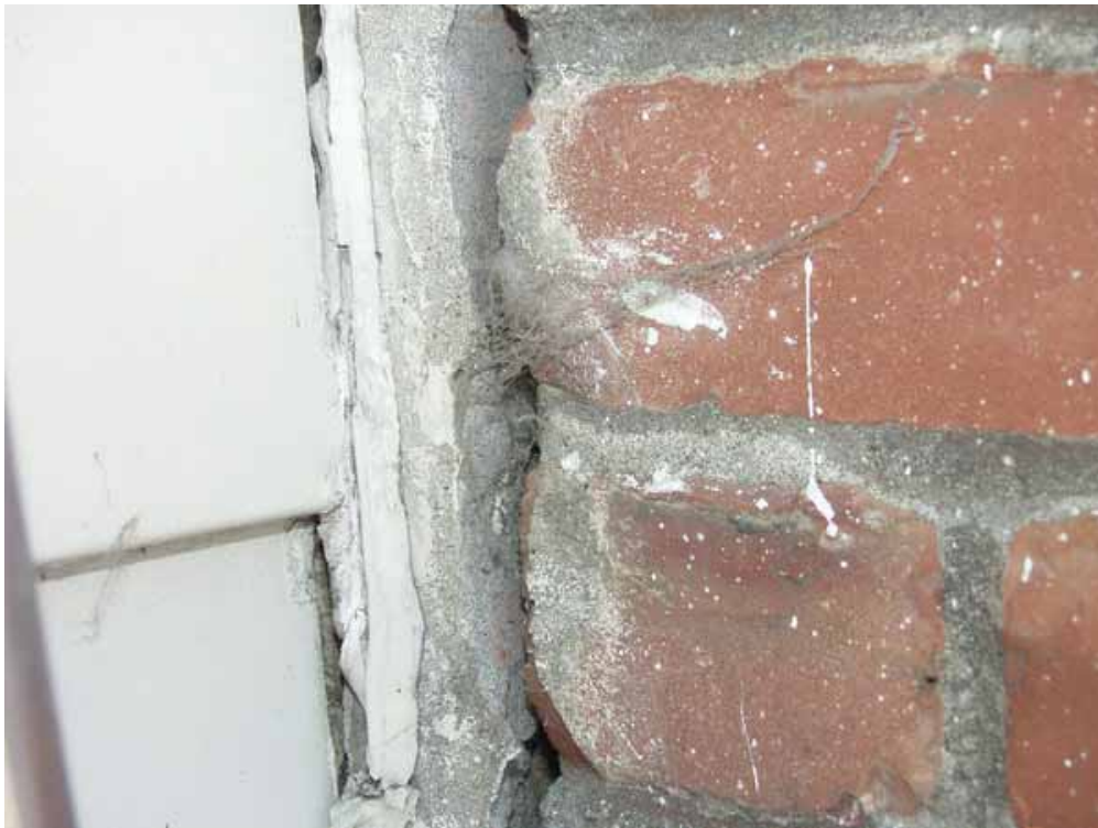
Figure 7.12. Gap between chimney and house – note mortar filler used to fill previous gap, movement since that repair, paint in gap, cobweb spanning gap (not earthquake damage) [Exponent].
