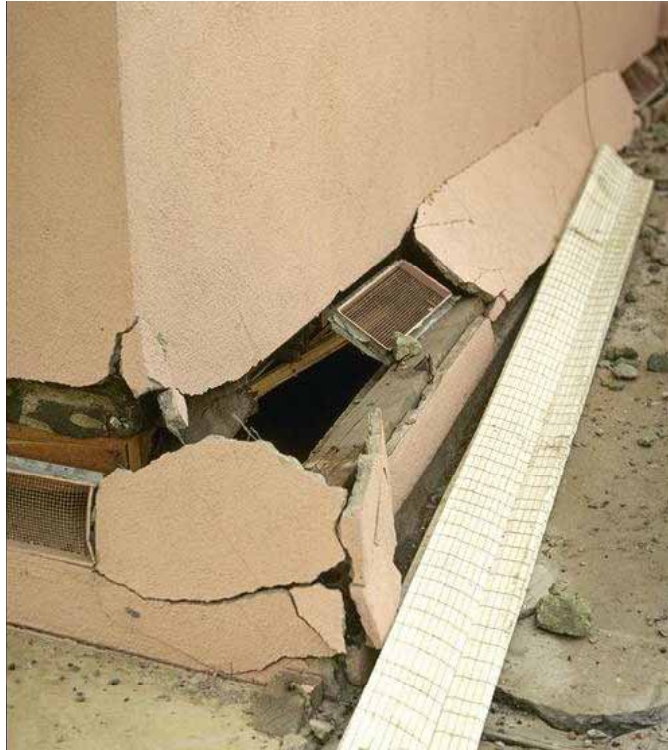
Figure 6.26. Sliding of joists on mudsill due to earthquake [NISEE].
