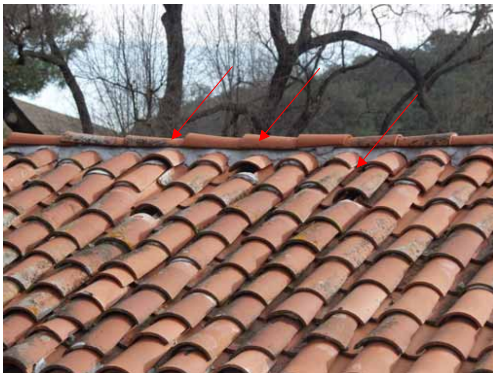
Figure 6.16. Clay roof tile and mortar joints shifted by earthquake shaking [Exponent].
