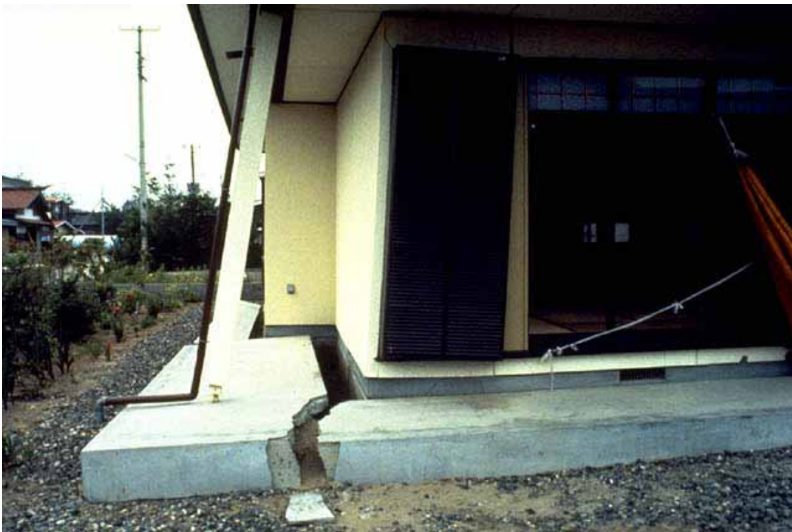
Figure 3.45. Damage from lateral spreading to house foundation in Wakami, Japan during the 1983 Nihonkai-Chubu Earthquake [NISEE].
