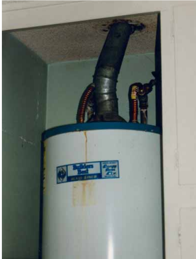
Figure 8.11. Flexible piping between unsecured water heater and house piping (no damage) [Exponent].
