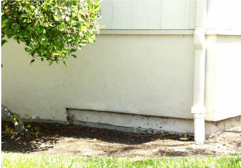
Figure 5.9. Stucco terminated at weep screed on mudsill of recent addition (right) juxtaposed with stucco extended down onto the original foundation (left), as was commonly done prior to the early 1970s – slab-on-grade floor with continuous perimeter footings shown (not earthquake damage) [Exponent].
