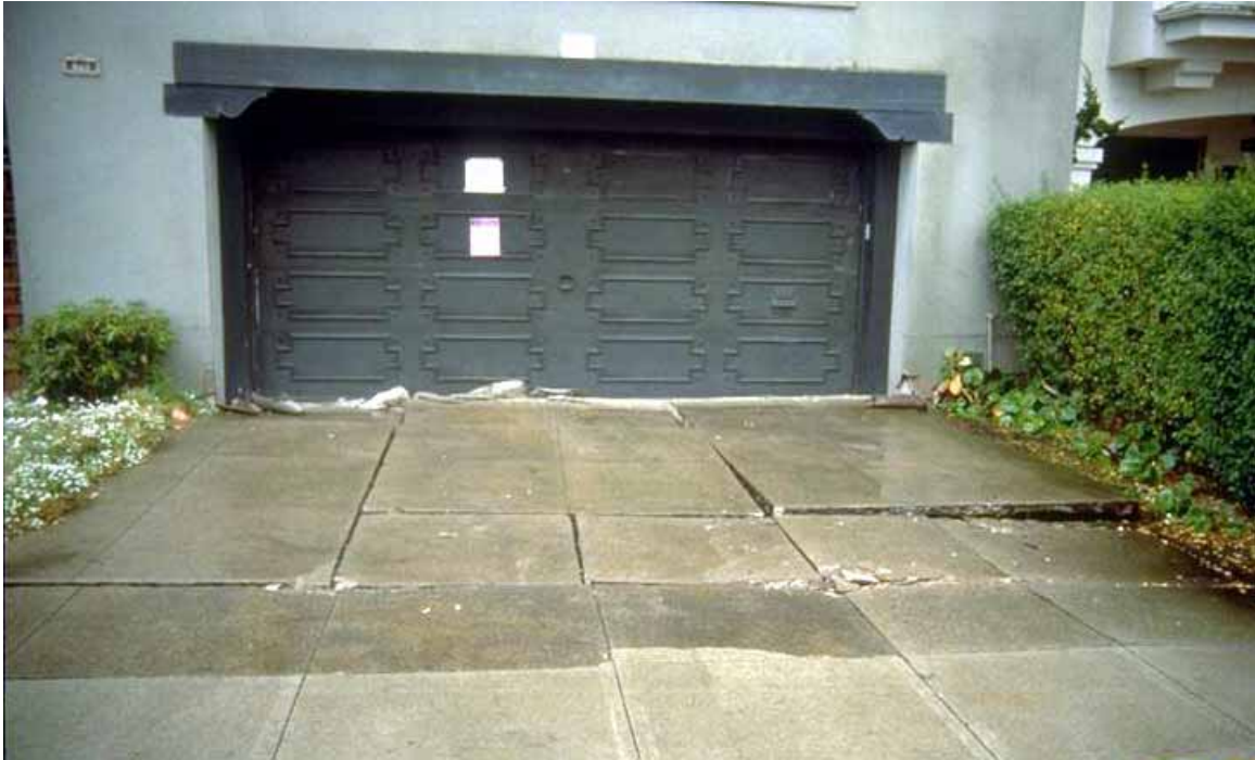
Figure 3.36. Driveway cracking and differential settlement following the 1989 Loma Prieta Earthquake [NISEE].
