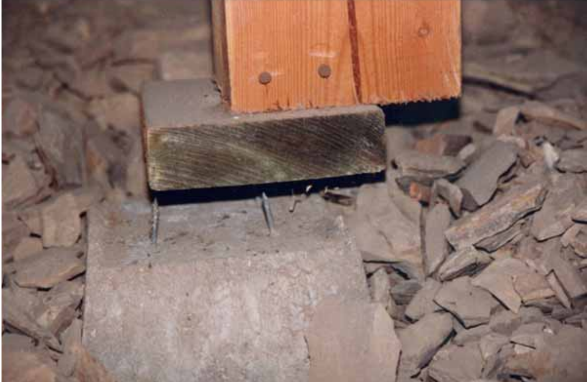
Figure 6.8. Gap between post and pier foundation in crawlspace (not earthquake damage) [Exponent].
