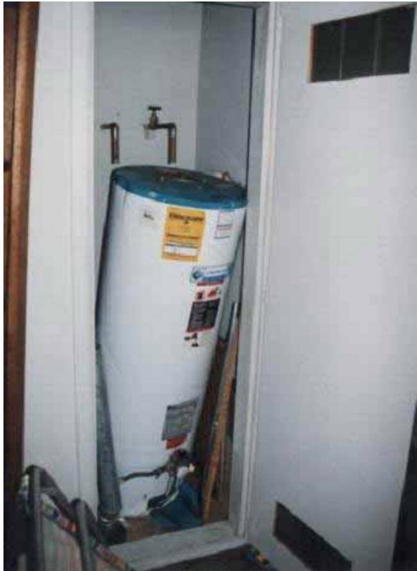
Figure 8.3. Displacement of unsecured water heater during 1994 Northridge Earthquake [Exponent].
