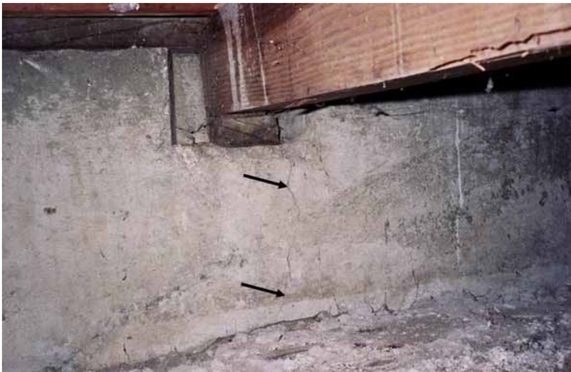
Figure 4.11. Shrinkage crack in a concrete stem wall emanating from a beam pocket [Exponent].
