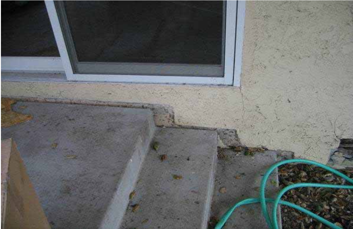
Figure 3.38. Concrete porch and steps offset from original position by earthquake-induced permanent ground deformation as evidenced by exposed foundation concrete [Exponent].
