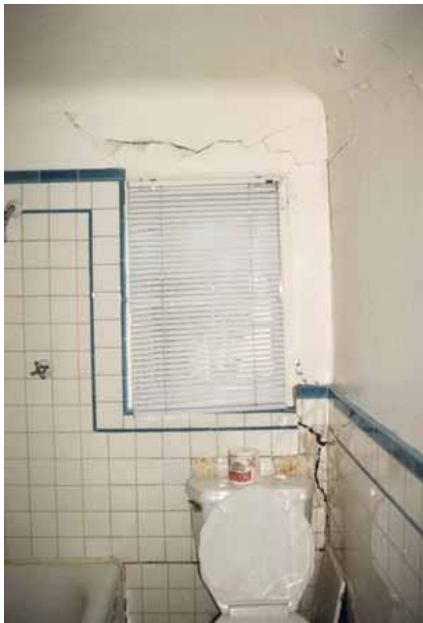
Figure 5.19. Earthquake-induced cracking of ceramic tile [Exponent].
