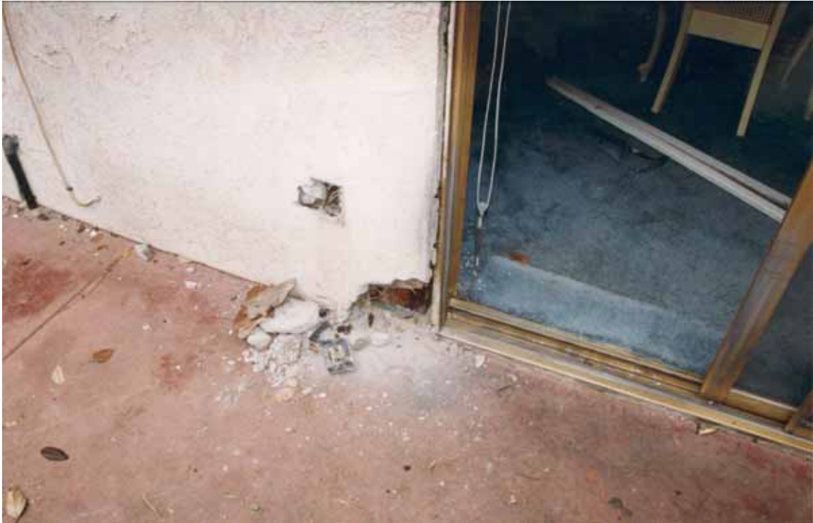
Figure 8.8. Racking and delamination of exterior stucco resulting in damage to electrical outlet during 1994 Northridge Earthquake [Exponent].
