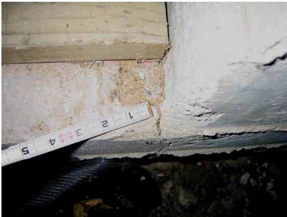
Figure 4.32. Debris (sawdust) from original construction in foundation crack observed shortly following the 2003 San Simeon Earthquake (not earthquake damage) [Exponent].
