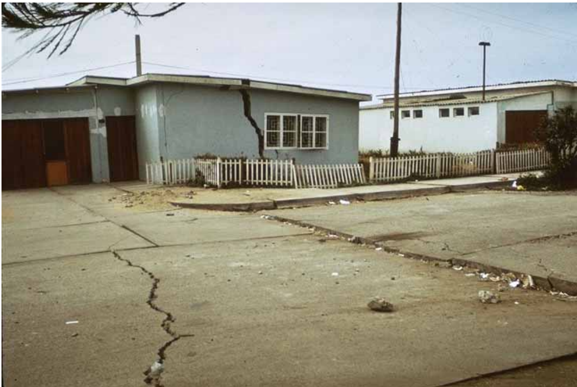
Figure 3.34. Projection of liquefaction-induced ground cracking through a building in the city of Chimbote during the 1970 Peru Earthquake [NISEE].
