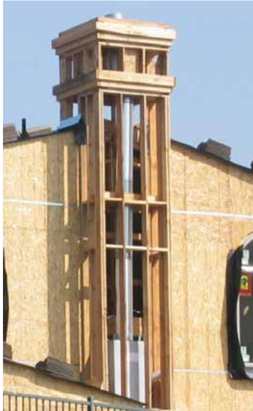
Figure 7.7. Factory-built fireplace and metal flue in woodframe chase during construction (no damage) [Exponent].
