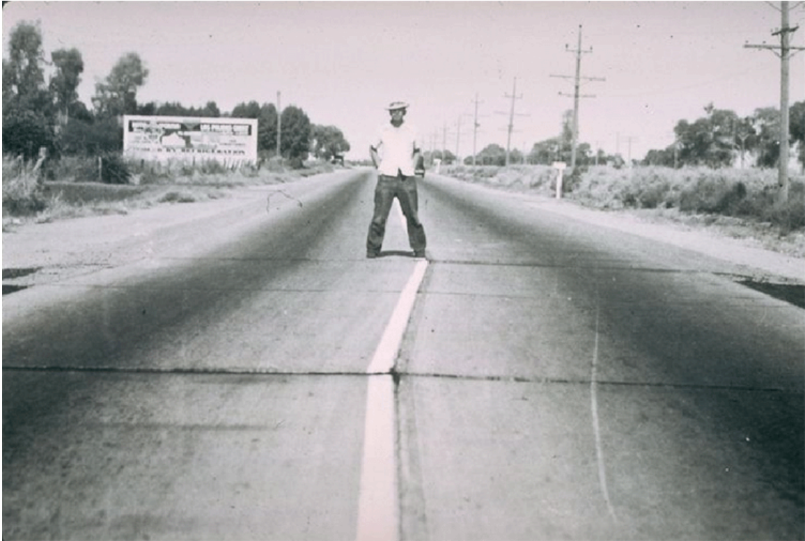
Figure 3.11. Surface faulting midway between El Centro and Holtville from the 1940 El Centro, California Earthquake [NISEE].
