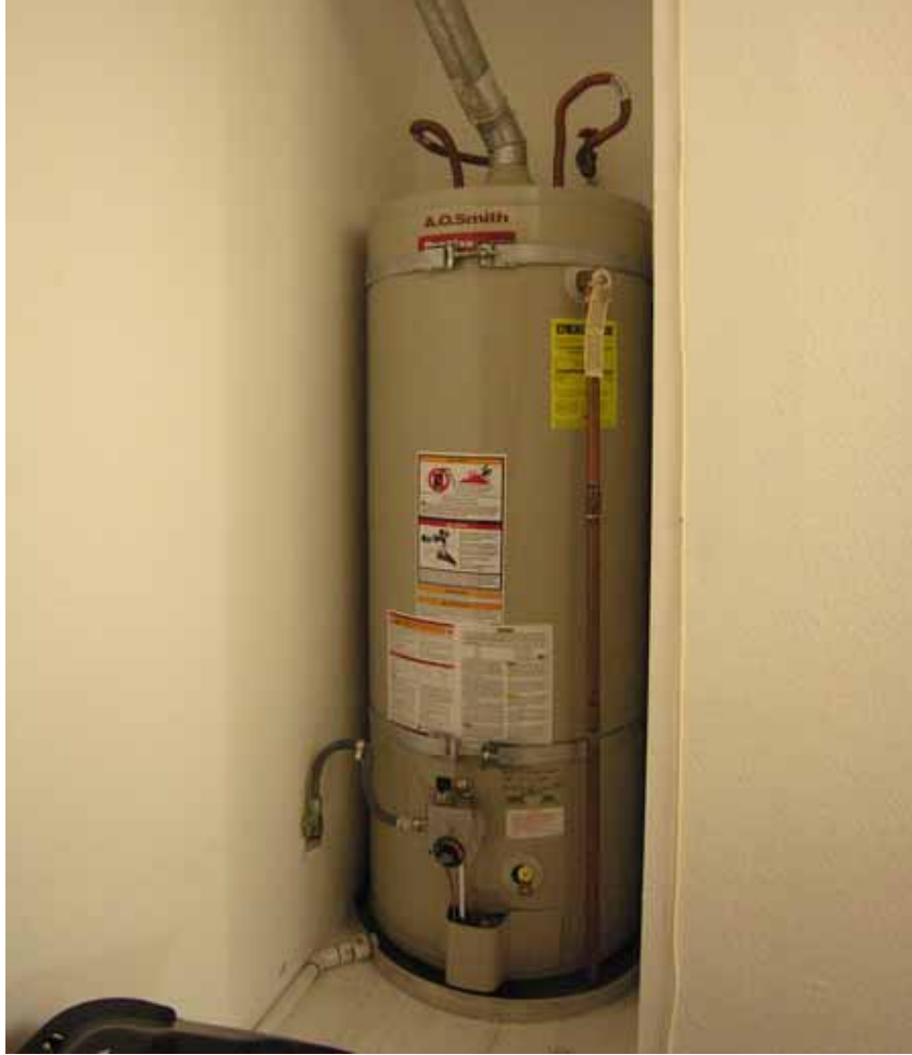
Figure 8.10. Water heater with flexible piping and securing strapping (no damage) [Exponent].
