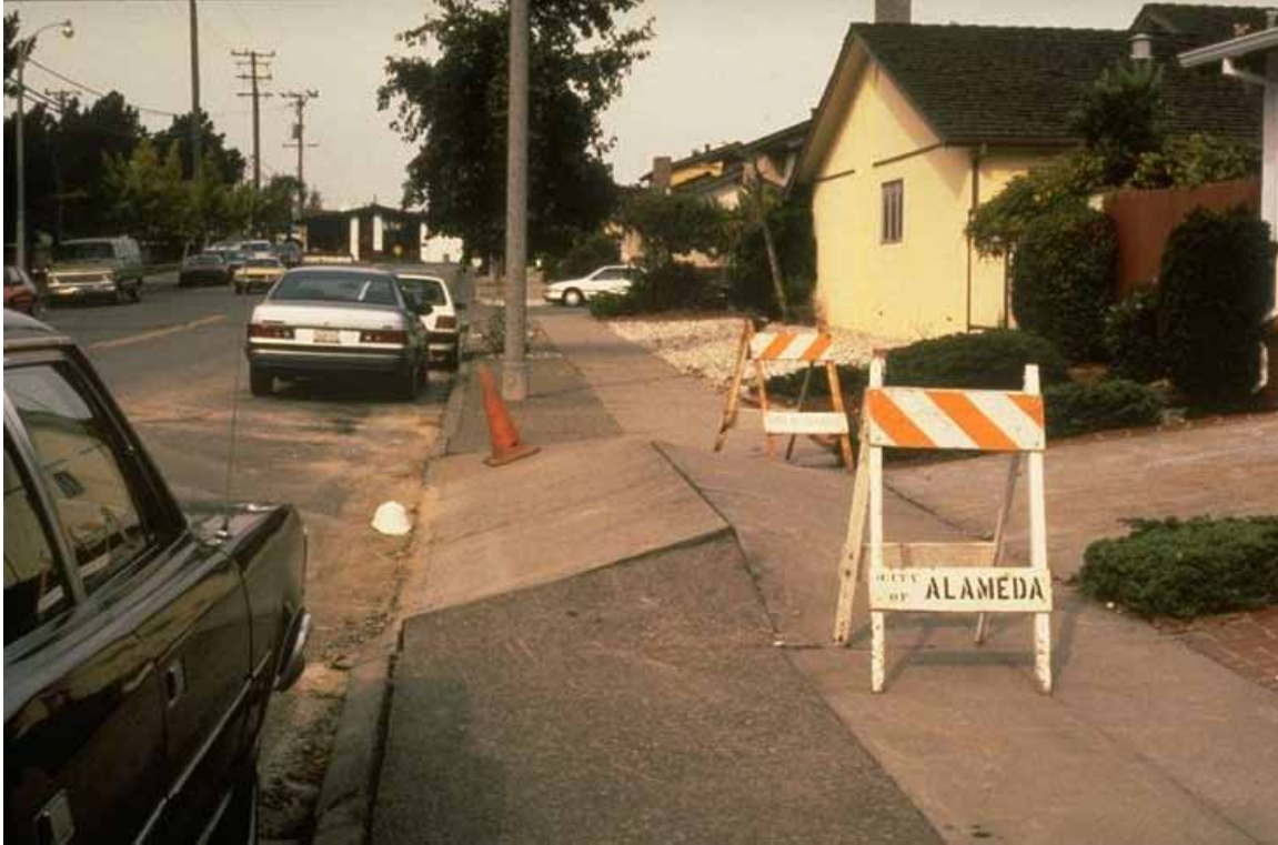
Figure 3.33. Buckling of driveway reportedly due to liquefaction during the 1989 Loma Prieta Earthquake [NISEE].
