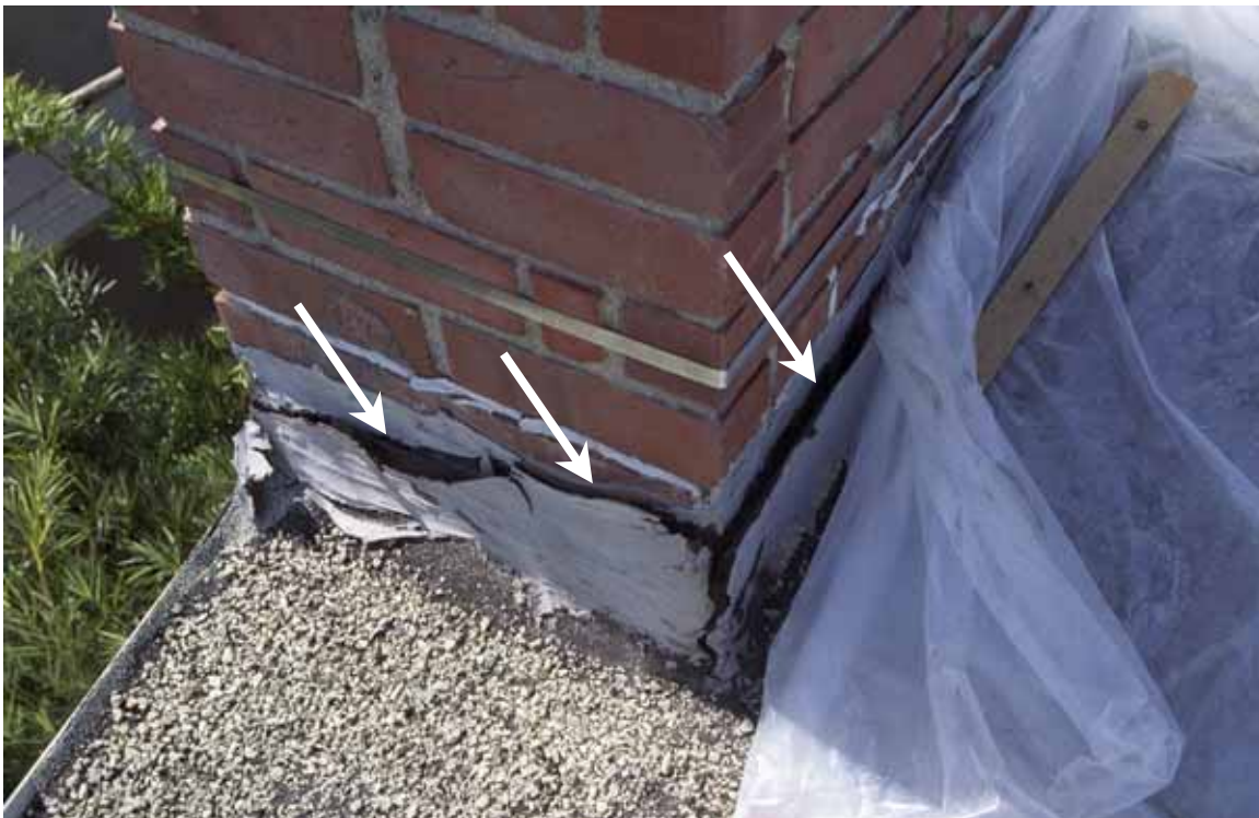
Figure 7.27. Tearing of flashing between chimney and roof caused by relative movement between chimney and building during 1994 Northridge Earthquake [Exponent].
