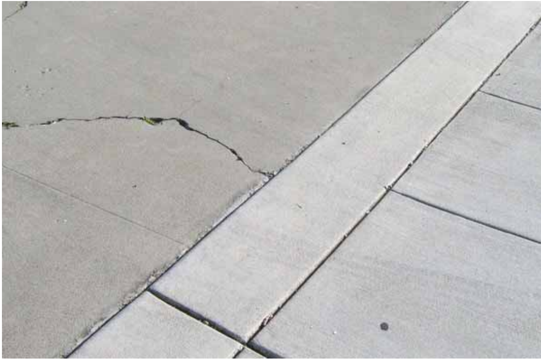
Figure 4.37. Termination of crack in older concrete (upper left) where it abuts newer concrete (lower right) indicates that crack existed prior to the installation of the newer concrete [Exponent].
