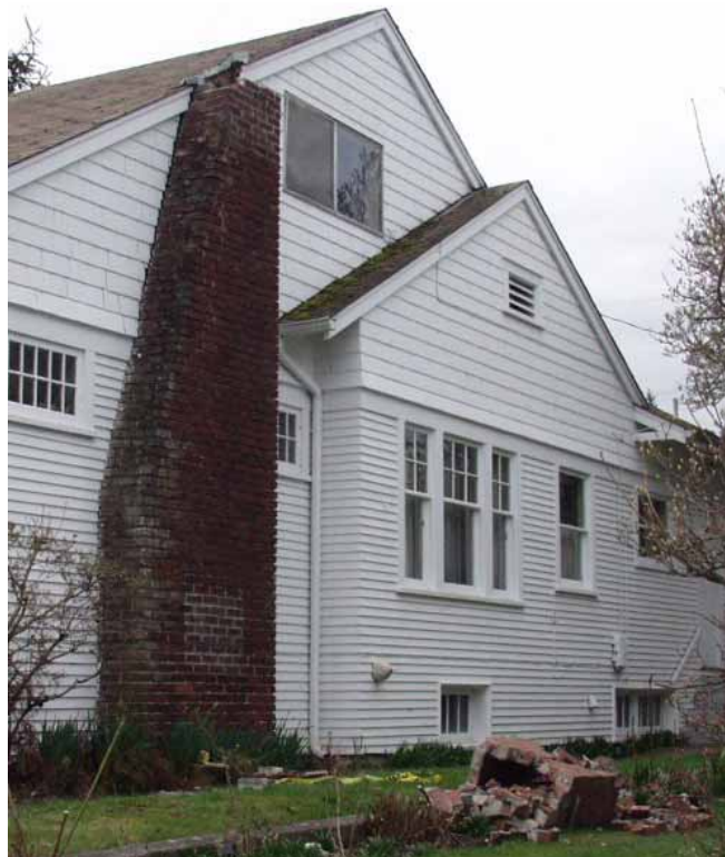
Figure 7.18. Failure of masonry chimney at roofline caused by the 2001 Nisqually Earthquake [Exponent].
