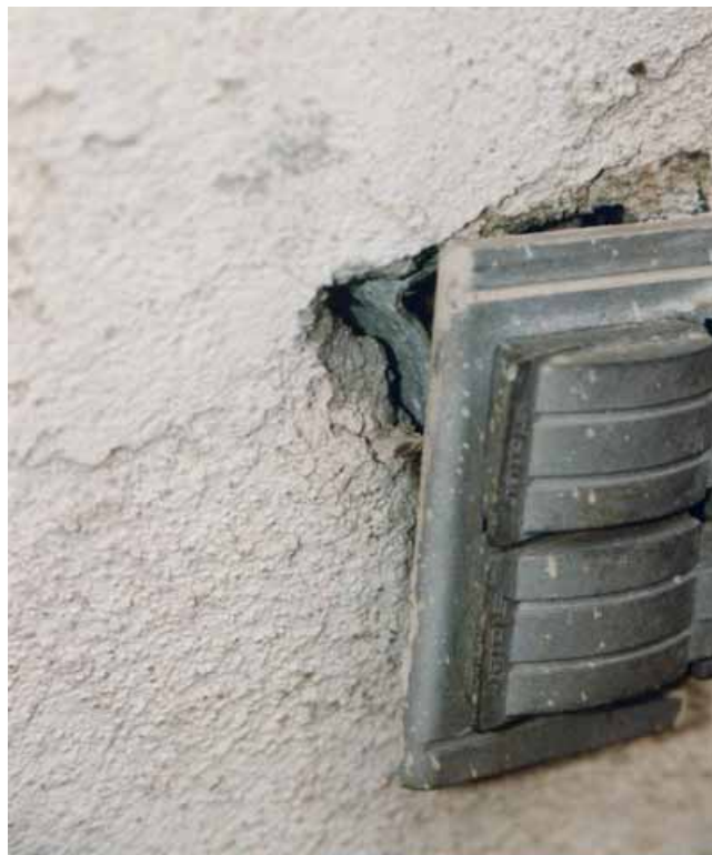
Figure 8.9. Close-up of earthquake damage to electrical outlet box [Exponent].
