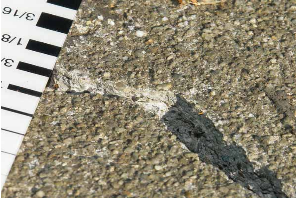
Figure 4.23. Fresh crack in concrete exhibiting lighter color on crack face relative to weathered surface [Exponent].
