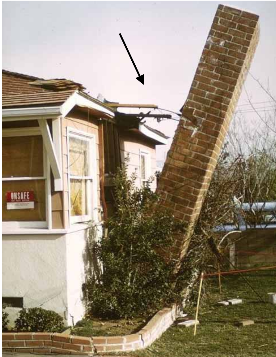
Figure 7.24. Masonry chimney and fireplace that has tilted away from the structure, and torn loose woodframing to which steel tie straps from the chimney were attached – caused by the 1971 San Fernando Earthquake [Cluff].
