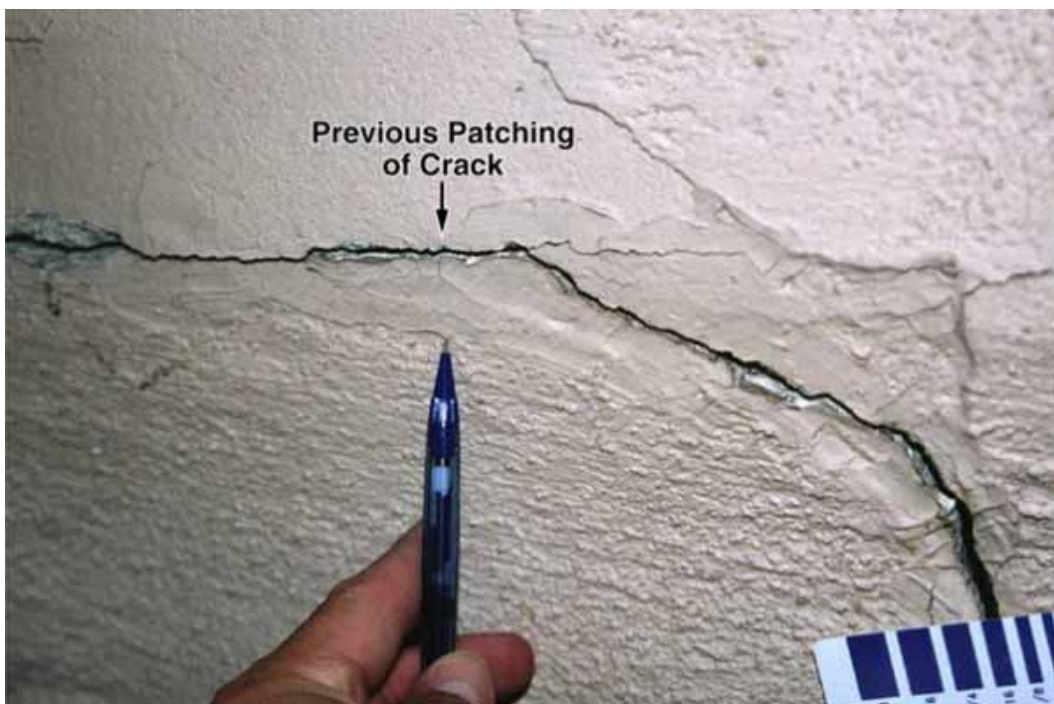
Figure 4.28. Older crack in foundation stem wall exhibiting prior patching and painting [Exponent].
