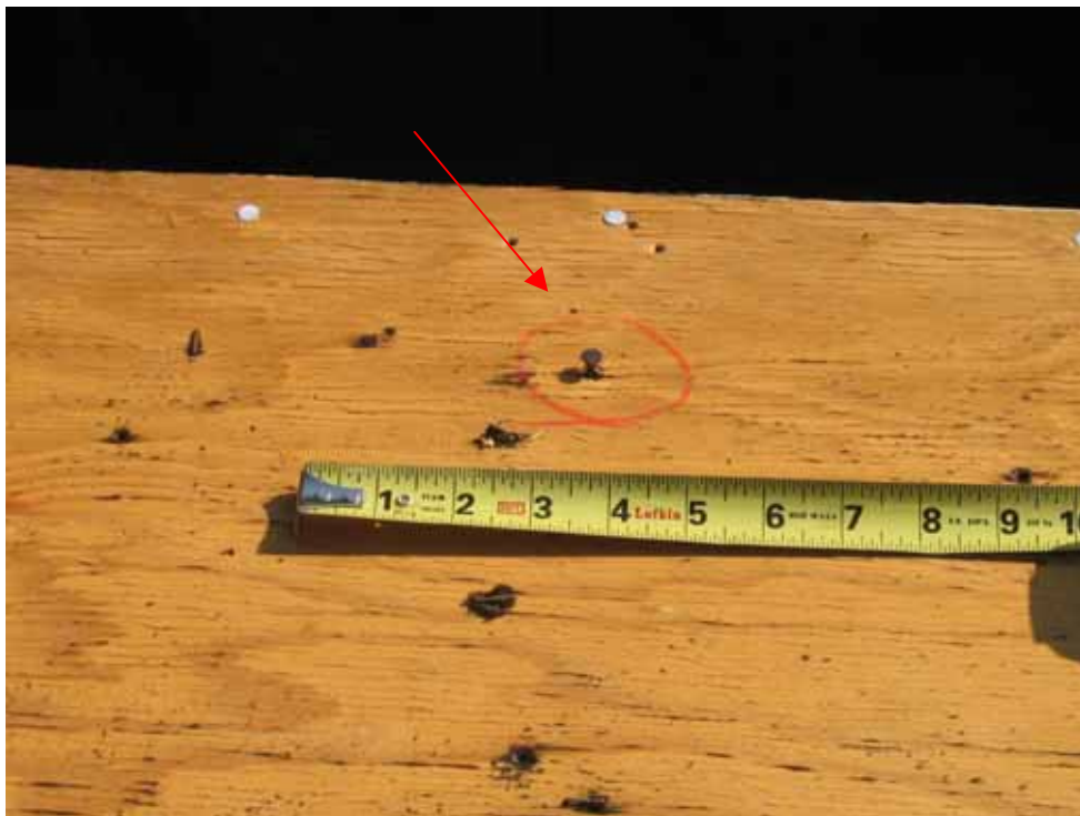
Figure 6.5. Nail withdrawal from plywood roof sheathing due to long-term moisture cycling (not earthquake damage) [Exponent].
