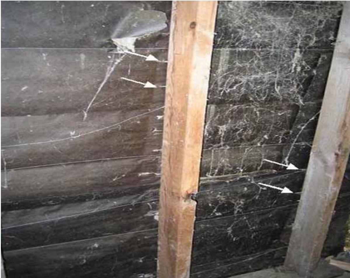
Figure 5.22. Earthquake-induced racking and delamination of stucco as viewed from backside (garage) [Exponent].
