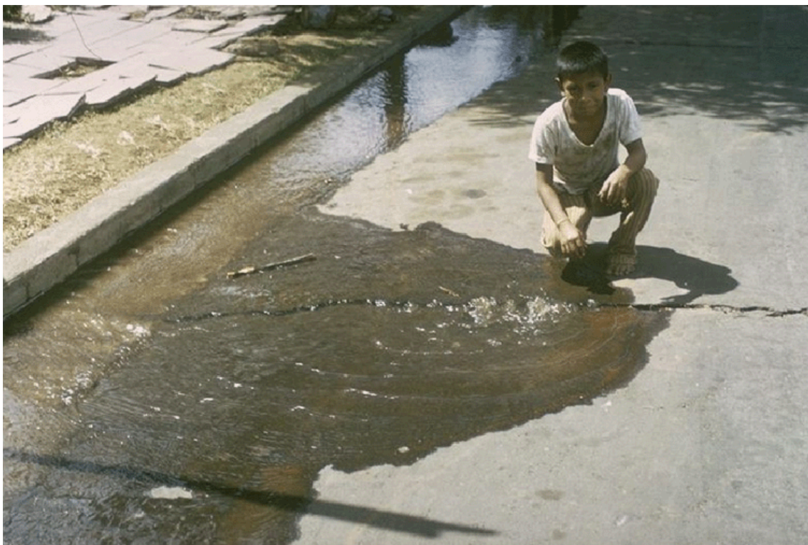
Figure 3.10. Waterline break along fault rupture from the 1972 Managua, Nicaragua Earthquake [NISEE].
