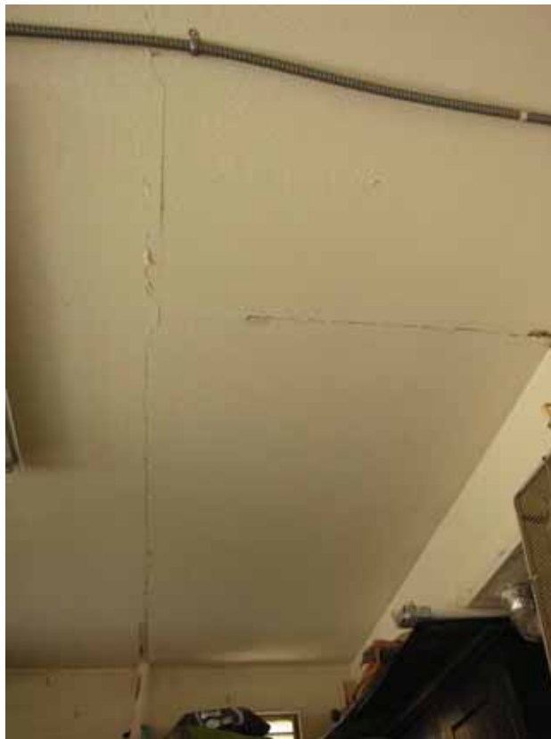
Figure 6.23. Earthquake damage to tape joints at vertical load path discontinuity [Exponent].
