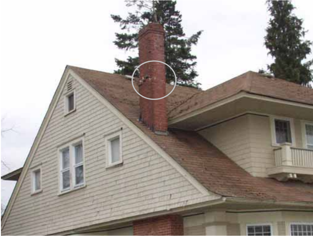
Figure 7.17. Failure of masonry chimney above roofline caused by the 2001 Nisqually Earthquake [Exponent].
