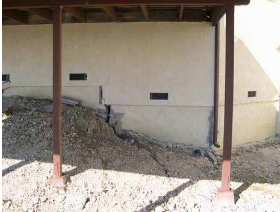
Figure 3.48. Foundation and ground cracking following the 2003 San Simeon Earthquake [Exponent].
