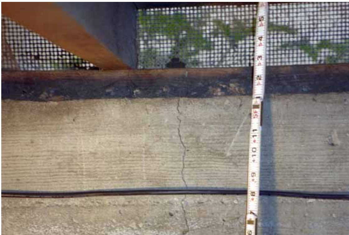
Figure 4.10. Shrinkage crack in a concrete stem wall emanating from an anchor bolt [Exponent].
