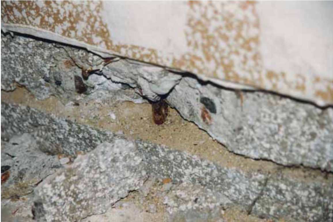
Figure 4.15. Earthquake-induced relative movement at slab/footing interface in two-pour slab-on-grade construction due to sand covering the footing during construction [Exponent].
