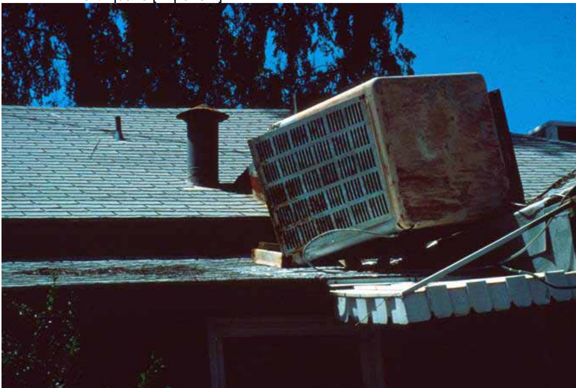
Figure 8.5. Toppled “swamp cooler” due to earthquake [Exponent].
