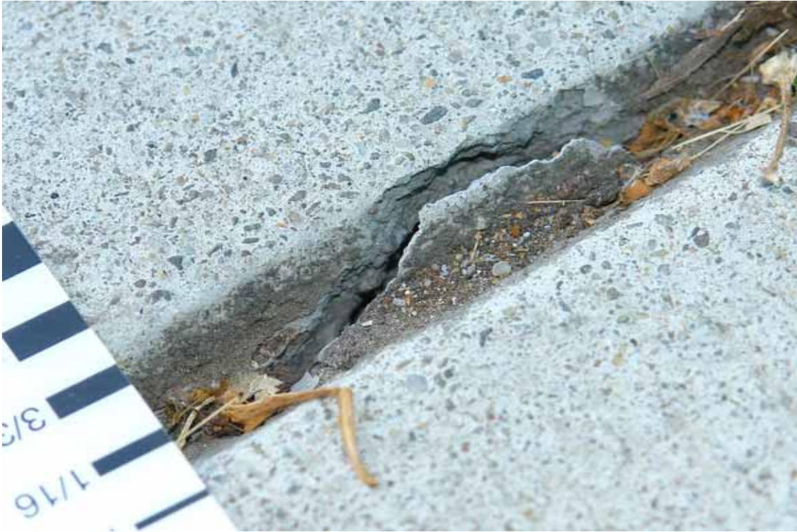
Figure 4.21. Fresh crack in concrete exhibiting sharp edges, crack faces free of contamination and gap clear of debris [Exponent].
