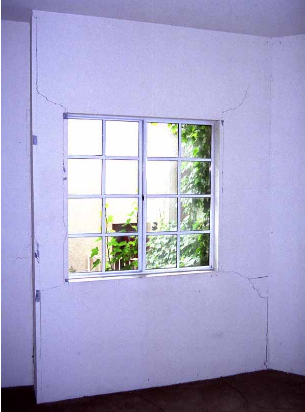
Figure 5.17. Earthquake-induced cracking of drywall as a result of strong shaking [Exponent].
