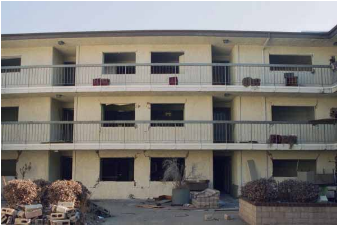
Figure 5.11. Severity of earthquake-induced cracking of wall finishes of multi-story buildings generally decreases at upper stories [Exponent].
