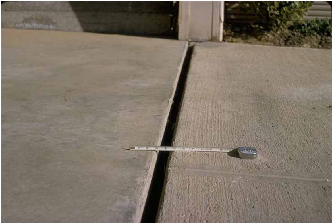
Figure 3.37. A 2-inch separation opened at the construction joint between the garage slab and driveway slab following the 1957 Daly City Earthquake [NISEE].
