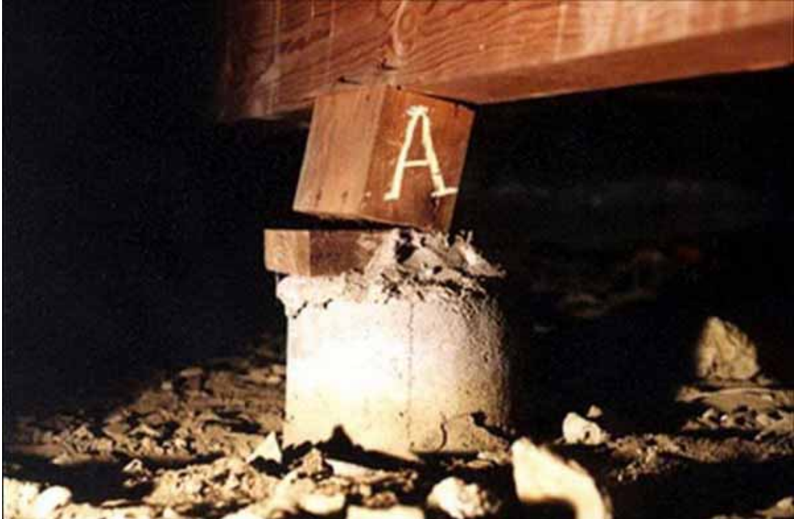
Figure 6.9. Tilted support posts in crawlspace (not earthquake damage) [Exponent].
