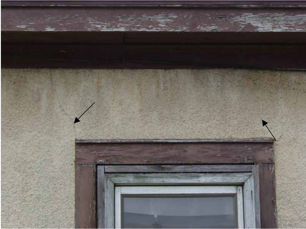
Figure 5.5. Diagonal shrinkage cracks extending from the corners of a wall opening in stucco (not earthquake damage) [Exponent].
