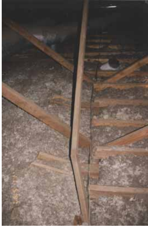
Figure 6.20. Diagonal ridge brace buckled due to earthquake; this brace is in line with the brace shown in Figure 6.21 [Exponent].
