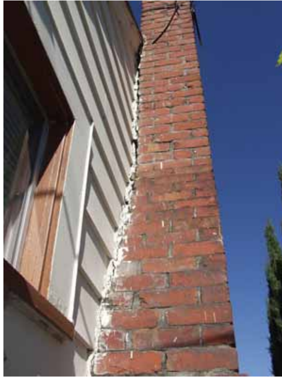
Figure 7.13. Tapered gap between chimney and house that has resulted from long-term differential settlement of fireplace foundation; note mortar filler used to fill previous gap (not earthquake damage) [Exponent].
