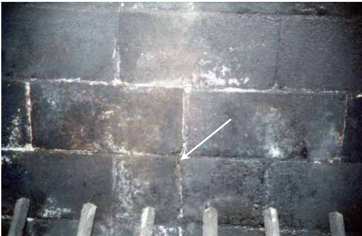
Figure 7.10. Typical thermal cracking of firebrick and mortar lining hearth and firebox of a masonry fireplace (not earthquake damage) [Exponent].
