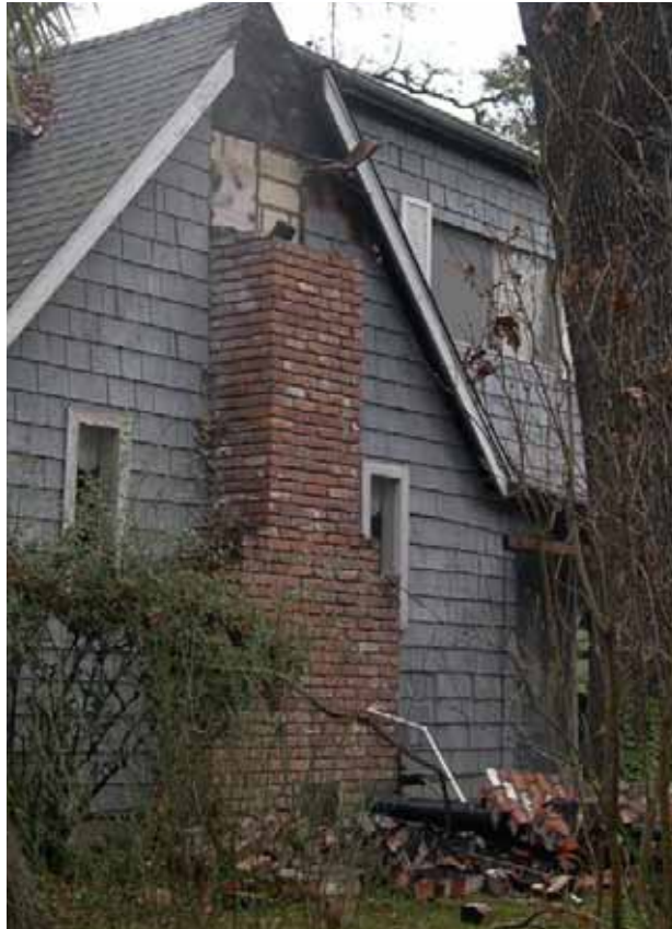
Figure 7.20. Failure of masonry chimney at gable caused by the 2001 Nisqually Earthquake [Exponent].
