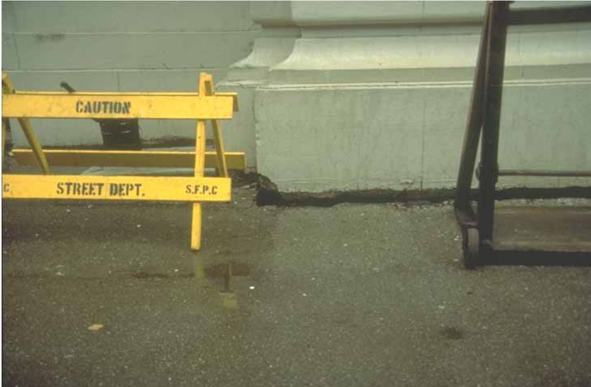
Figure 3.19. Minor settlement caused by densification of loose sandy fill at Embarcadero, Pier 1 in San Francisco during the 1989 Loma Prieta Earthquake; the building is pile-supported [NISEE].
