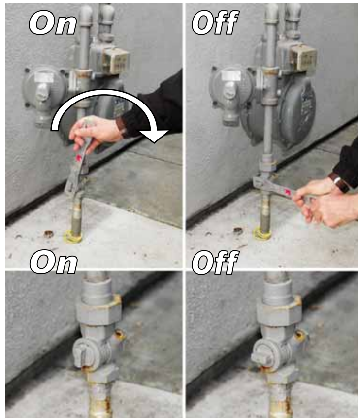
Figure 8.2. Manual gas shut-off valve [Exponent].
