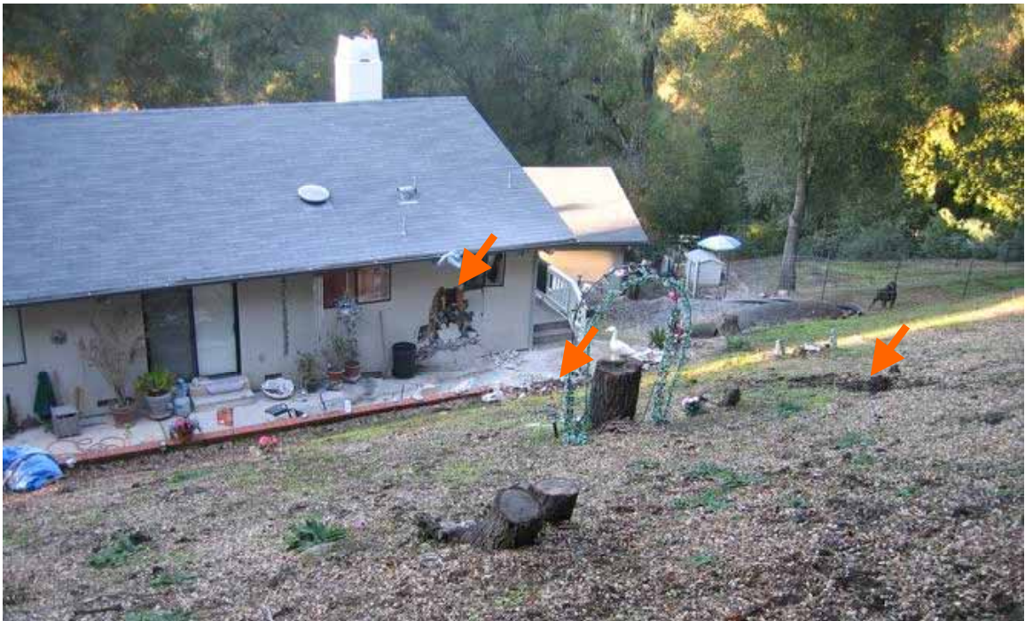
Figure 3.22. Rockfall from 2003 San Simeon Earthquake (top); similar rockfall occurred downslope and impacted house; impact marks on slope and house indicated by arrows (bottom) [Exponent].
