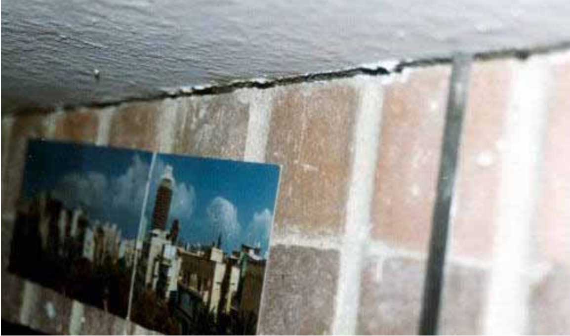
Figure 7.30. Masonry mantle which separated slightly from the wall finish during the 1994 Northridge Earthquake [Exponent].
