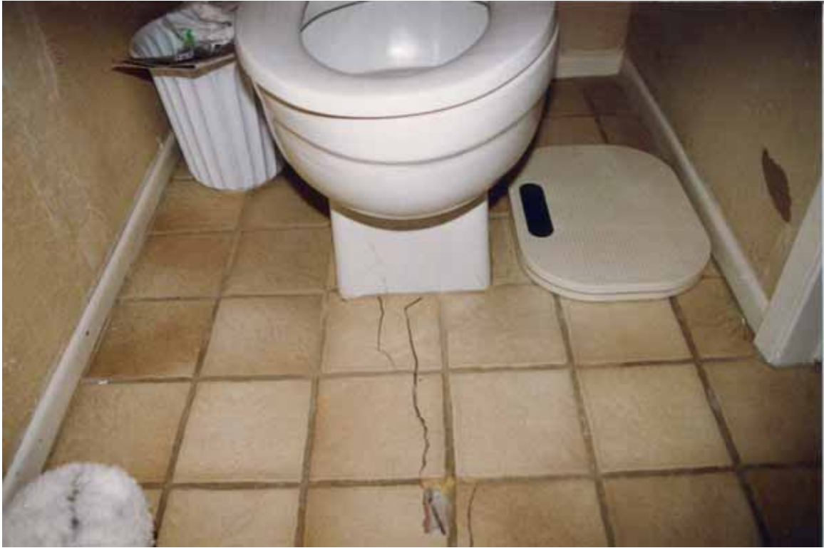
Figure 4.19. Earthquake-induced cracking of ceramic tile on a slab-on-grade [Exponent].
