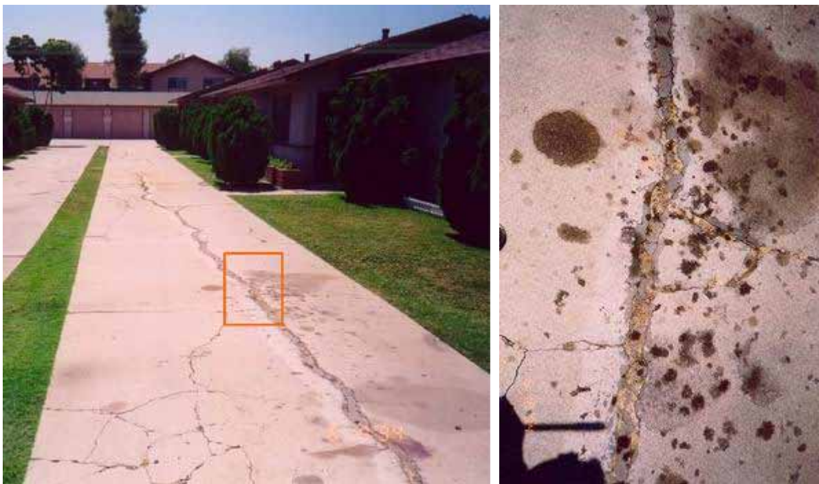
Figure 3.41. Grout within driveway slab-on-grade crack indicates long-term problem with expansive soil beneath driveway rather than earthquake damage [Exponent].
