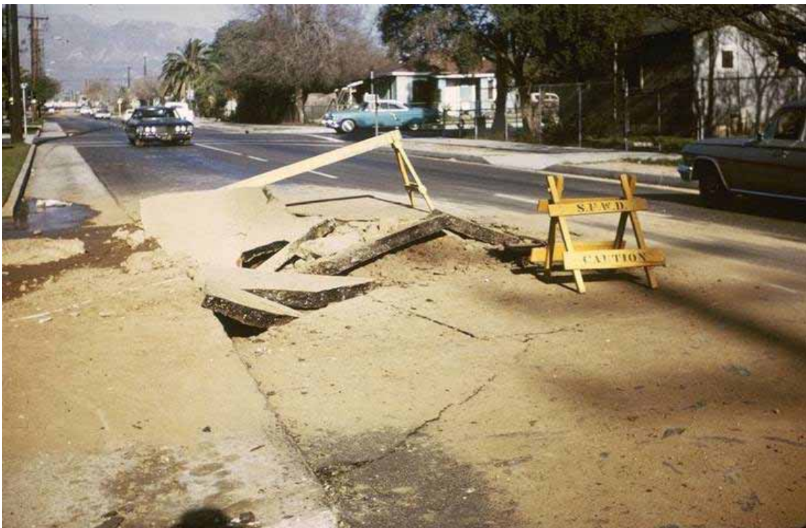
Figure 3.43. Pipe failures and resulting pavement distress and settlement from the 1971 San Fernando Earthquake [NISEE].
