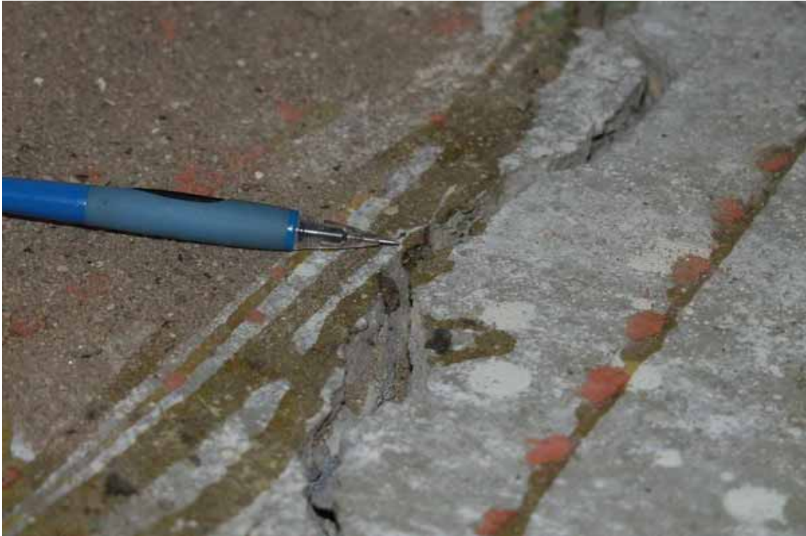
Figure 4.25. Older crack in concrete floor slab contaminated with carpet pad adhesive [Exponent].
