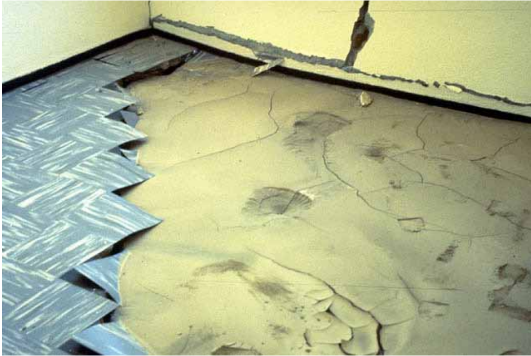
Figure 3.50. Damaged concrete slab-on-grade floor of the house shown in Figure 3.49; sandy mud ejected by liquefaction covers part of the floor [NISEE].
