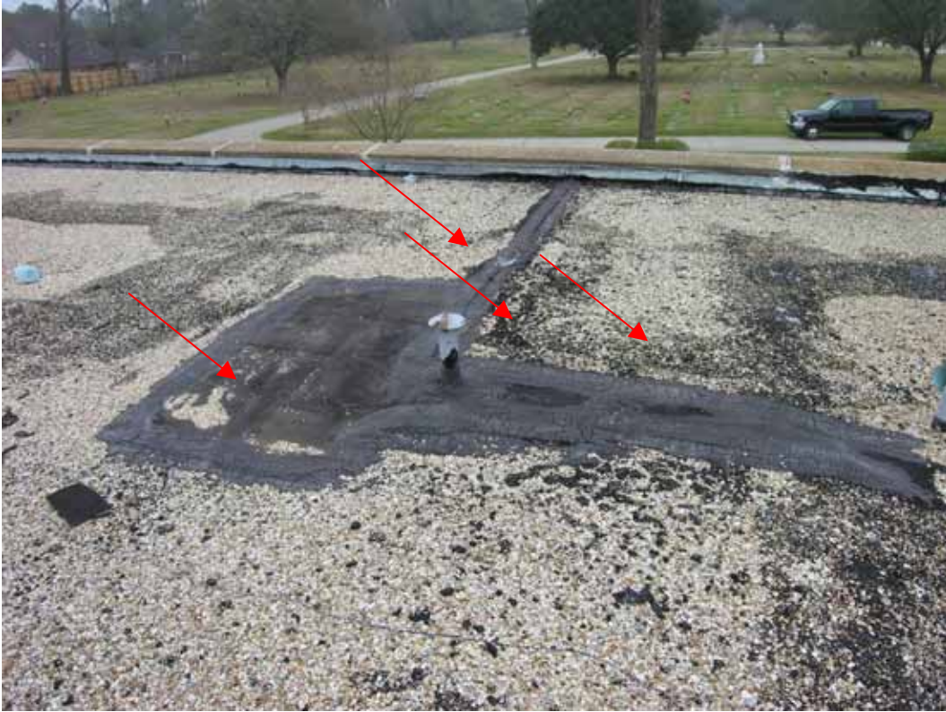
Figure 6.6. Deteriorated mastic at repair of built-up roof (not earthquake damage) [Exponent].
