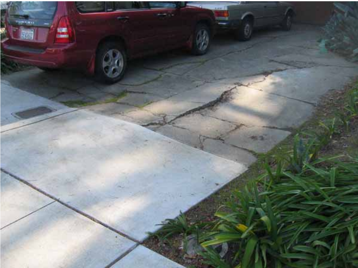
Figure 4.14. Cracking due to vehicle loads on a concrete driveway over soft soil [Exponent].
