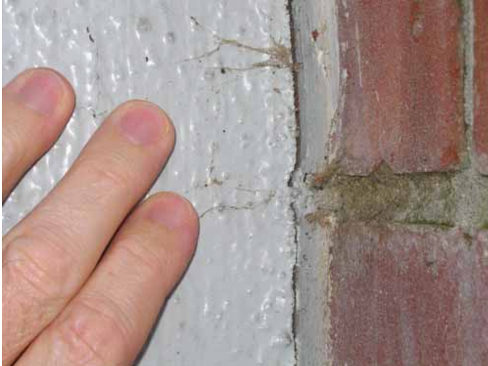
Figure 7.11. Normal crack between masonry fireplace/chimney and exterior stucco wall (not earthquake damage) [Exponent].
