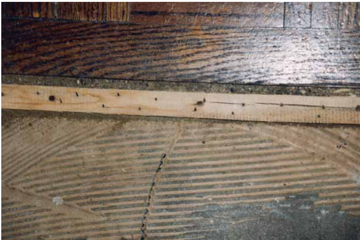
Figure 4.26. Parquet flooring adhesive filling crack in concrete slab [Exponent].
