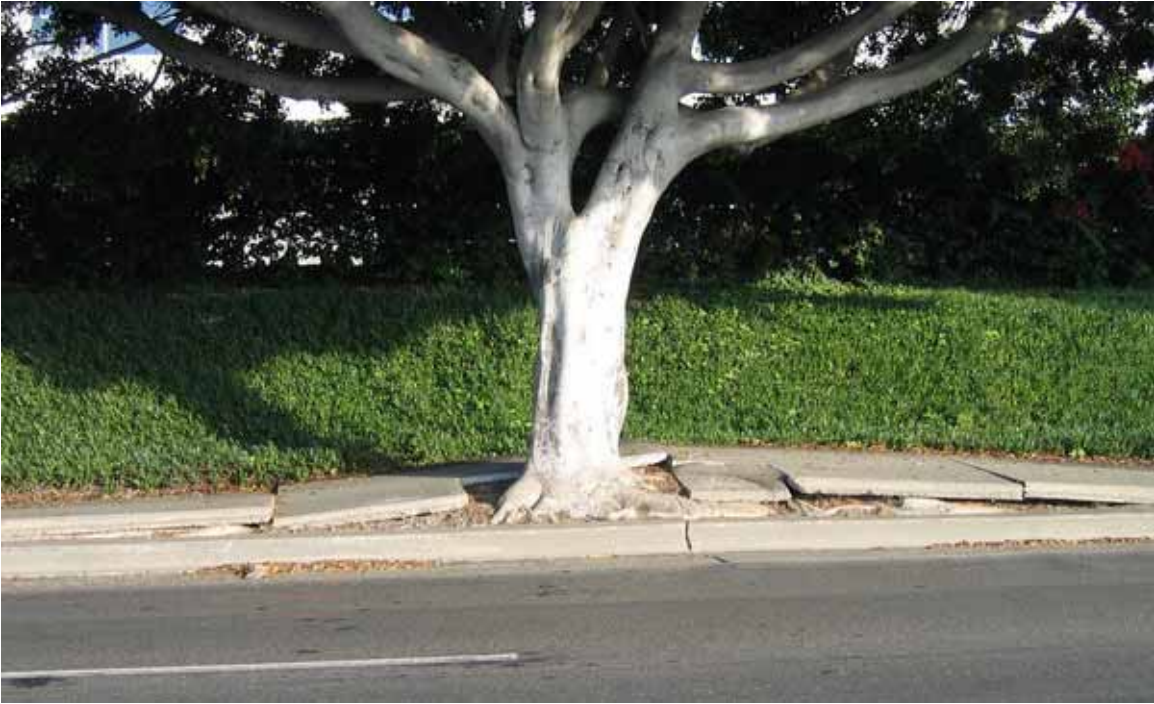
Figure 4.13. Uplift and cracking of concrete sidewalk caused by tree roots [Exponent].
