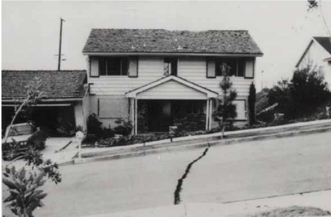
Figure 3.29. Street and house damaged by several inches of landslide displacement during the 1971 San Fernando Earthquake; displacement is readily visible as street crack in photograph [ATC, Youd].
