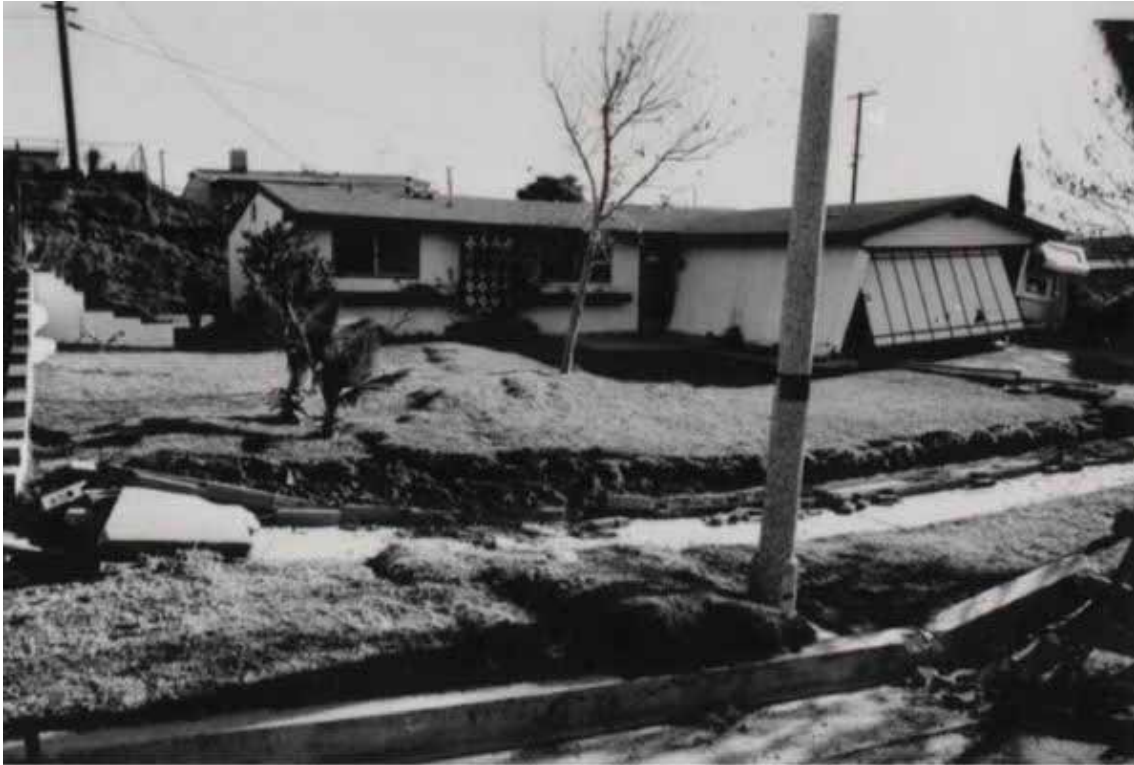
Figure 3.9. House damaged by surface fault rupture from the 1971 San Fernando Earthquake [ATC, Castle].
