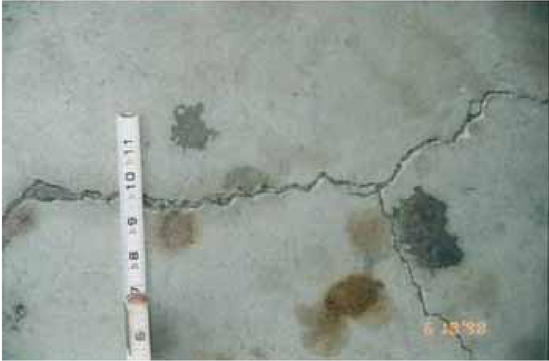
Figure 4.29. Mortar within garage slab-on-grade crack indicates previous patching of crack (not earthquake damage) [Exponent].
