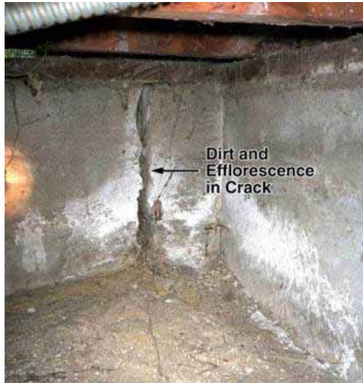
Figure 4.33. Dirt and efflorescence indicates age of foundation wall crack is not recent (not earthquake damage) [Exponent].
