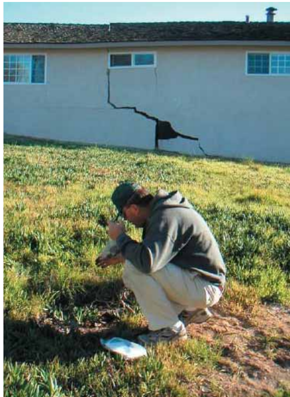
Figure 3.51. Damage to a residence in Oceano, California from lateral spreading following the 2003 San Simeon Earthquake [USGS].
