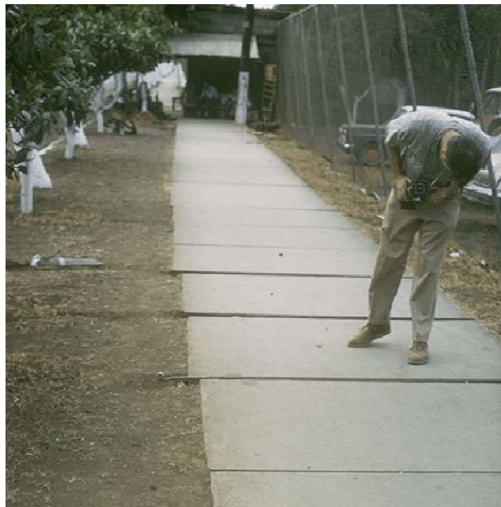
Figure 3.12. Sidewalk displaced by distributed faulting from the 1972 Managua, Nicaragua Earthquake [NISEE].
