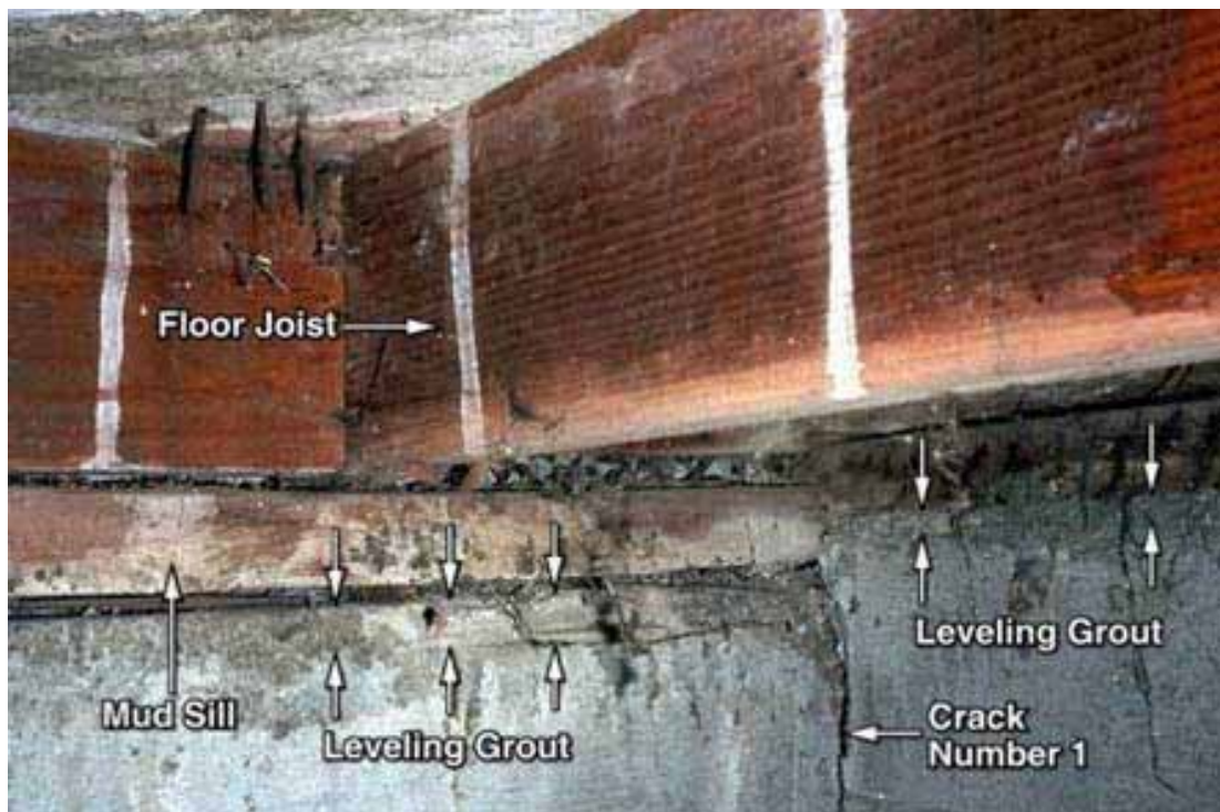
Figure 3.53. Releveling of foundation indicates prior settlement and possibly on-going deformation mode rather than earthquake damage [Exponent].
