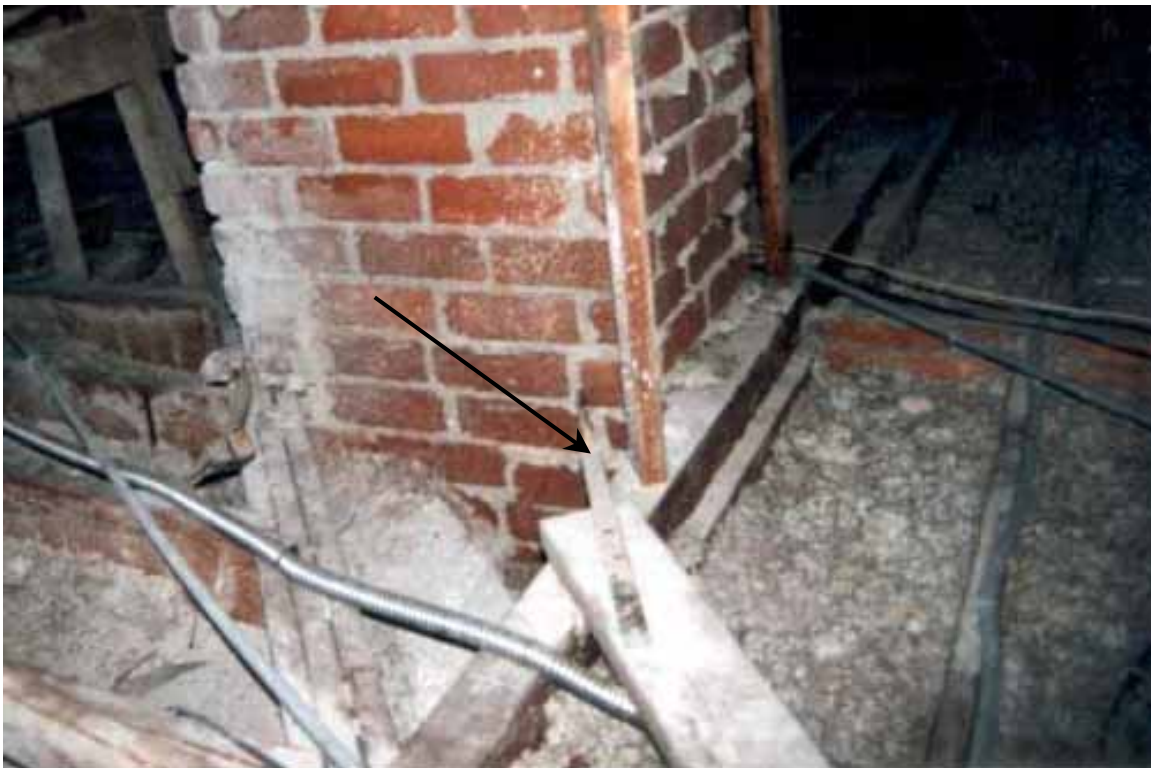
Figure 7.4. Chimney visible in attic – note undamaged steel tie strap between chimney and framing [Exponent].
