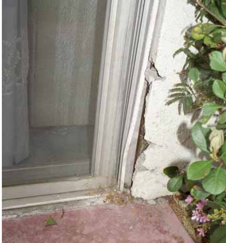
Figure 5.15. Earthquake-induced delamination of stucco from woodframing and associated damage to aluminum door frame [Exponent].
