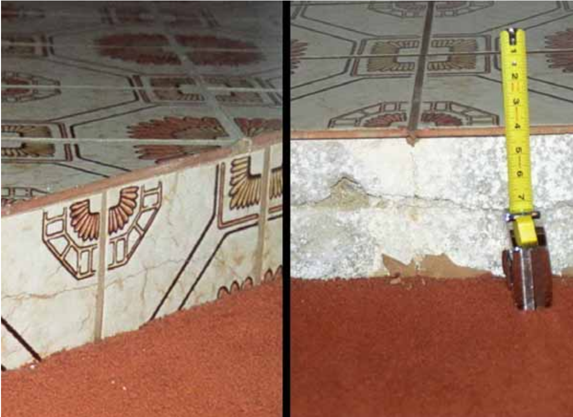
Figure 4.17. Earthquake-induced cracking of ceramic tile spanning the cold joint between the floor slab and the stem wall in a two-pour system [Exponent].
