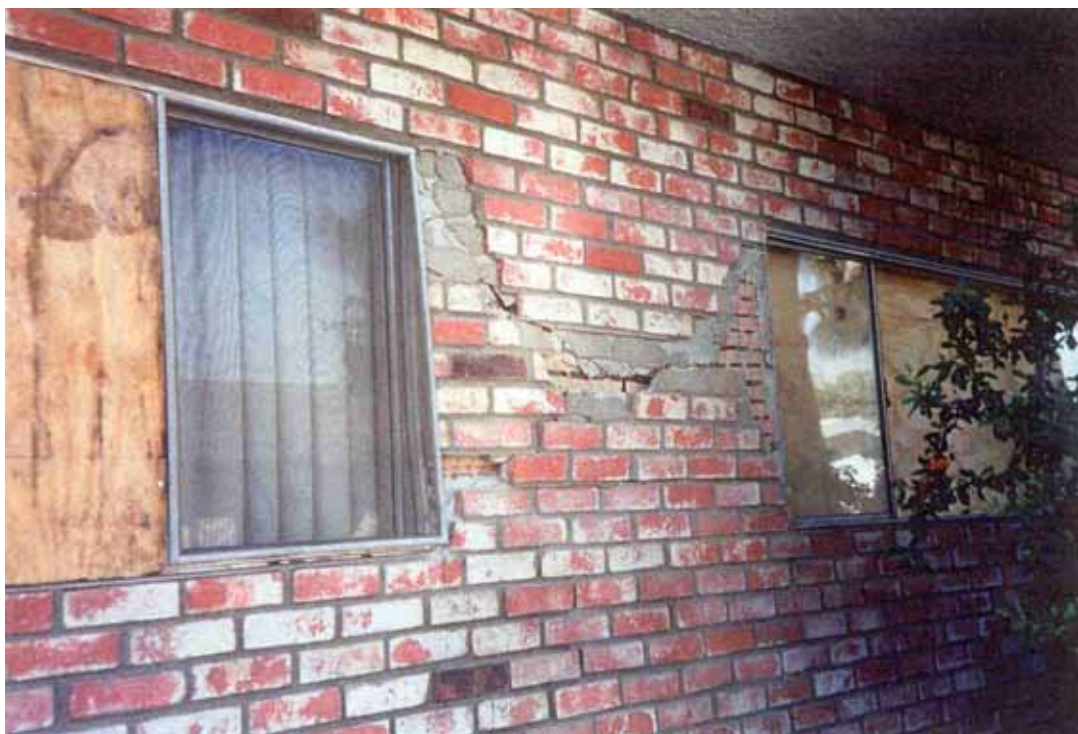
Figure 5.13. Earthquake-induced “X” cracking in stucco panels between windows (thin brick veneer had been installed over stucco).
