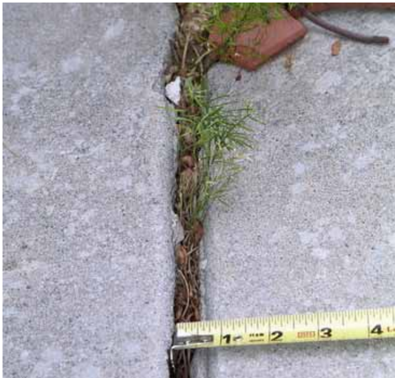
Figure 4.34. Debris and vegetation in older crack (not earthquake damage) [Exponent].
