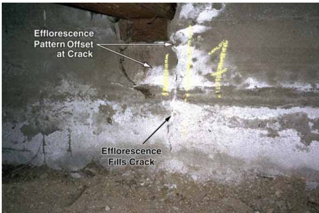
Figure 4.38. Pattern of efflorescence around crack in stem wall indicates that crack is not of recent origin [Exponent].
