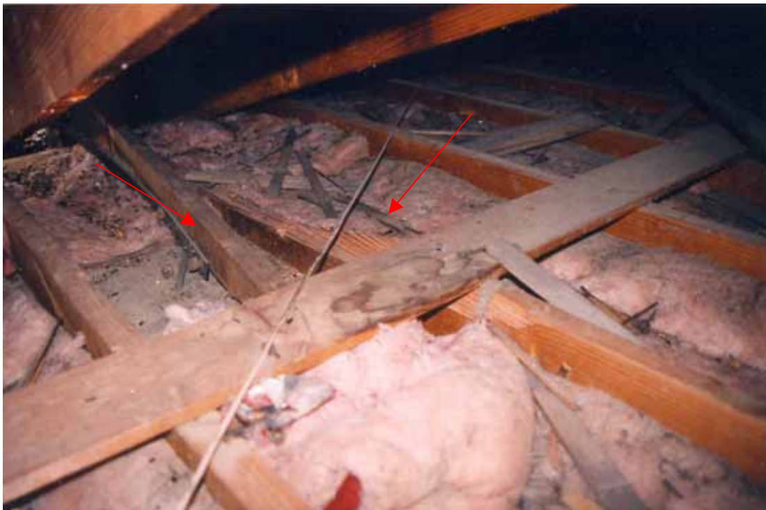
Figure 6.19. Earthquake-induced framing damage due to loads from chimney strap; note the strap was attached to the top of a ceiling joist (left arrow), which split from the bottom (right arrow) when the chimney, located just outside rafter ends in top left of photo, moved relative to the house [Exponent].
