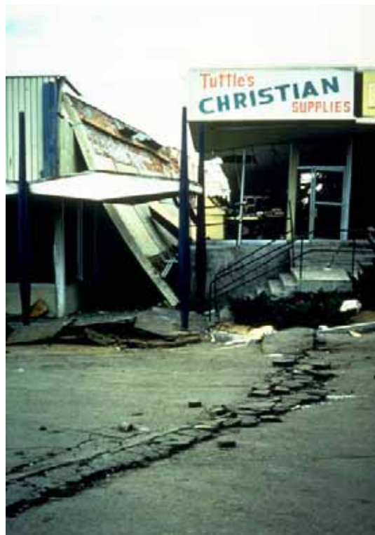
Figure 3.8. Surface fault rupture from the 1971 San Fernando Earthquake and associated damage to pavement and buildings in the Sylmar area [NISEE].
