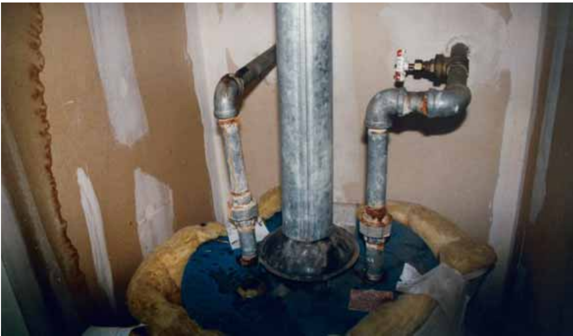
Figure 8.12. Water heater with “hard” piping (no damage) [Exponent].
