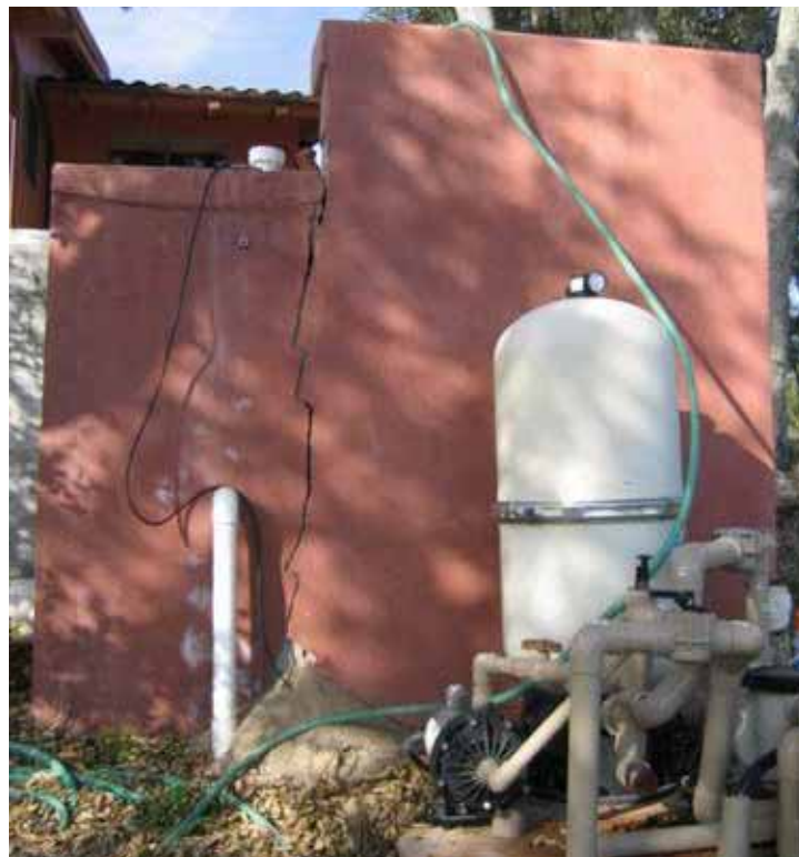
Figure 3.24. Retaining wall damage during the 2003 San Simeon Earthquake; granular backfill spilling from new crack in retaining wall [Exponent].
