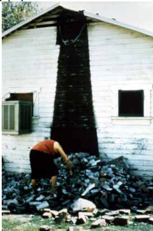
Figure 7.29. Collapsed unreinforced masonry chimney.
