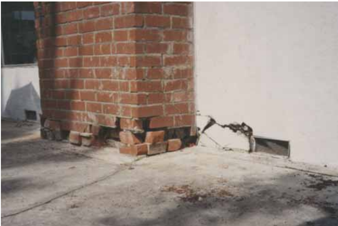
Figure 7.23. Failure of masonry fireplace at foundation level caused by the 1994 Northridge Earthquake [Exponent].
