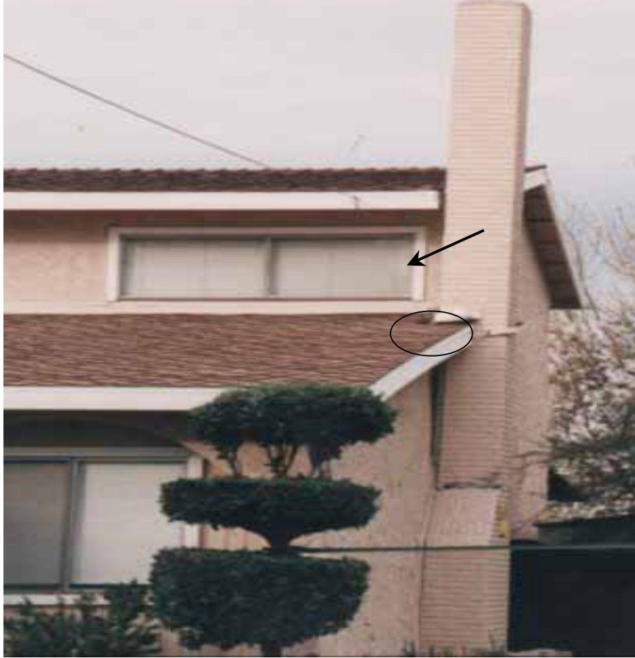
Figure 7.1. Monolithic precast concrete fireplace and chimney that cracked at the shoulder (oval) and pulled away from the building (arrow) due to earthquake.
