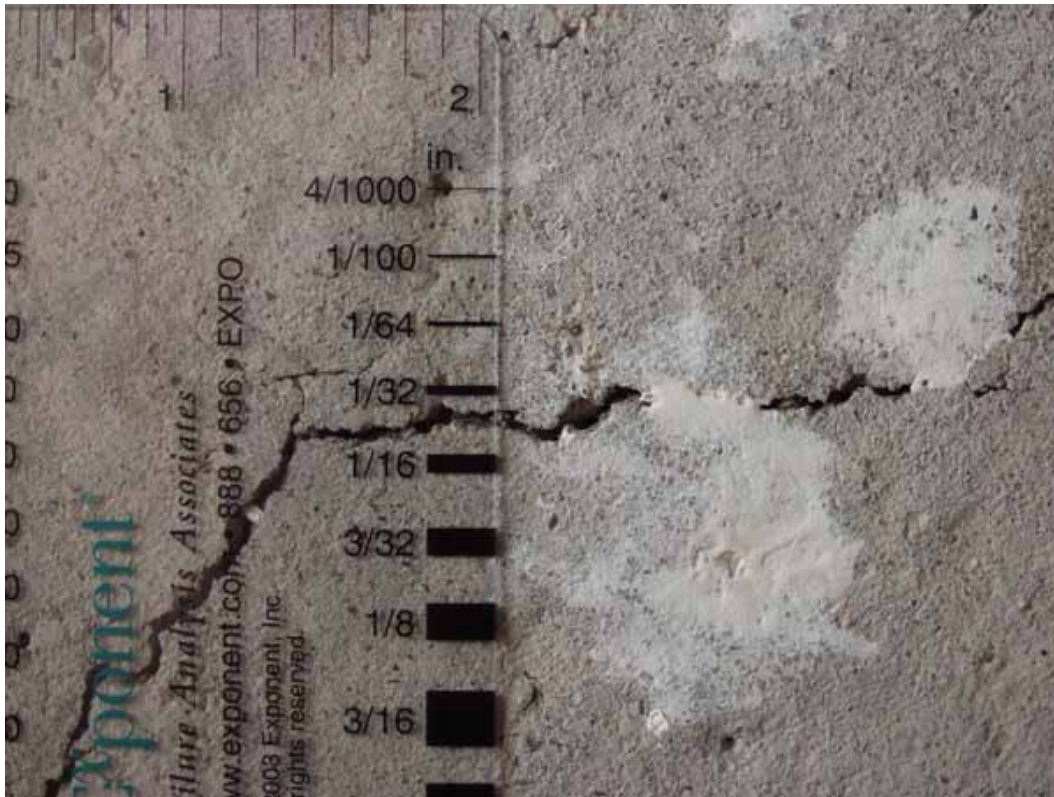
Figure 4.27. Dabs of drywall joint compound within shrinkage crack in concrete slab-on-grade floor [Exponent].
