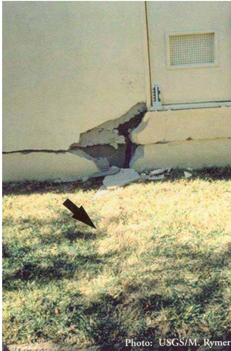
Figure 3.46. Foundation slab and wall of this house in the Balboa Boulevard area was damaged by small settlement and ground cracking that is evident in the lawn (arrow) during the 1994 Northridge Earthquake [USGS].
