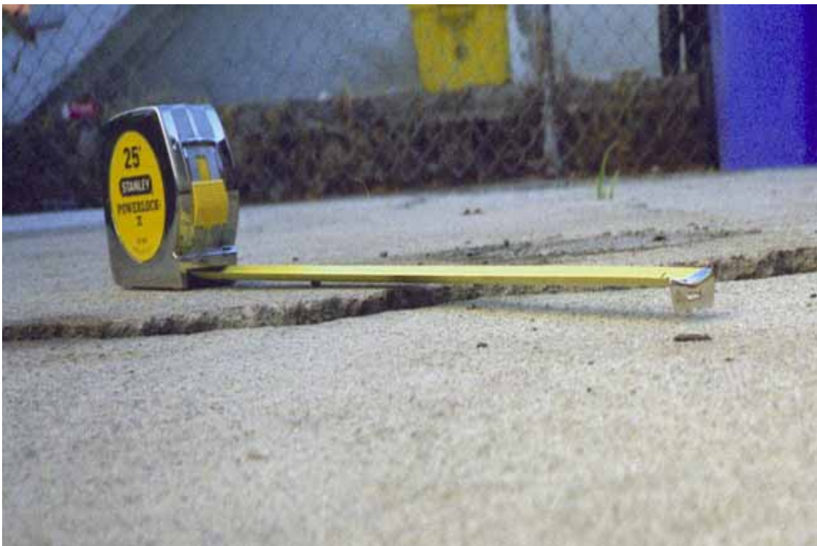
Figure 4.20. Illustration of out-of-plane offset in a concrete slab-on-grade [Exponent].
