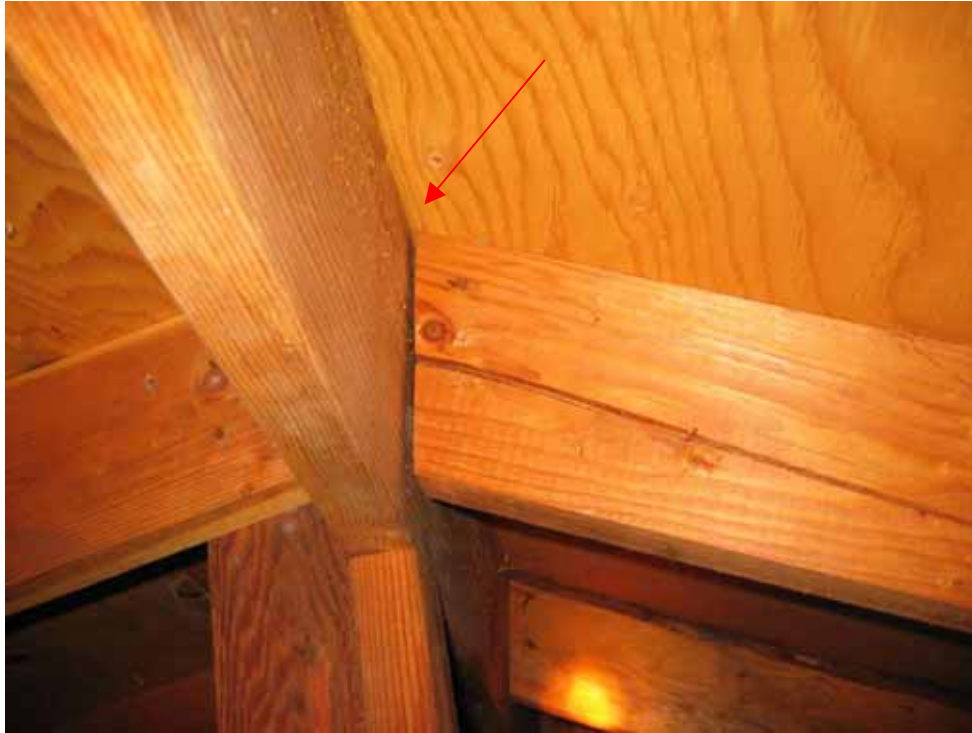
Figure 6.4. Poor fit-up of roof framing at rafter to ridge board junction (not earthquake damage) [Exponent].
