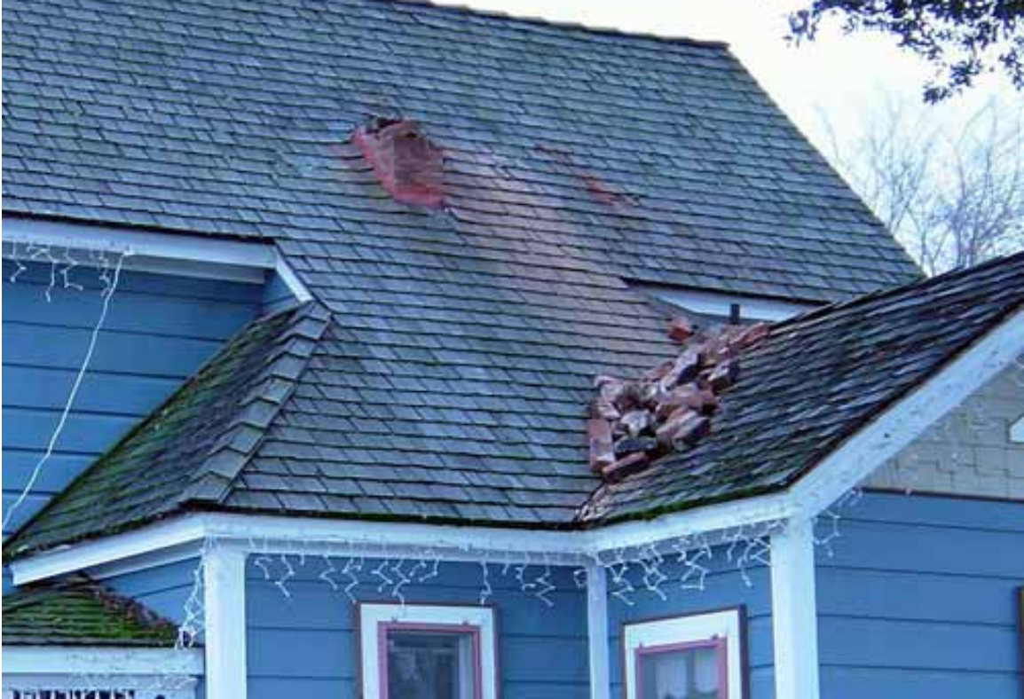
Figure 7.28. Rooftop debris from collapse of masonry chimney during the 2003 San Simion Earthquake [Dyce].
