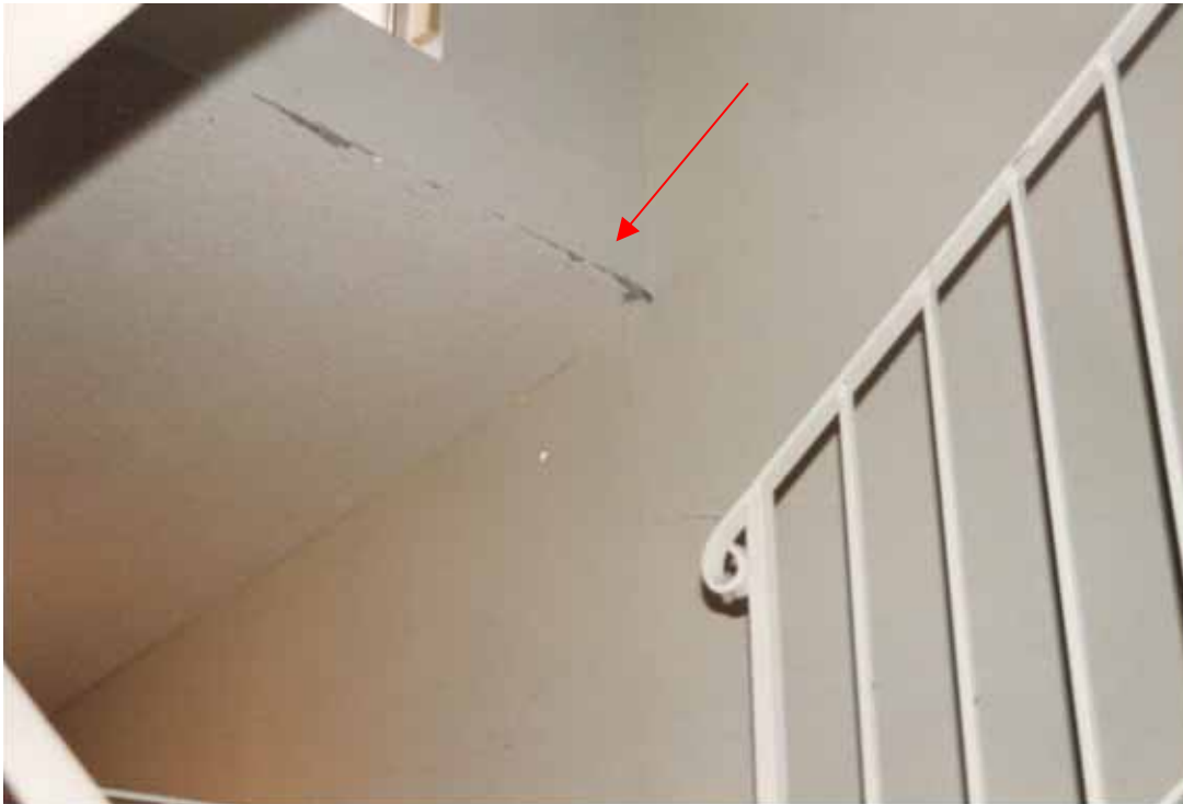
Figure 6.22. Earthquake damage to ceiling corner bead at stairwell [Exponent].
