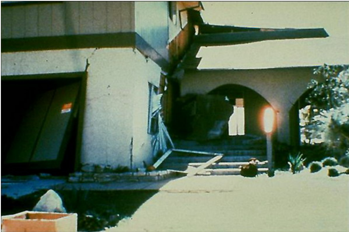
Figure 6.15. Earthquake-induced separation across discontinuous floor and roof diaphragms of a split level house.
