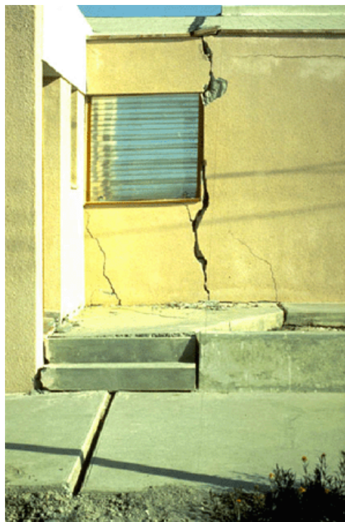
Figure 3.49. One-story masonry house in a main housing development in the town of Caucete, damaged due to differential settlement caused by liquefaction during the 1977 Caucete, San Juan, Argentina Earthquake; damage to the interior slab is shown in Figure 3.50 [NISEE].
