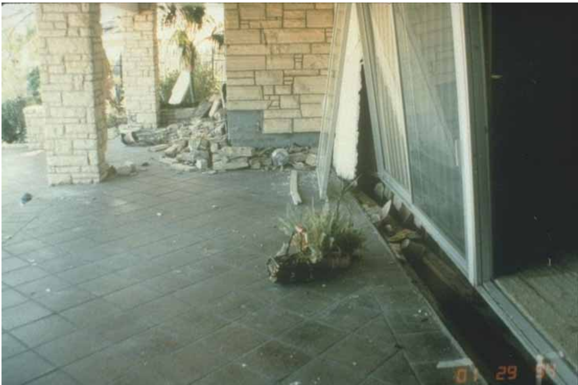
Figure 3.18. Evidence of lateral ground movement, near back of building shown in Figure 3.17 [NISEE].
