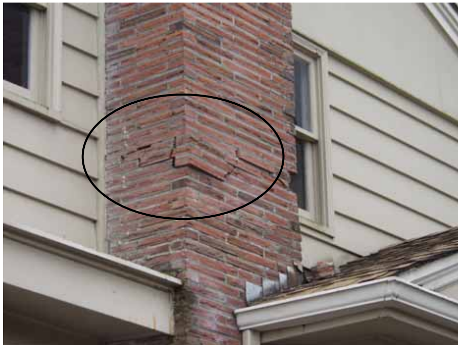
Figure 7.21. Failure of masonry chimney mid-story caused by the 2001 Nisqually Earthquake [Exponent].
