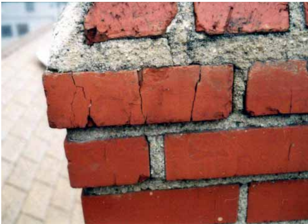
Figure 7.14. Random isolated cracking of brick and mortar joints commonly found on masonry fireplaces and chimneys (not earthquake damage) [Exponent].
