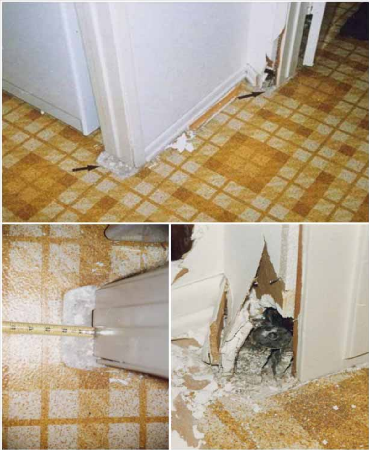
Figure 5.23. Earthquake-induced displacement of an interior partition due to inadequate attachment to floor slab [Exponent].
