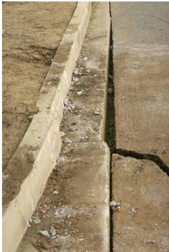
Figure 3.32. Damaged street, gutter, and curb from the 1971 San Fernando Earthquake [NISEE].
