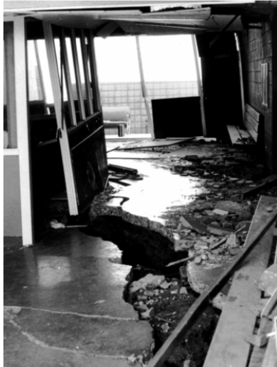
Figure 3.52. Damage to a slab-on-grade from liquefaction at Los Angeles County Juvenile Hall, Sylmar, California during the 1971 San Fernando Earthquake [Meehan].
