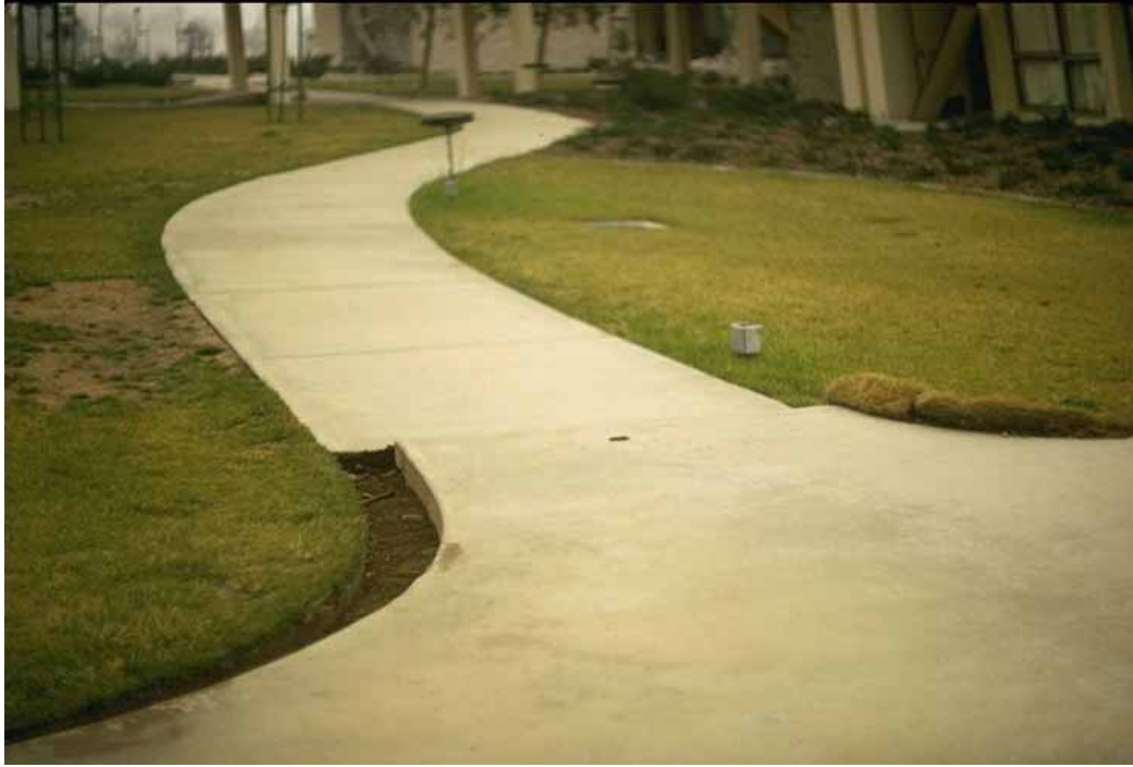
Figure 3.31. Offset sidewalk from the 1971 San Fernando Earthquake [NISEE].
