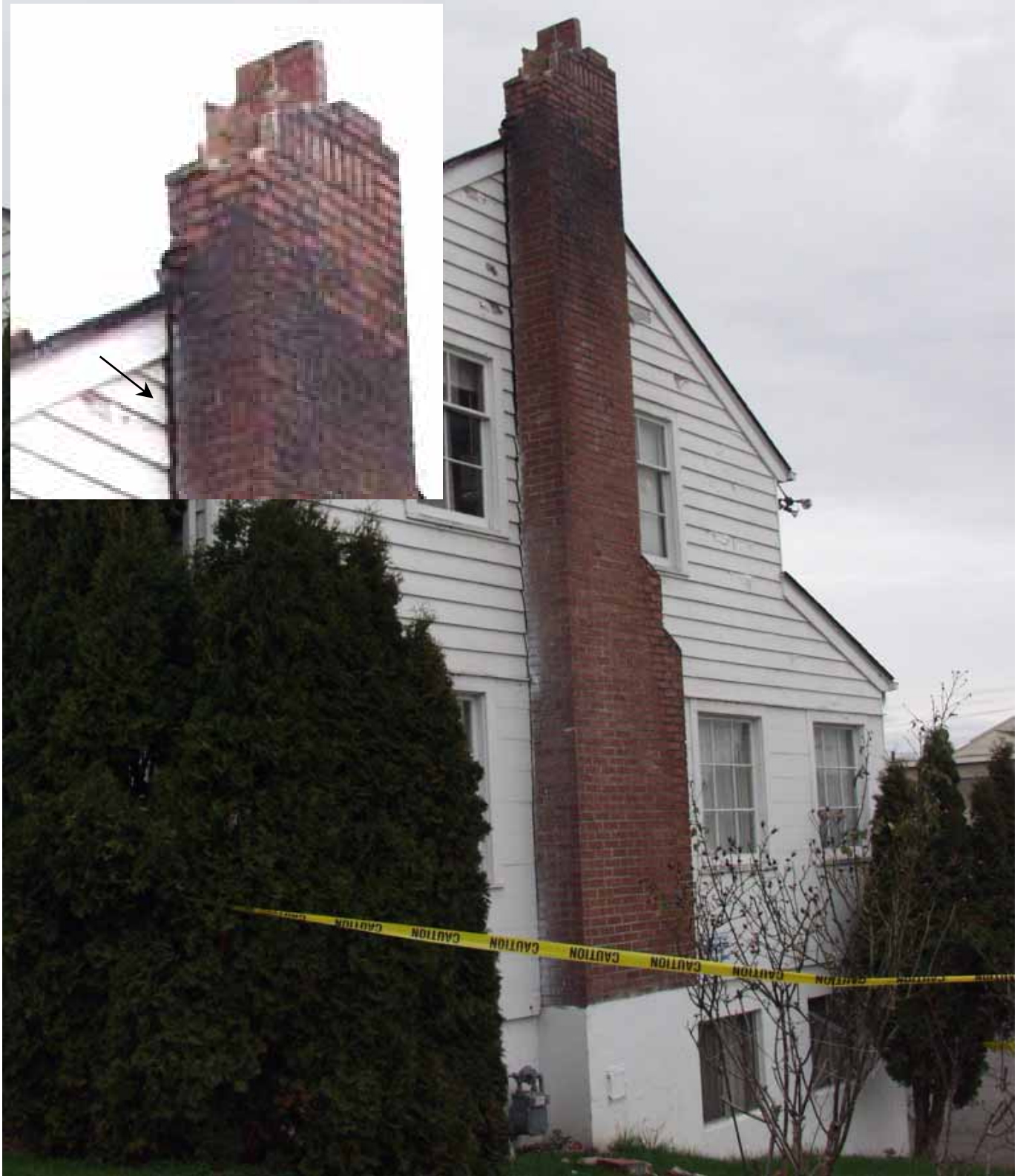
Figure 7.25. Earthquake-induced tapered separation between masonry chimney and exterior wall caused by the 2001 Nisqually Earthquake; note also damage to top of chimney due to deterioration of mortar [Exponent].
