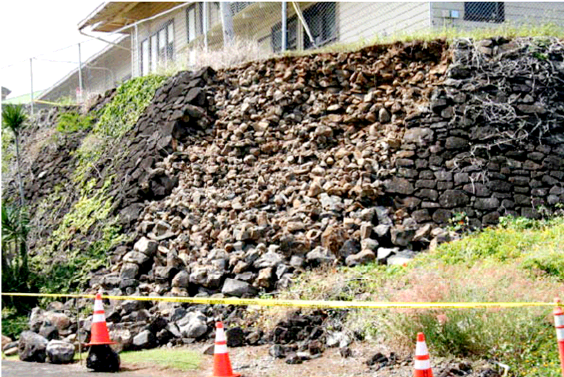
Figure 3.25. Collapse of un-mortared and unreinforced stone retaining wall in Honokaa, Hawaii during the 2006 Hawaii Earthquakes [UHM].
