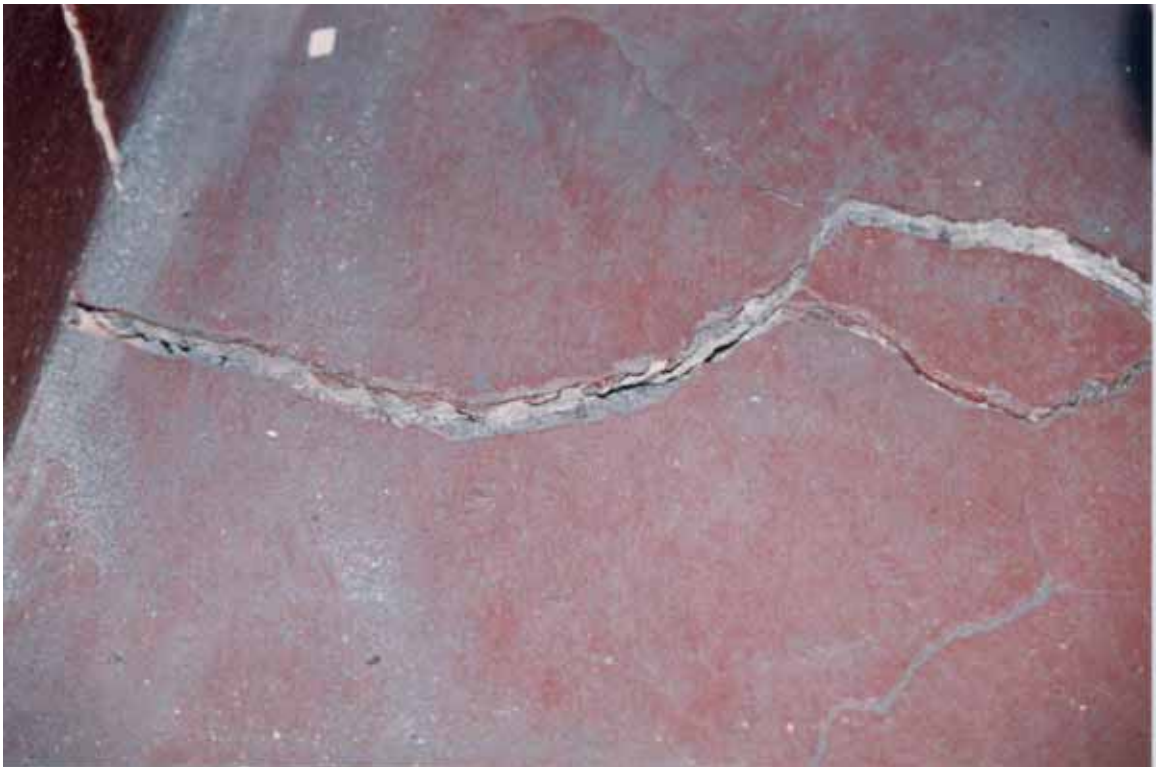
Figure 4.24. Older crack in concrete exhibiting worn and rounded edges contaminated with paint [Exponent].
