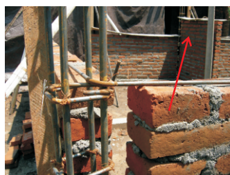
Picture of Connection between wall and column
