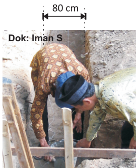
Dig picture for foundation base width of digging is 80 cm
