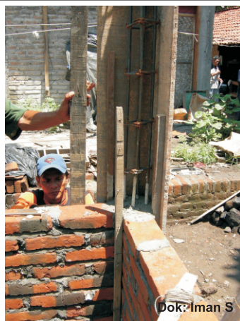
Concreting doing partly every 1 m
