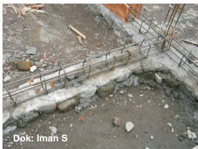
Picture of connection between column and tie beam/ sloof
