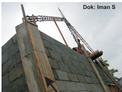
Make sure that form work is hard/ rigid and no bleeding
