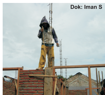
Compaction using wood, bamboo, or reinforcing bar stick
