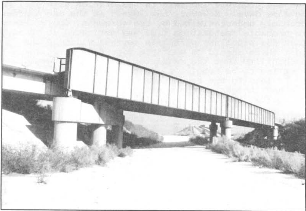
Figure 10 A Railroad Bridge Estimated to Collapse Onto Highway 138 (Highway 138 is located under the right span)
