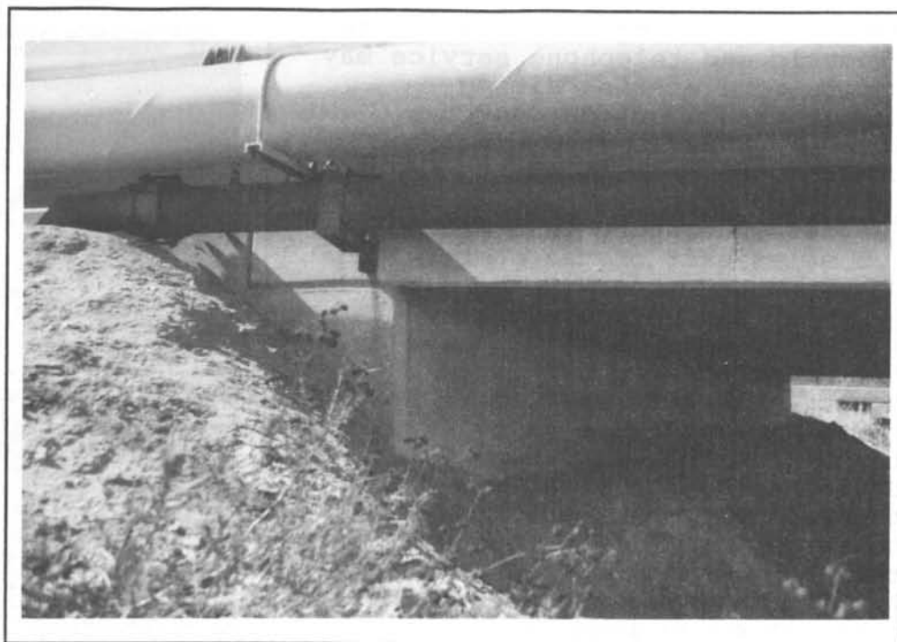
Figure 3.2-8 A Fiber Optic Conduit Hung From a Bridge With a Water Distribution Pipe Directly Above It
