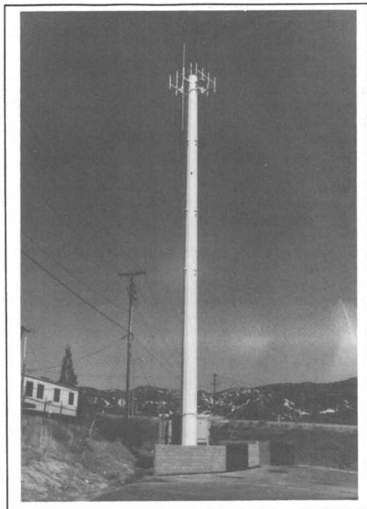
Figure 3.2-9 Cajon Junction Cellular Phone Antenna
