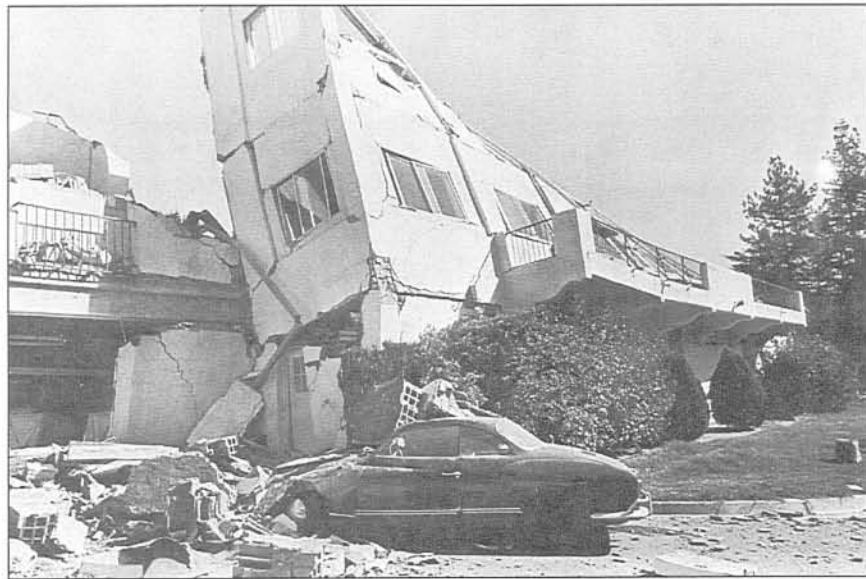
FIGURE A.3 Following the collapse of the Veteran's Administration hospital in the San Fernando earthquake of 1971, the VA has required seismic design for all its facilities. The hospital building shown in this photo was constructed in 1925 with concrete frames and concrete floors, and hollow-tile walls. This type of building is known to be hazardous in the event of a strong earthquake. (Source: Engineering Features of the San Fernando Earthquake , California Institute of Technology, EERL, 1971)
