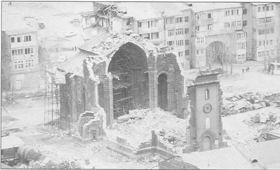
FIGURE 3.6 The extensive damage in Armenia in 1988 can be attributed to the lack of seismic-resistant design and construction. The same limitations are true of existing building stock throughout the United States. (Photo: NOAA)
