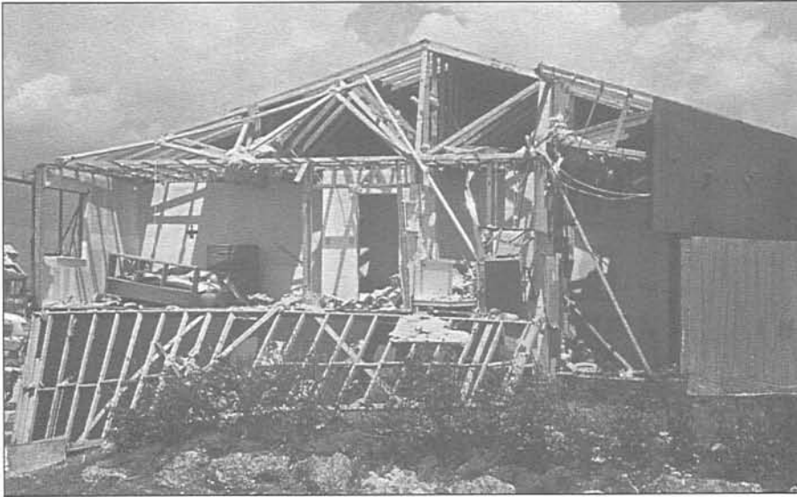
FIGURE 6.1 A substantial portion of the damage from Hurricane Andrew in 1992 was from lack of enforcement of the South Florida Building Code. 1 (Source: FEMA 1993)
