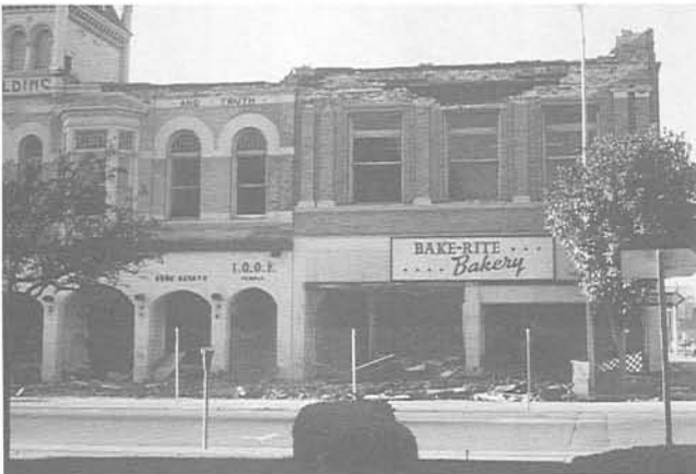
MMI VIII: Causes near panic; partial collapse of unreinforced masonry structures. (Photo: Rob Olshansky)
