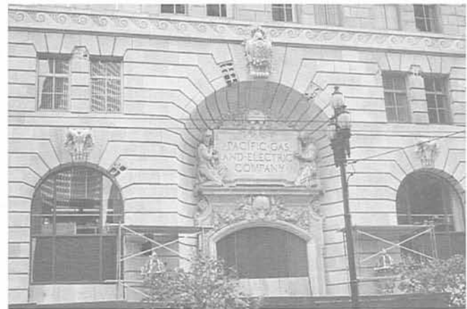
MMI VII: Disturbance frightens all; cracked chimneys; cracking in unreinforced masonry structures. (Photo: Rob Olshansky)
