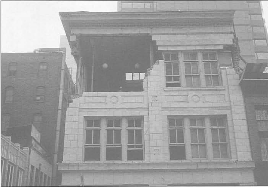
FIGURE 3.1 Most of the building damage in the 1989 Loma Prieta earthquake was to older unreinforced masonry buildings built before the adoption of seismic codes. (Photo: Rob Olshansky)
