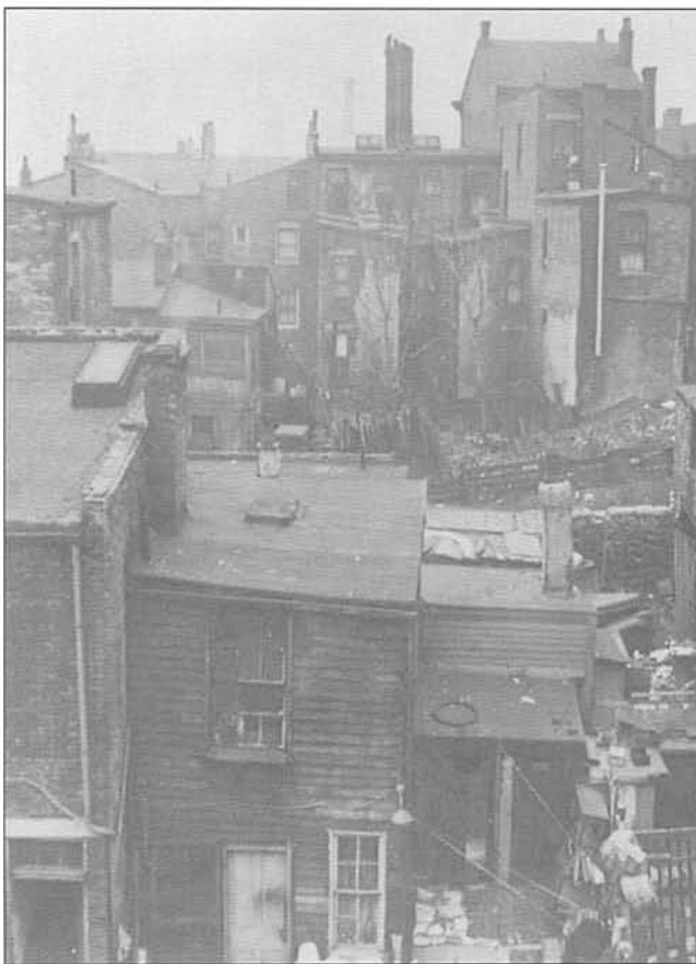
FIGURE 2.1 The first building codes were designed to improve substandard housing. (Photo: Presidents Commission on Urban Housing, 1968)
