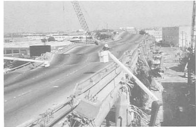
MMI IX: General panic; ground-cracking; considerable damage in buildings designed to seismic code. (Photo: J. David Rogers)
