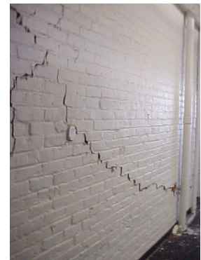
■ Figure 19. URM building damage, 2001 Nisqually, Washington earthquake.
