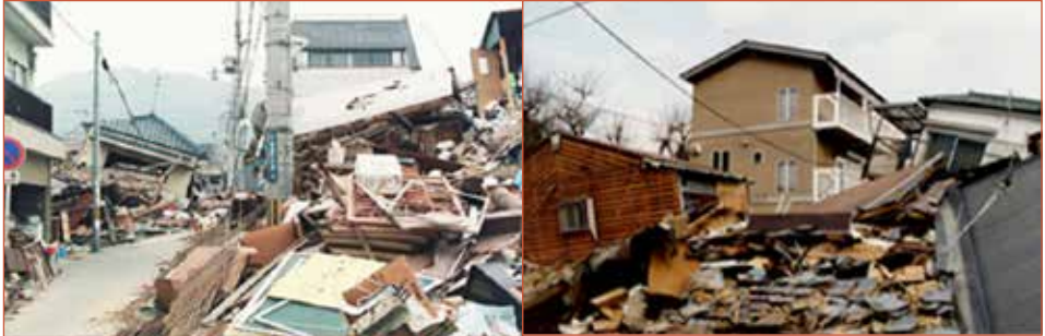
Figure 5.4.3 Many wooden houses collapsed in the Kobe Earthquake 1995 (left), but new houses, following the revised code in 1981, suffered little damage, even in otherwise heavily damaged areas (right)
