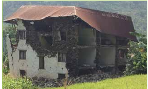
Figure 3.1.7. Delamination of masonry walls
