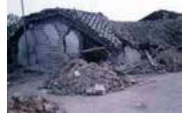
Adobe houses destroyed by EQ, 2001
