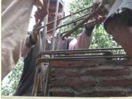
Figure 3.2.18. Connection of RC members Horizontal rebar for beams is not connected at the corner
