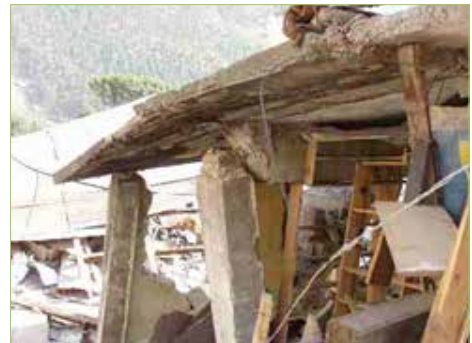
Figure 3.1.21. Connection failure
