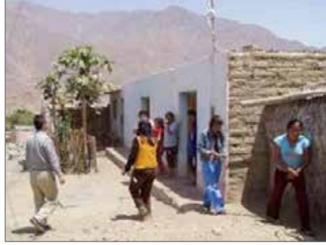
Figure A.2.8 House B: A house without reinforcement, next to House A
