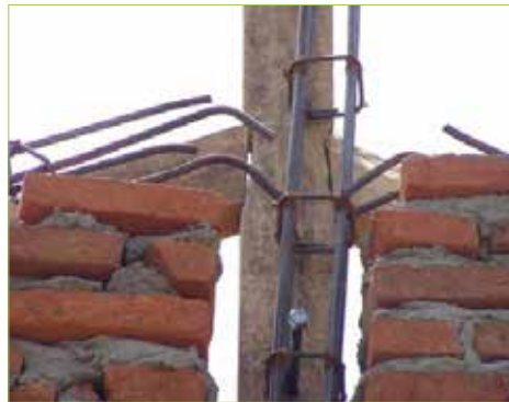
Figure 3.2.6. Construction practice on site Insufficient connection of longitudinal rebar
