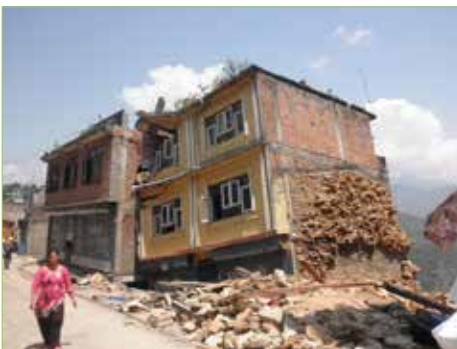
Figure 3.1.8. Damages to RC-framed brick building (Sindhupalchowk District)
