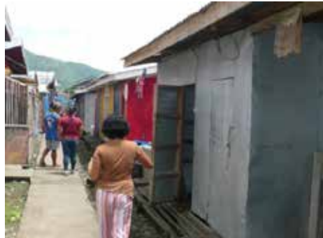
Bunk House in Tacloban City, Leyte, the Philippines (Photo: July 2015)
