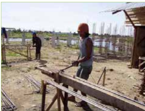
Figure 3.2.7 Bending works on site with simple tools Assembling of rebar is also conducted on ground
