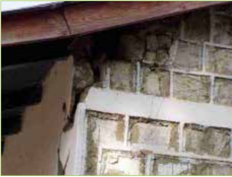
Figure 3.1.26. A school building made of dressed stone
