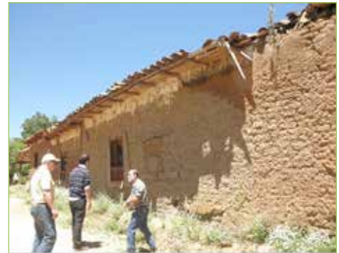
Figure 3.1.12. Adobe construction without appropriate maintenance work in Huerta del Maule in Maule Region
