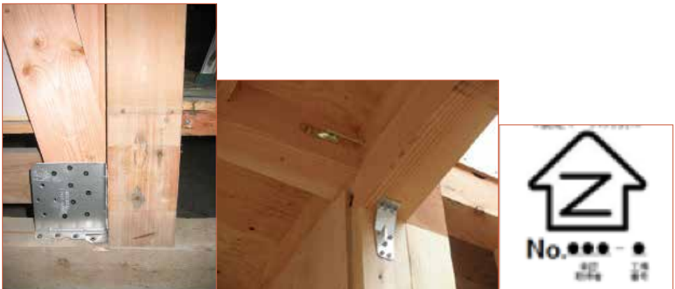
Figure 5.4.6 Example of metal connectors. Brace to plinth/column type (left), column to beam type (middle) Certificate mark of quality assurance scheme (right)
