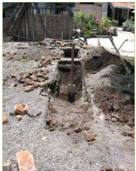
Figure 3.2.16. Excavation works for foundation
