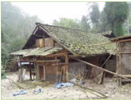
Figure 3.1.16. Timber house that did not collapse
