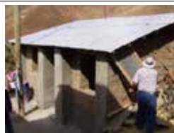
A seismic adobe house being constructed in the rural area development project by the NGOs
