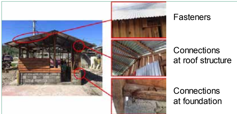
Figure 1. A non-engineered construction (left) and identified weak points by field survey (right).
