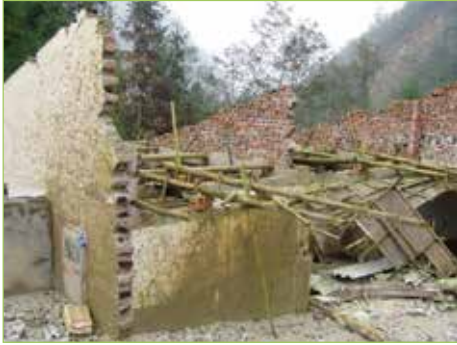
Figure 3.1.18. Damaged brick house
