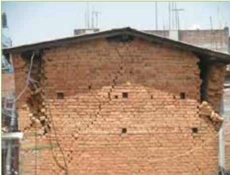
Figure 3.1.8. Damages to RC-framed brick building (Sindhupalchowk District)
