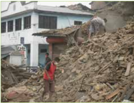
Figure 3.1.1. Completed destroyed structure (Gorkha earthquake in 2015)
