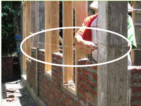
Figure 3.2.20. Laying work of bricks with taut line
