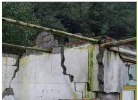
Figure 3.1.17. Damaged concrete block house
