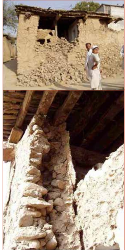
Figure 5.2.3 Typical damage to houses of undressed stone masonry with mud mortar, as shown in the Guideline (2005 Northern Pakistan Earthquake (Kashmir Earthquake)) Much typical damage to various types of structures are addressed
