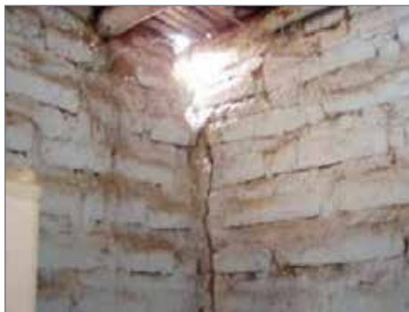
Figure A.2.10 maged Heavy cracks in House B
