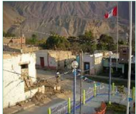
Figure A.2.6 Collapsed houses in central area of Zuniga, Lima state
