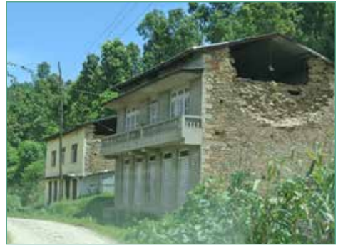
Figure 3.1.5. Out-of-plane failure in masonry walls
