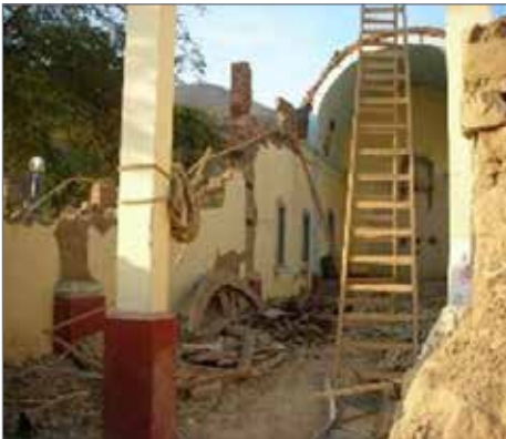
Figure A.2.5 Heavily damaged church (Adobe wall, vaulted roof made from quincha), Zuniga, Lima state
