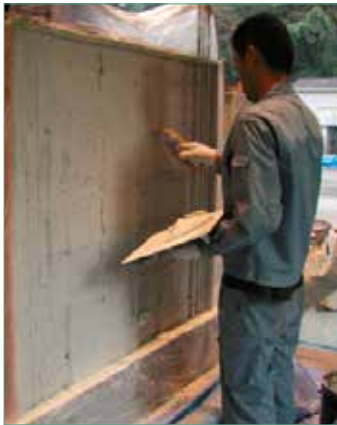
Figure 1. Construction of reinforced PCM wall
