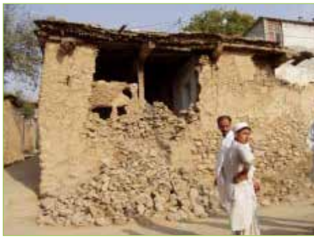
Figure 3.1.25. A house made of natural stone with mud mortar
