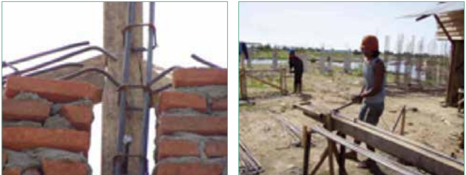
Figure 1.1.5 Inadequate detailing of rebar connections (left), and bending of rebar on site with simple tools (right), in Banda Aceh, Indonesia
