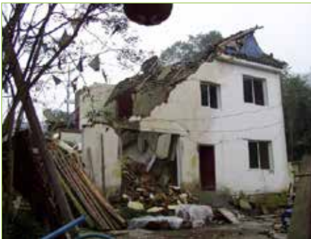
Figure 3.1.14. Damaged house with hollow core slabs PCa
